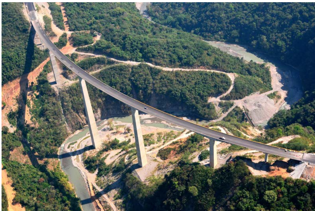
Figure 32. Overview of the finished bridge.
