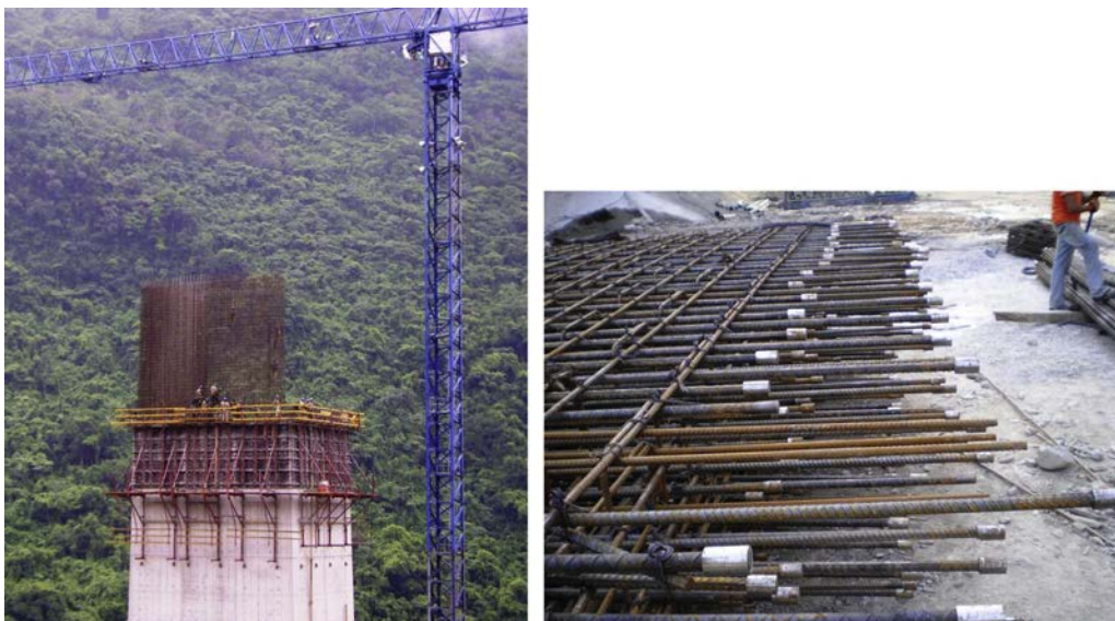
Figure 24. Pre-assembly of pier reinforcement.
