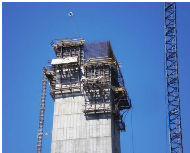
Figure 25. Conventional climbing formwork on piers 2, 3 and 5.
