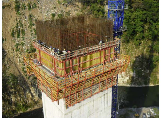
Figure 26. Self-climbing formwork on pier 4.
