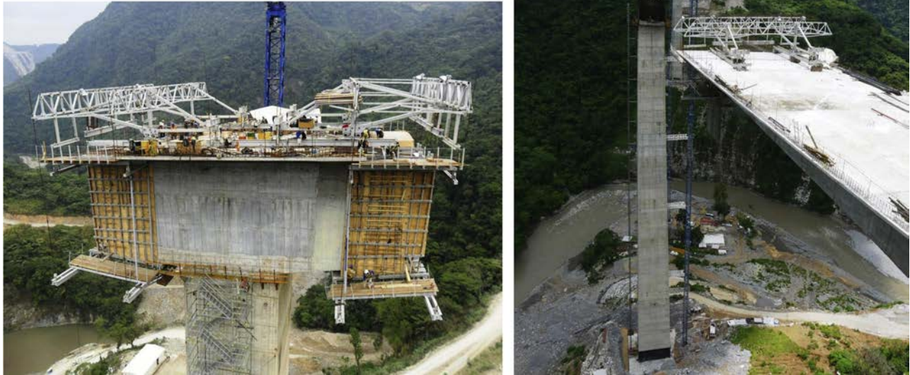
Figure 28. Overview of travelling formwork.
