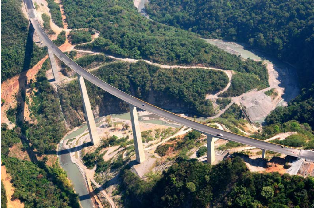
Figure 32. Overview of the finished bridge.
