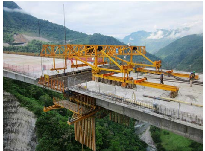
Figure 30. Locking a centre span.
