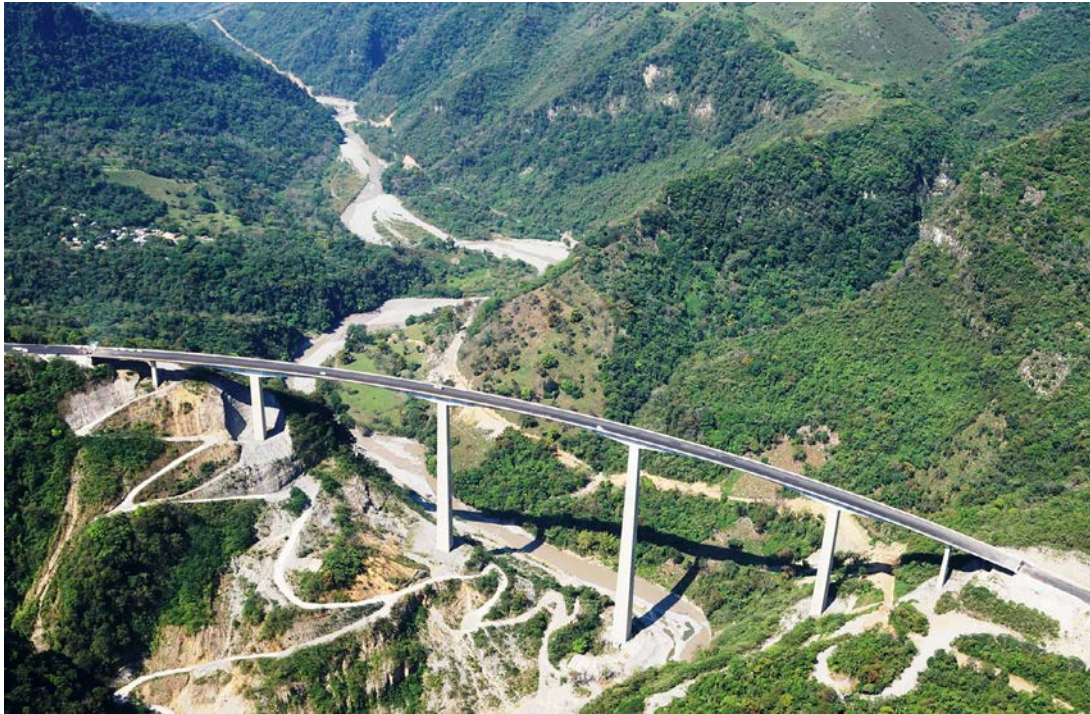
Figure 2. Overview of bridge.
