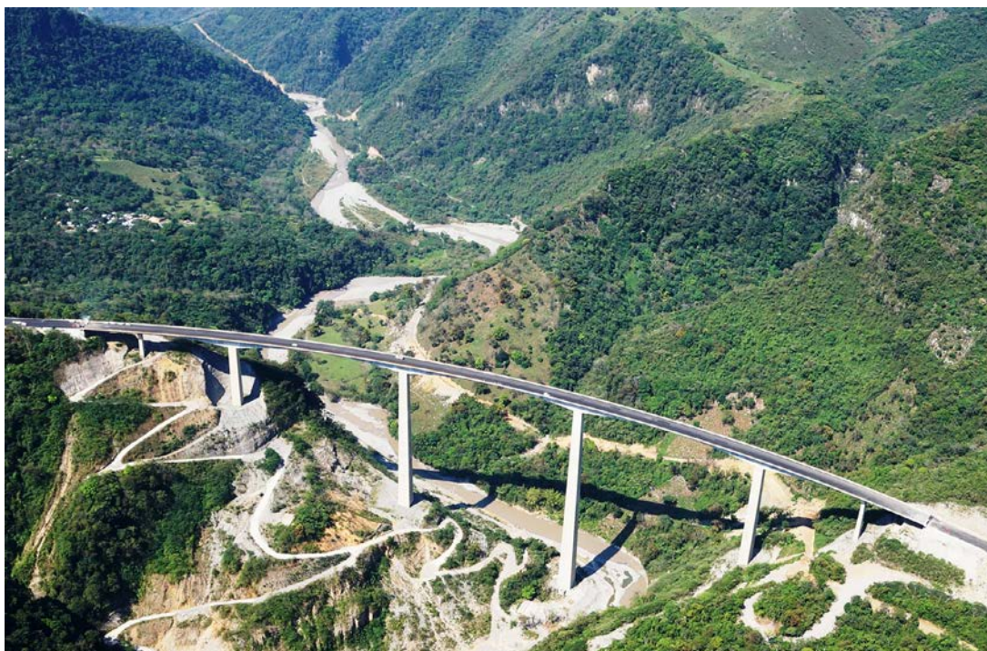
Figure 2. Overview of bridge.
