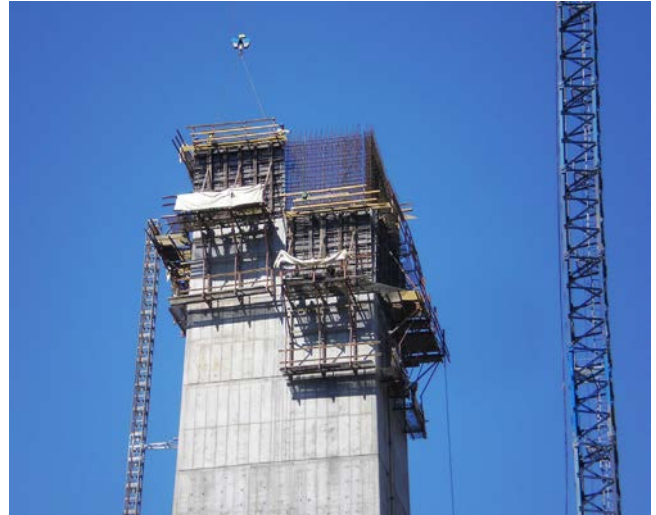
Figure 25. Conventional climbing formwork on piers 2, 3 and 5.
