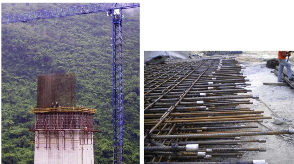
Figure 24. Pre-assembly of pier reinforcement.
