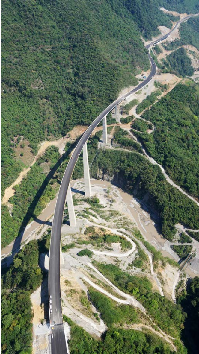
Figure 3. Overview of bridge.
