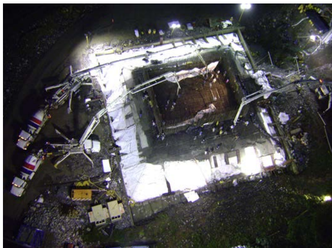
Figure 23. Continuous casting of pier 4 pile cap.
