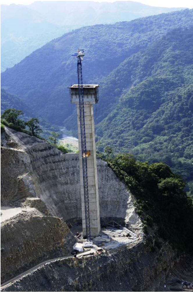
Figure 21. Pier 2 excavation.
