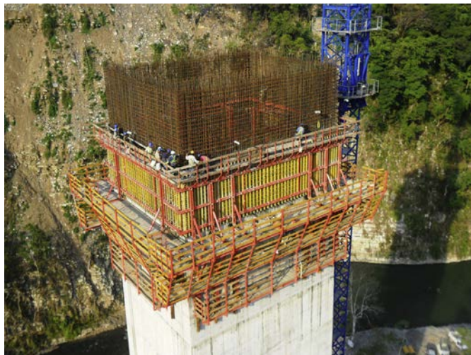
Figure 26. Self-climbing formwork on pier 4.
