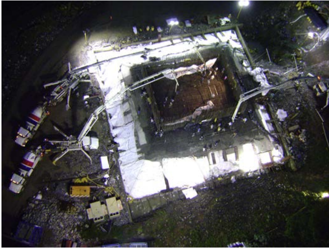
Figure 23. Continuous casting of pier 4 pile cap.
