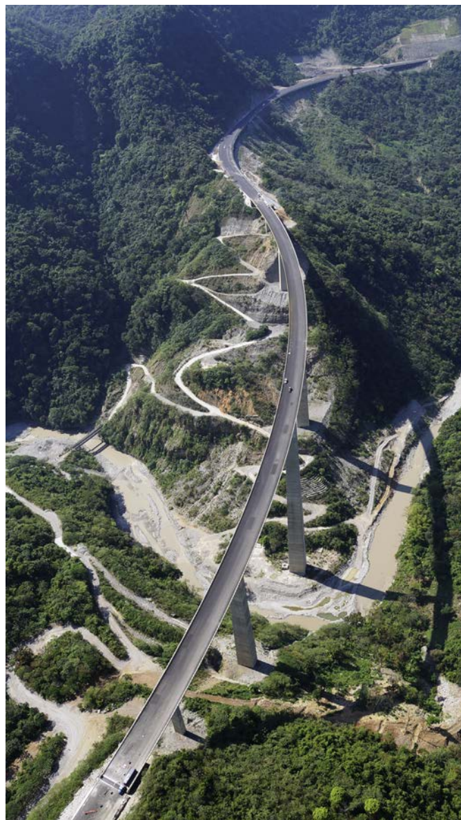
Figure 19. Overview of access road to the river from the Mexico City side of the valley.
