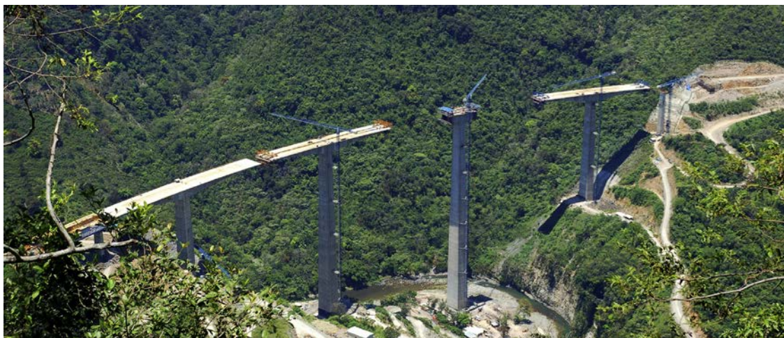
Figure 29. Simultaneous operation of three pairs of travellers.
