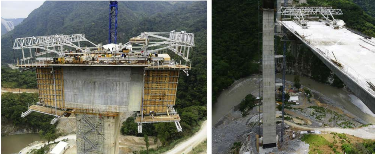
Figure 28. Overview of travelling formwork.
