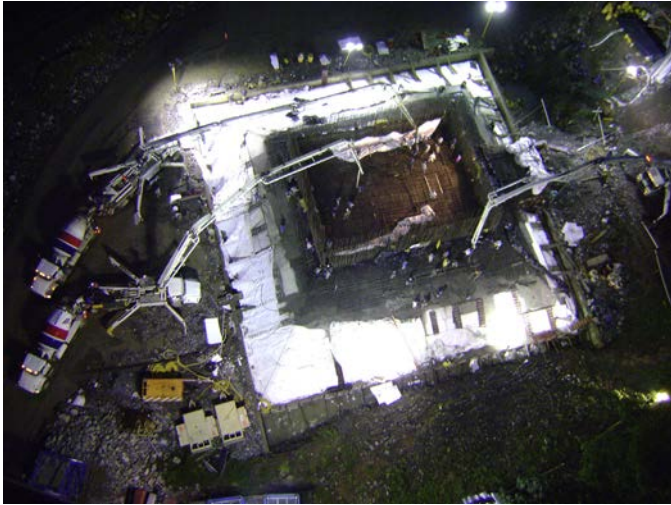
Figure 23. Continuous casting of pier 4 pile cap.
