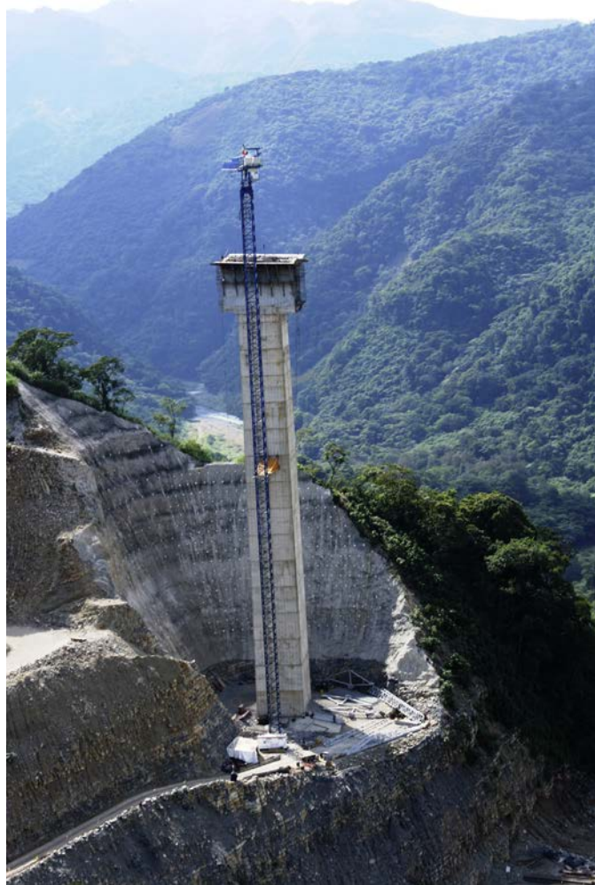
Figure 21. Pier 2 excavation.
