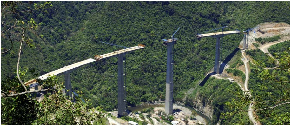
Figure 29. Simultaneous operation of three pairs of travellers.
