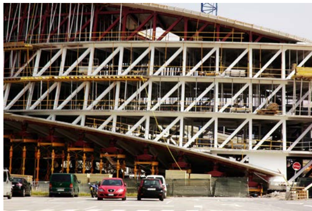
Figure 8. Side view of the outer truss during construction of the structural roof slab: note that the diagonals remain straight at the junction with bottom and roof slabs.
