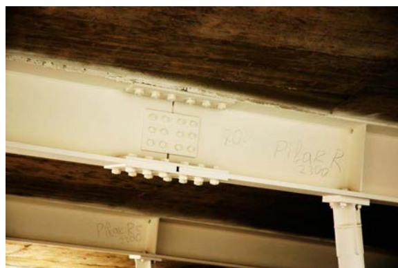
Figure 22. Bolted beam and beam-column joints.
