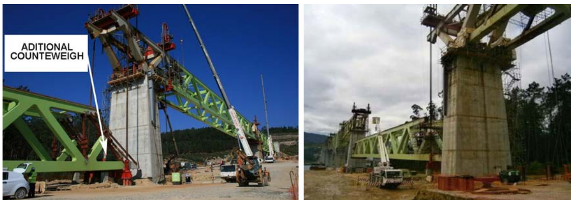
Figure 28. Hoisting sequence for spans 11 (left) and 10 (right).
