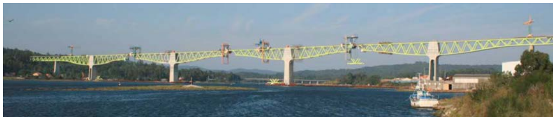
Figure 42. Hoisting the joining segment for span 6.
