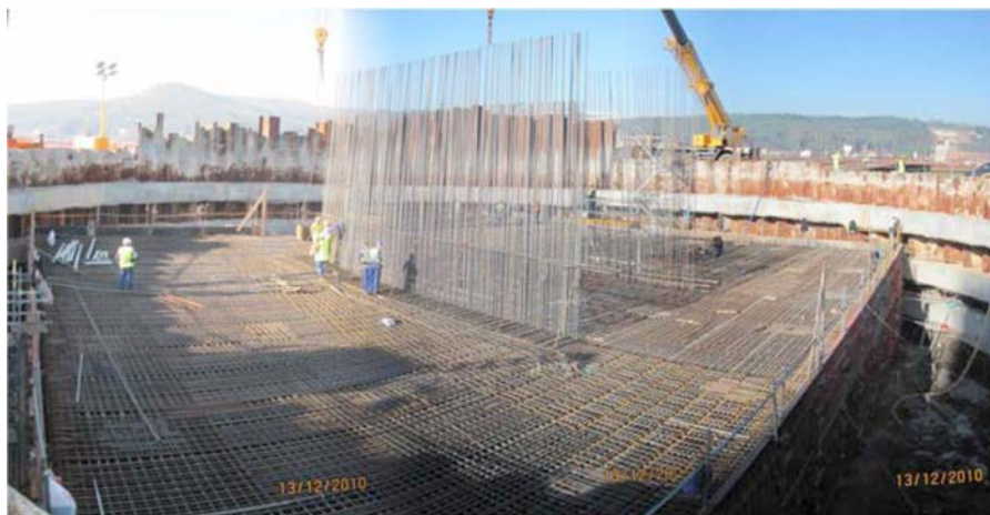
Figure 10. Reinforcement for P5 pile cap (30 m × 24.5 m × 4.5 m).
