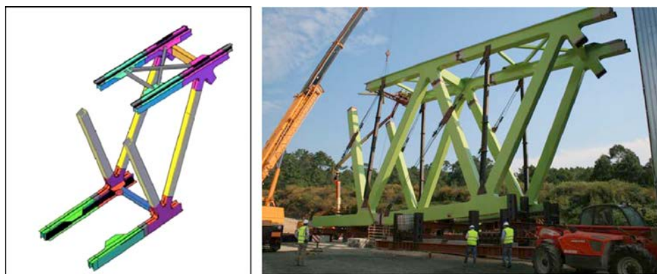
Figure 33. Segment breakdown into components and two segments assembled on the ground.
