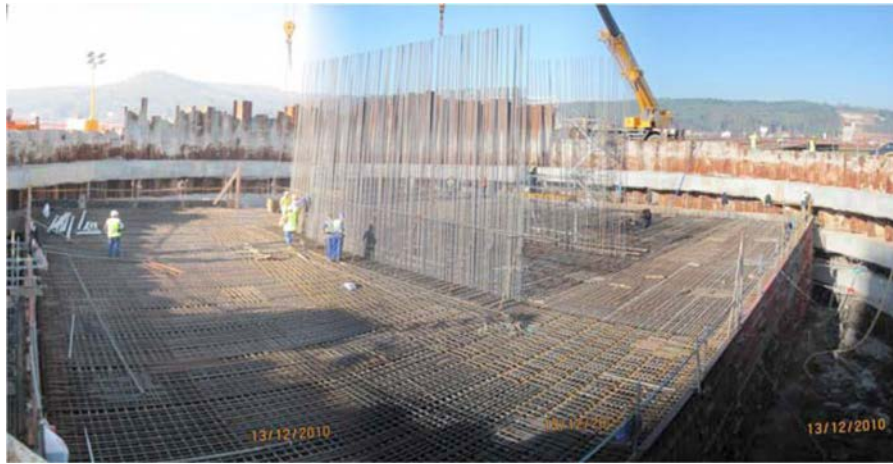
Figure 10. Reinforcement for P5 pile cap (30 m x 24.5 m x 4.5 m).
