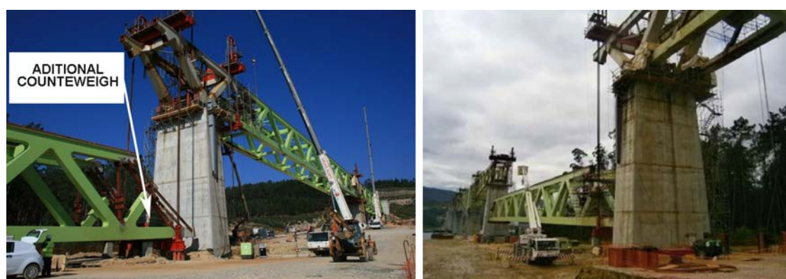
Figure 28. Hoisting sequence for spans 11 (left) and 10 (right).
