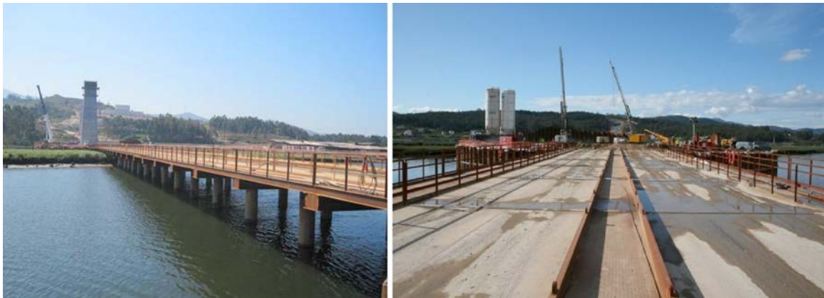
Figure 6. Wharf for accessing pier P5, P6 and P7 foundations.
