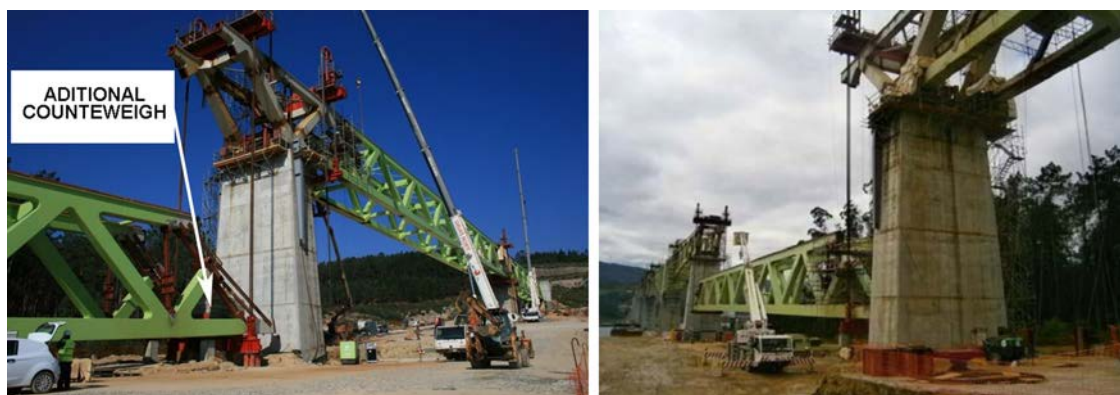
Figure 28. Hoisting sequence for spans 11 (left) and 10 (right).
