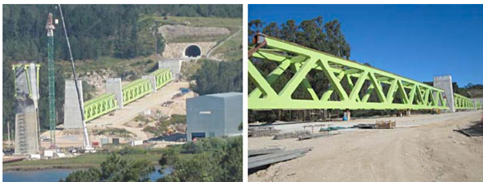
Figure 26. Sections for spans 10–12 built on the ground, ready for hoisting.
