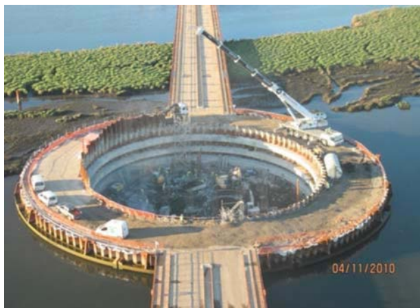
Figure 8. Inner excavation in P5 enclosure.
