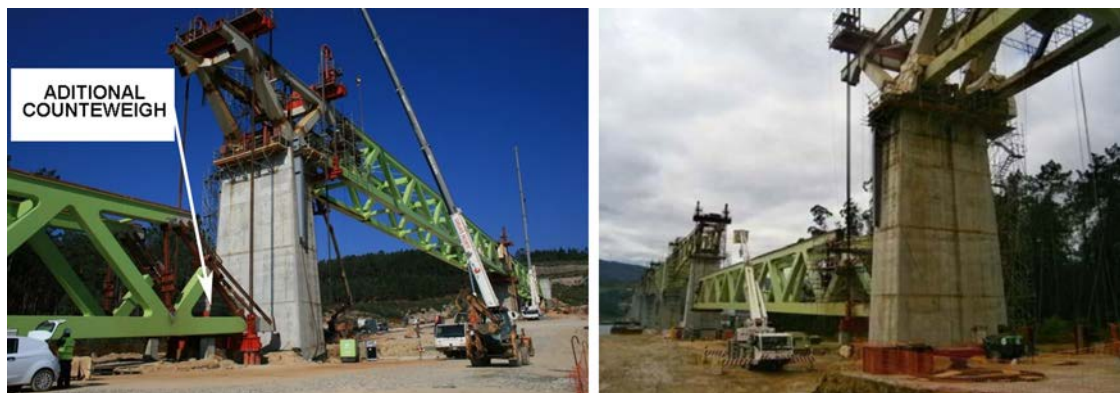
Figure 28. Hoisting sequence for spans 11 (left) and 10 (right).
