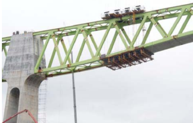
Figure 45. Travelling formwork for casting bottom slab concrete.
