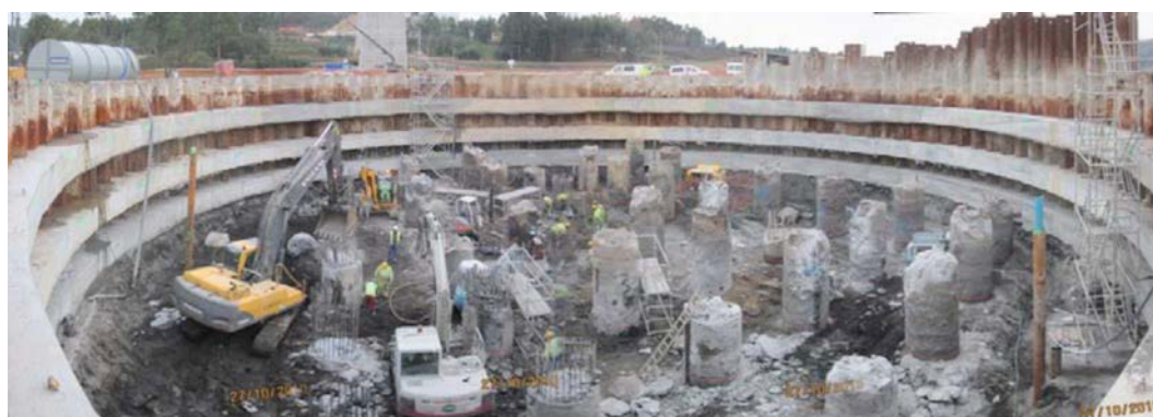
Figure 9. Cutting down P5 foundation pile heads.
