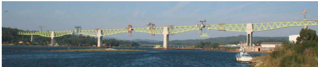
Figure 42. Hoisting the joining segment for span 6.
