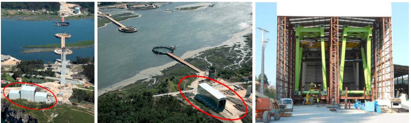
Figure 14. On-site segment assembly bays.
