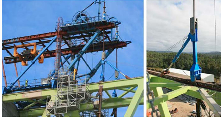
Figure 35. Hoisting a segment with a stationary derrick crane and detail of transverse hoisting beam.
