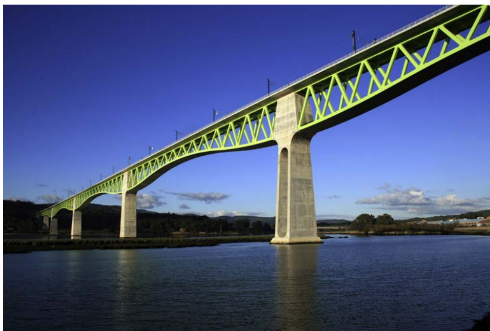
Figure 2. Variable depth centre spans. Pier 5 in the foreground.
