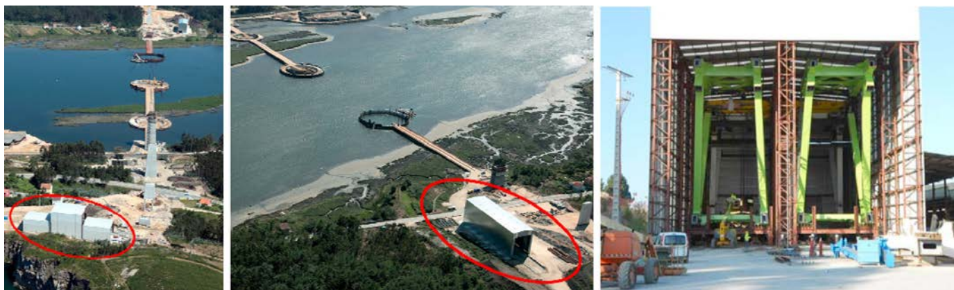
Figure 14. On-site segment assembly bays.
