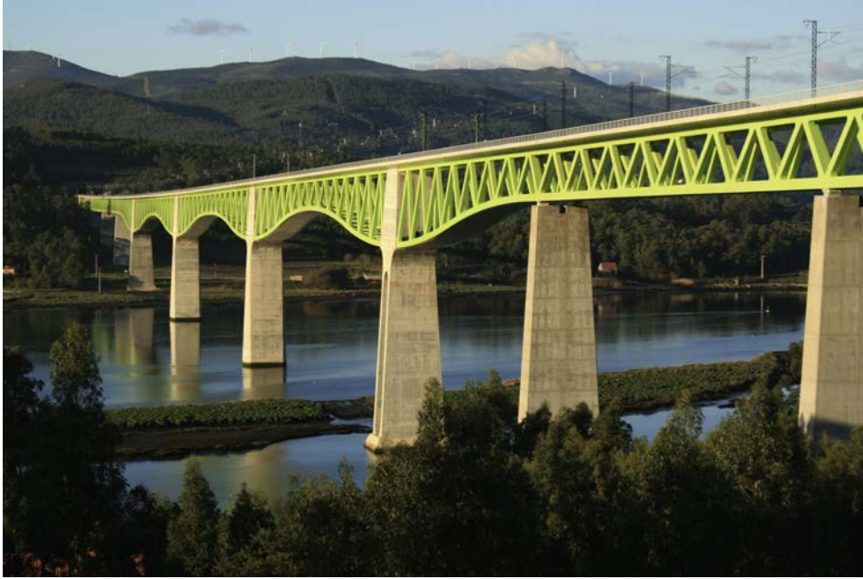
Figure 48. Finished viaduct, side view.
