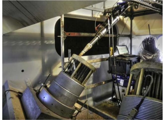
Figura 3. Isotension® Freyssinet.
