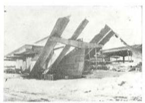
Fig. 6.—Anchorage: Derrumbamiento del Alaska Sales and Service.
