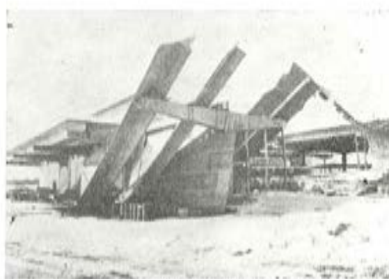
Fig. 6.—Anchorage: Derrumbamiento del Alaska Sales and Service.
