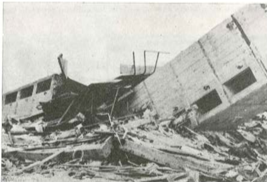
Fig. 8.—Anchorage (Four Seasons Building): Vista del inmueble hundido.
