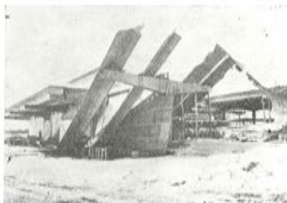
Fig. 6.—Anchorage: Derrumbamiento del Alaska Sales and Service.
