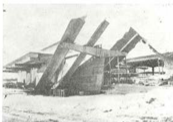
Fig. 6.—Anchorage: Derrumbamiento del Alaska Sales and Service.
