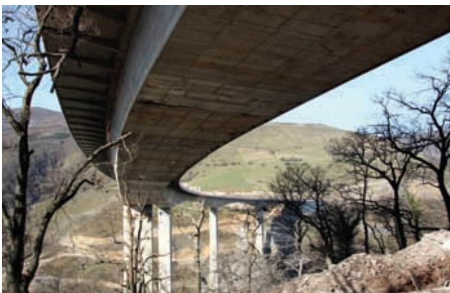
Figura 14. Vista inferior del tablero desde el estribo 2. Figure 14. Underneath view of the deck from abutment 2.
