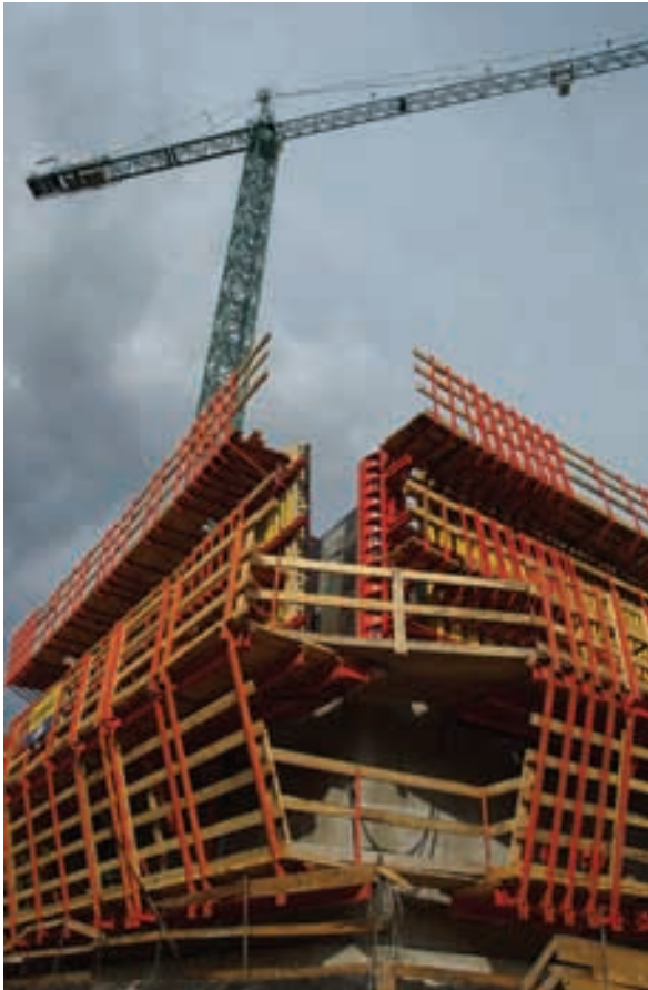
Figura 23. Detalle de autotrepa. Figure 23. Detail of the self-climbing formwork.
