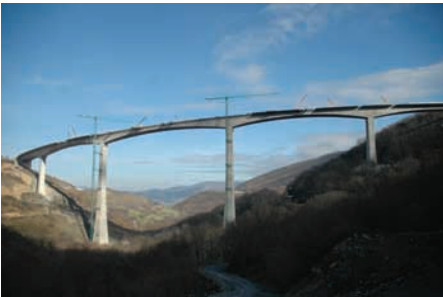
Figura 36. Vista general del viaducto. Figure 36. General view of the viaduct.
