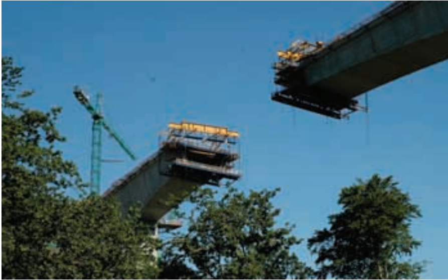
Figura 30. Detalle de carros acercándose en pilas 2 y 3. Figure 30. Detail of travellers approaching each other at piers 2 and 3.
