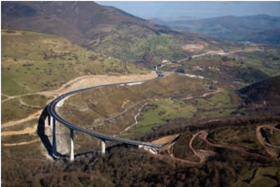
Figura 4. Vista general de la traza de la autovía. Figure 4. General view of the dual carriageway's alignment.
