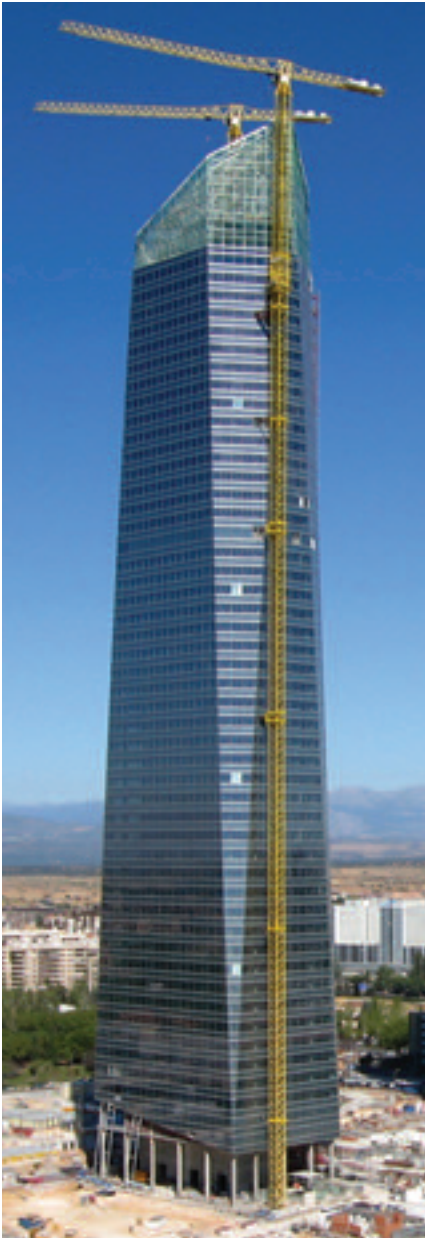
Figura 1. Torre. Vista general. Figure 1. Tower. Overview.
