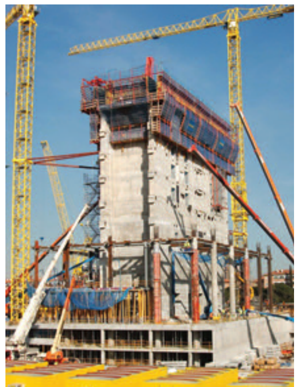
Figura 29. Vista general del arranque de la torre. Figure 29. Lower tower, at springing line.
