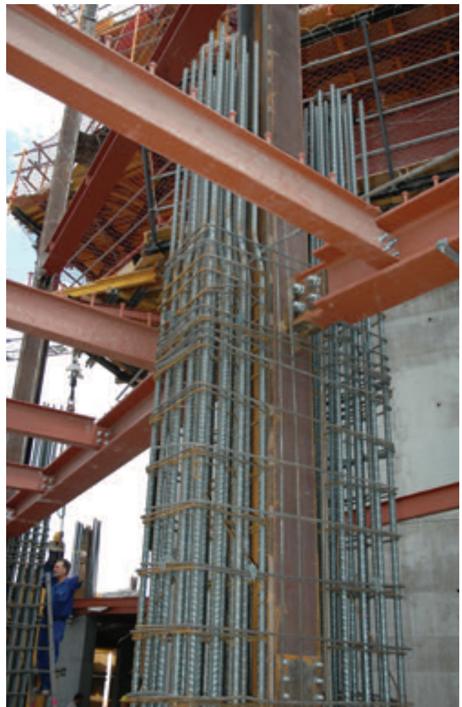
Figura 9. Soporte mixto densamente armado en la zona baja de la torre preparado para la colocación del encofrado. Figure 9. Joints between sections of steel supports, capable of withstanding the wind loads during construction.
