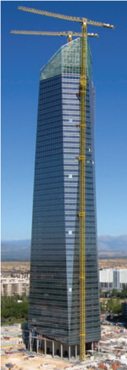
Figura 1. Torre. Vista general. Figure 1. Tower. Overview.
