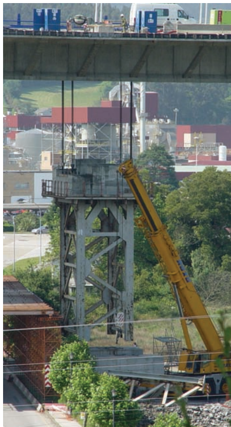
Figura 22. Retirada de pilas provisionales. Figure 22. Removal of provisional piers.
