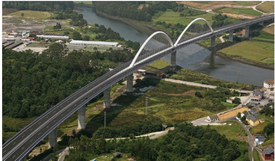
Figura 23. Vista aérea del viaducto acabado. Figure 23. Aerial view of the finished viaduct.
