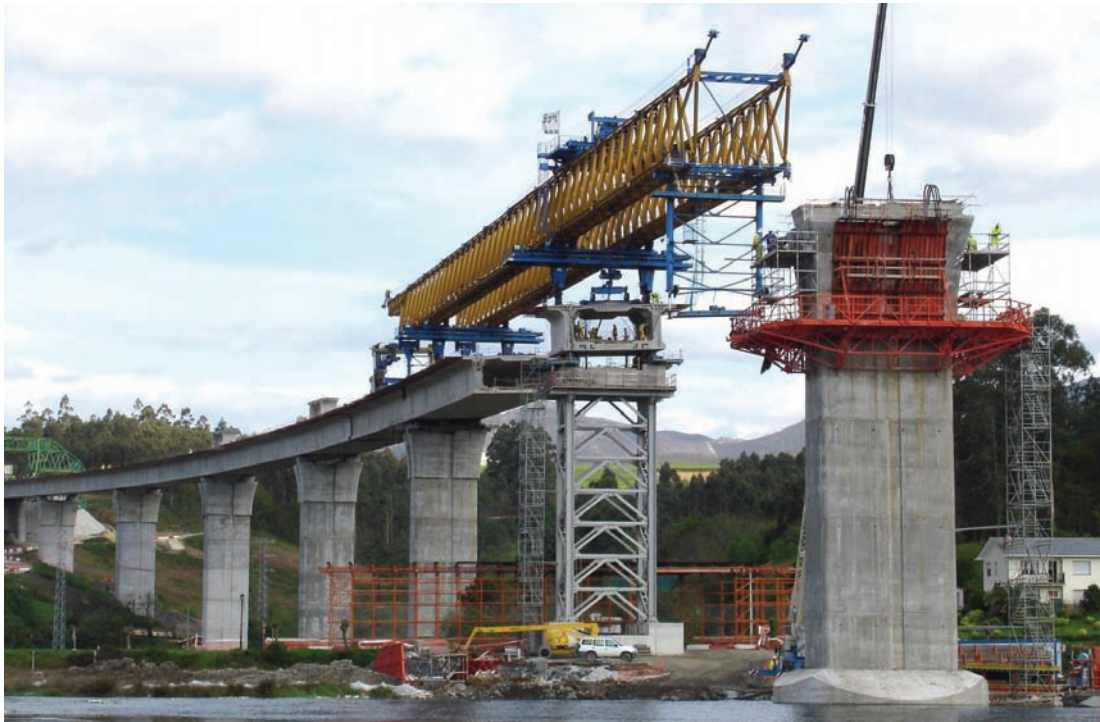
Figura 17. Montaje de dovelas. Figure 17. Segment assembly.
