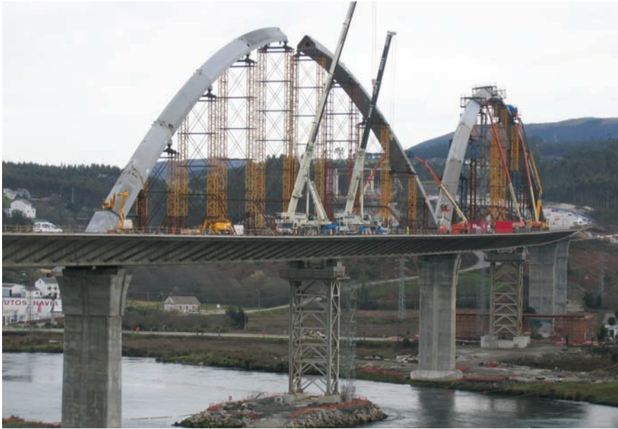
Figura 19. Montaje de arcos. Figure 19. Arch assembly.
