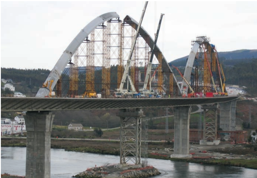
Figura 19. Montaje de arcos. Figure 19. Arch assembly.
