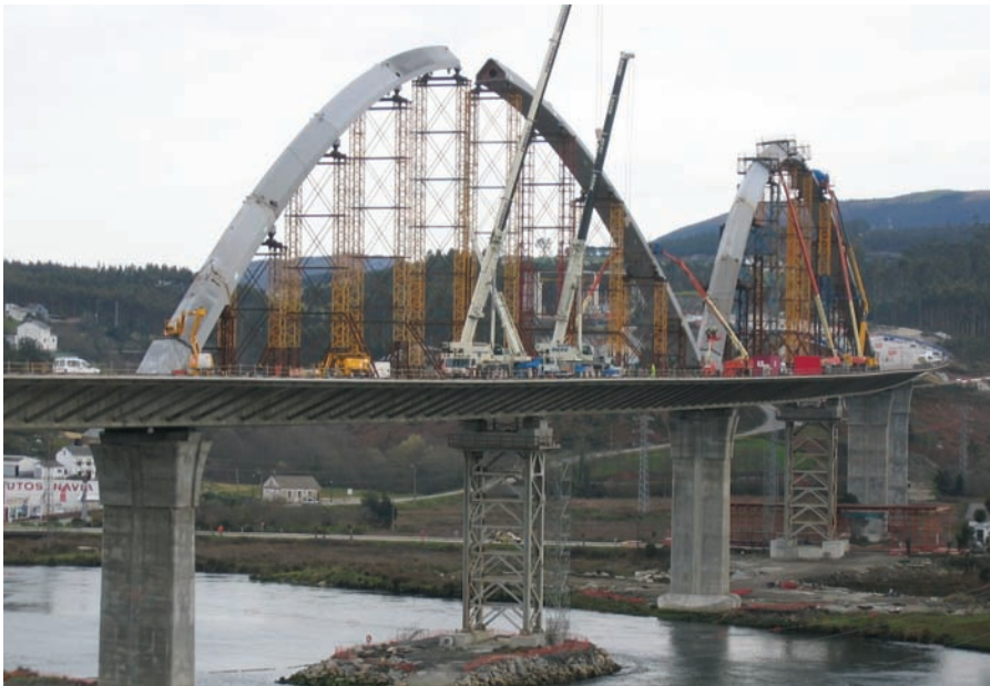
Figura 19. Montaje de arcos. Figure 19. Arch assembly.
