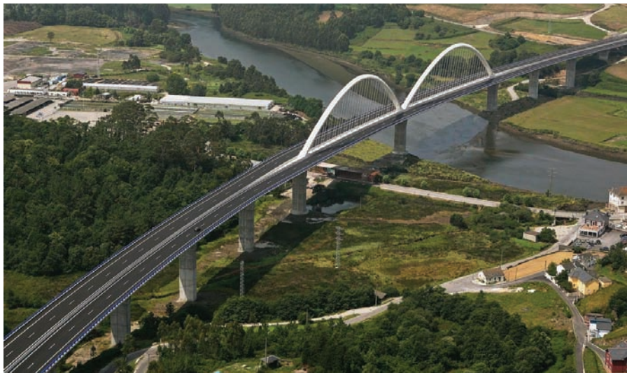
Figura 23. Vista aérea del viaducto acabado. Figure 23. Aerial view of the finished viaduct.
