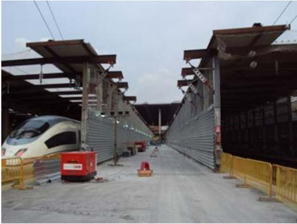
Figure 36. Provisional tunnels to protect tracks.
