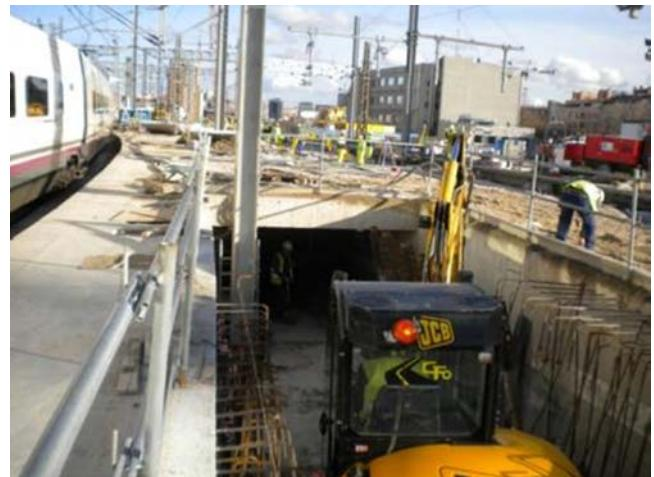
Figure 9. Catering ramps while under construction.
