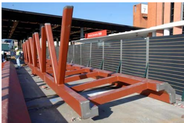
Figure 58. Roof module on the worksite.
