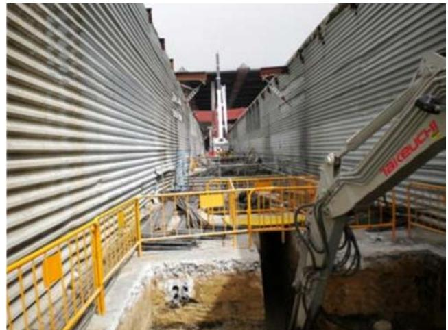
Figure 43. Micropile and pile cap construction between provisional track protection tunnels.
