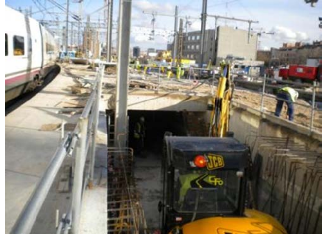
Figure 9. Catering ramps while under construction.
