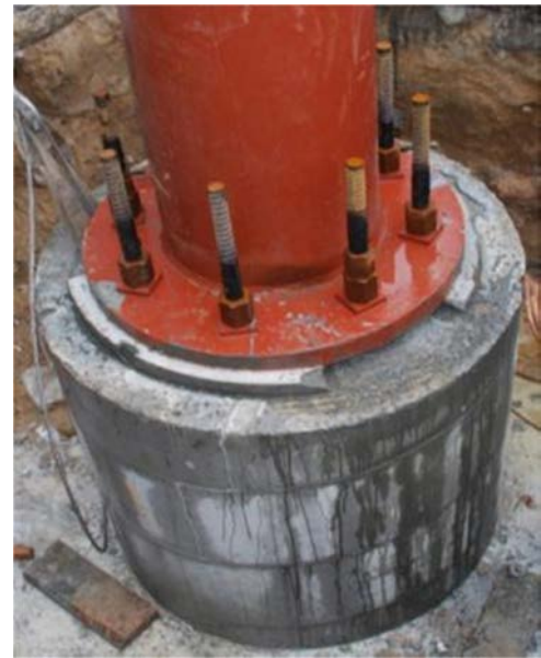
Figure 16. North side low-rise canopy foundations.
