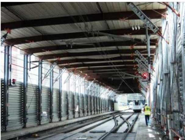
Figure 37. Inside view of provisional tunnels.
