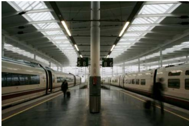
Figure 56. Finished low-rise canopies.
