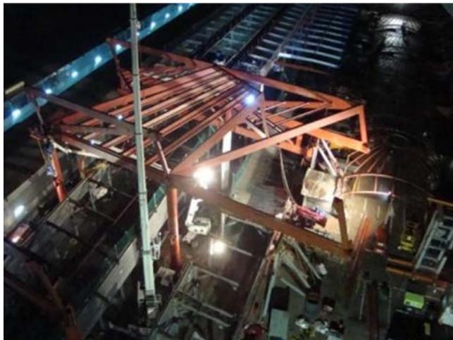
Figure 52. Assembly of the first high-rise canopy module.
