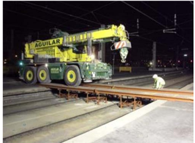
Figure 46. Inter-platform machinery traffic.
