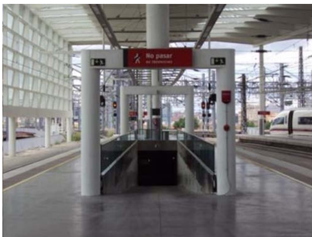
Figure 10. Finished catering ramps.
