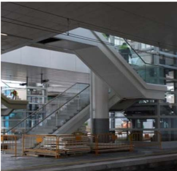
Figure 6. Stairway from platform to footbridge.
