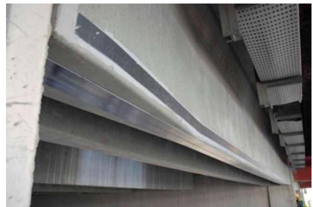
Figure 22. Carbon fibre flexural strengthening for secondary beams.
