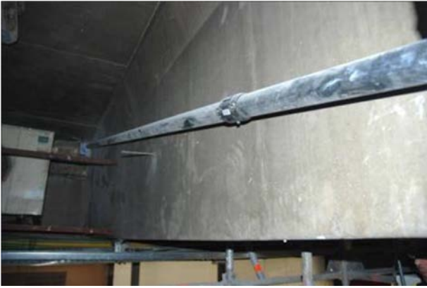
Figure 24. Existing beam strengthened with external post-tensioning.
