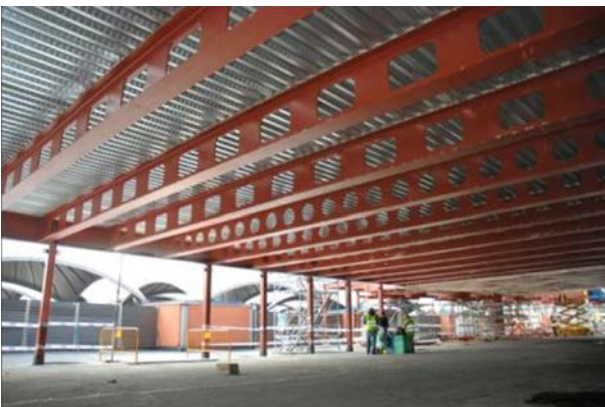
Figure 29. Composite beams with circular openings and “racecourses”.
