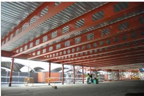
Figure 29. Composite beams with circular openings and “racecourses”.
