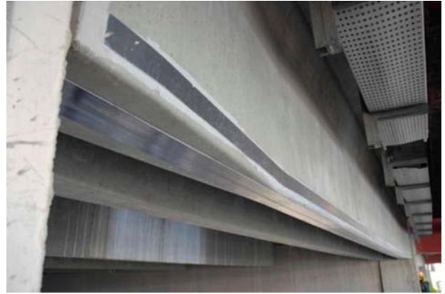
Figure 22. Carbon fibre flexural strengthening for secondary beams.
