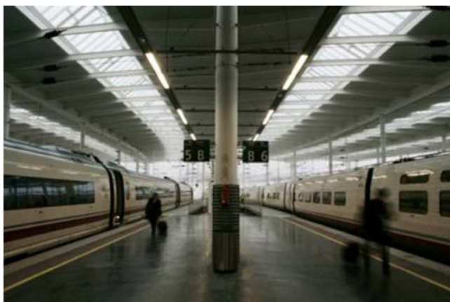
Figure 56. Finished low-rise canopies.
