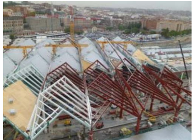
Figure 51. Bridge cranes over the high-rise canopies.
