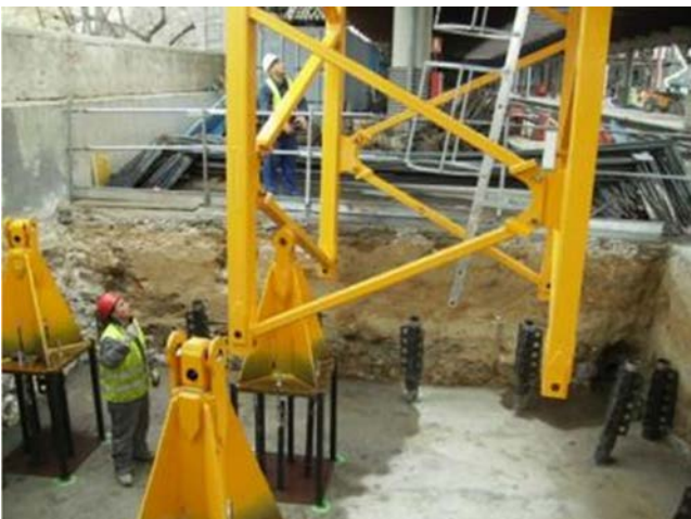
Figure 49. Erecting crane on platform 8.
