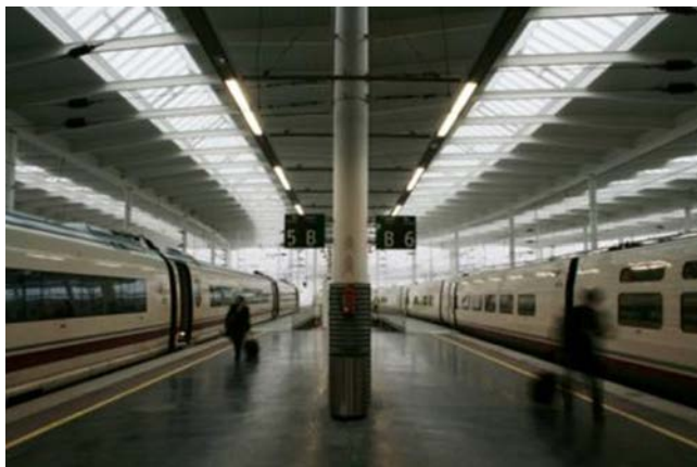
Figure 56. Finished low-rise canopies.
