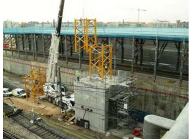
Figure 50. Portal frame for tower crane between local and high-speed lines.
