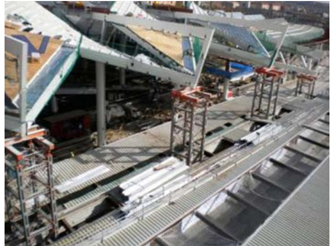
Figure 54. Shoring towers on platform 7.
