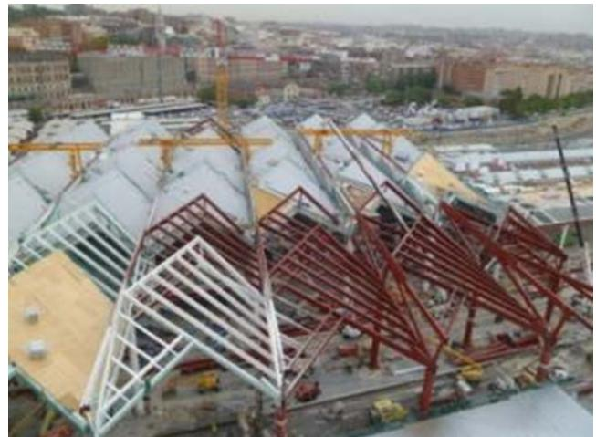
Figure 51. Bridge cranes over the high-rise canopies.
