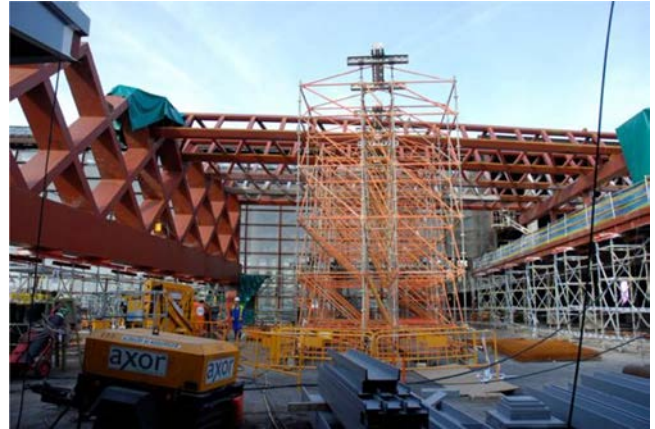
Figure 57. Modular roof construction.
