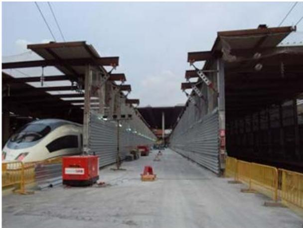
Figure 36. Provisional tunnels to protect tracks.
