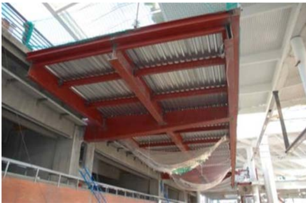
Figure 28. View of cantilevered by-pass from high-speed tracks.
