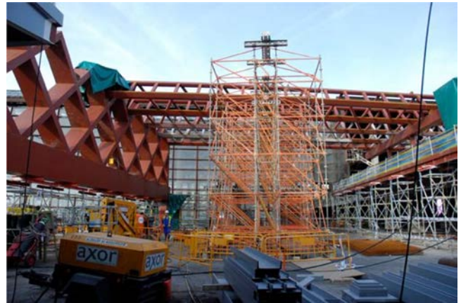
Figure 57. Modular roof construction.
