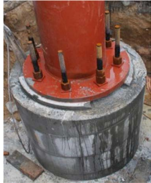
Figure 16. North side low-rise canopy foundations.
