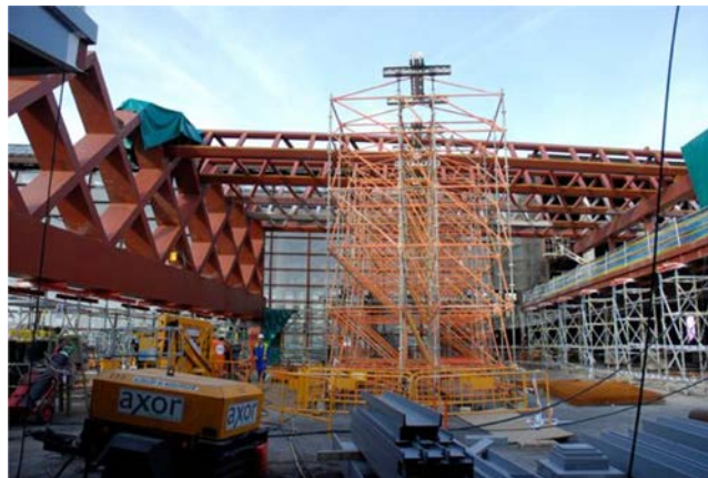
Figure 57. Modular roof construction.
