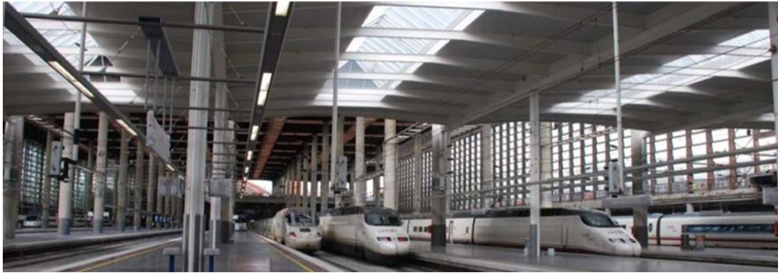
Figure 4. North side low-rise canopies.
