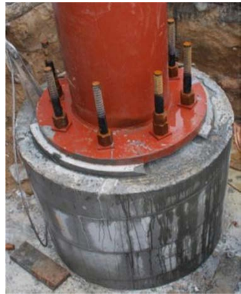
Figure 16. North side low-rise canopy foundations.
