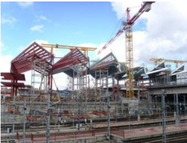
Figure 53. Shoring towers in the local train area.
