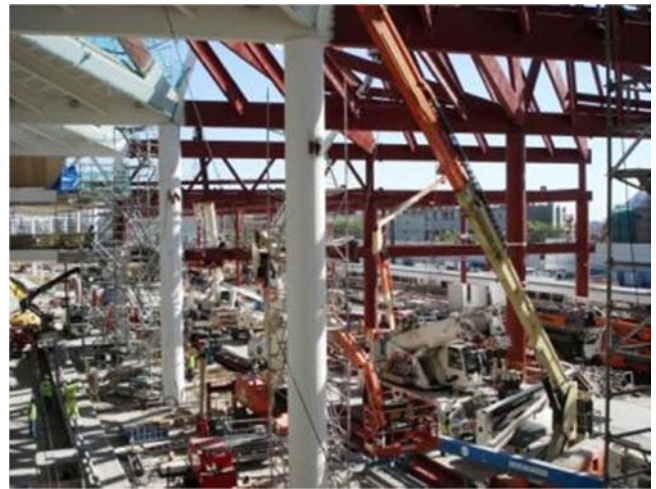
Figure 47. Coordination of machinery traffic.
