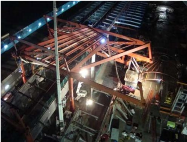
Figure 52. Assembly of the first high-rise canopy module.
