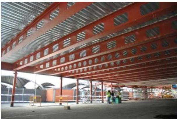
Figure 29. Composite beams with circular openings and "racecourses".
