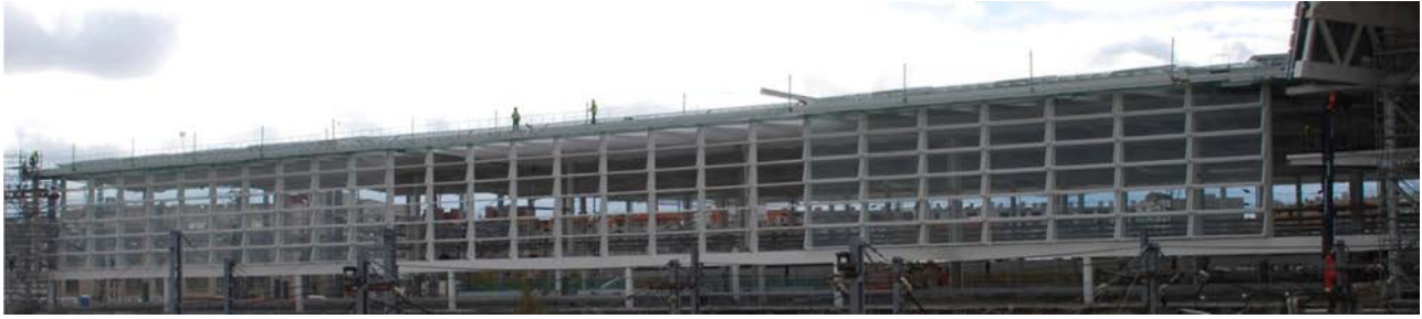
Figure 15. Curtain wall during construction.
