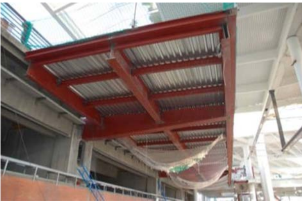
Figure 28. View of cantilevered by-pass from high-speed tracks.
