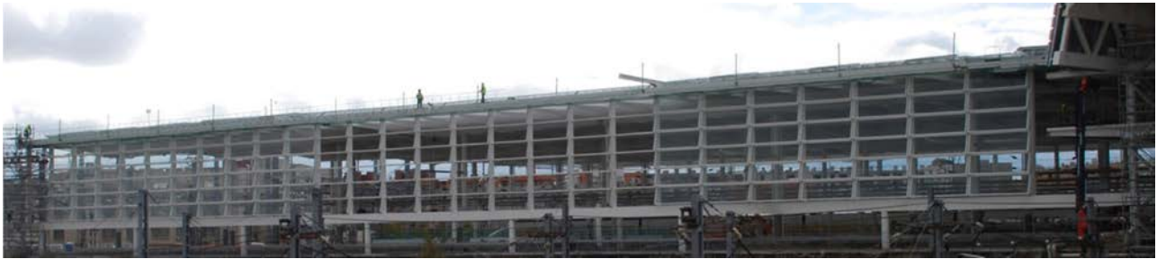
Figure 15. Curtain wall during construction.
