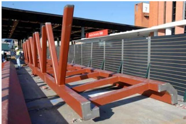
Figure 58. Roof module on the worksite.
