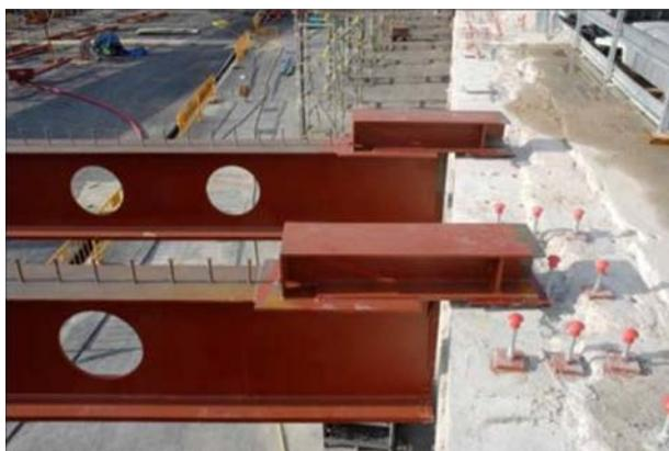
Figure 32. Rabbeted skid shoe (during construction).
