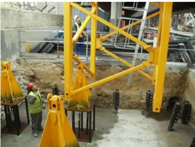
Figure 49. Erecting crane on platform 8.
