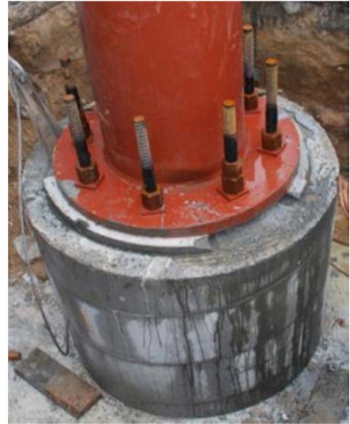
Figure 16. North side low-rise canopy foundations.
