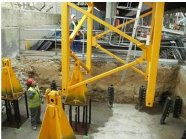
Figure 49. Erecting crane on platform 8.
