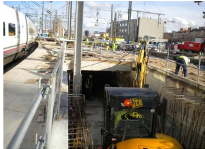
Figure 9. Catering ramps while under construction.
