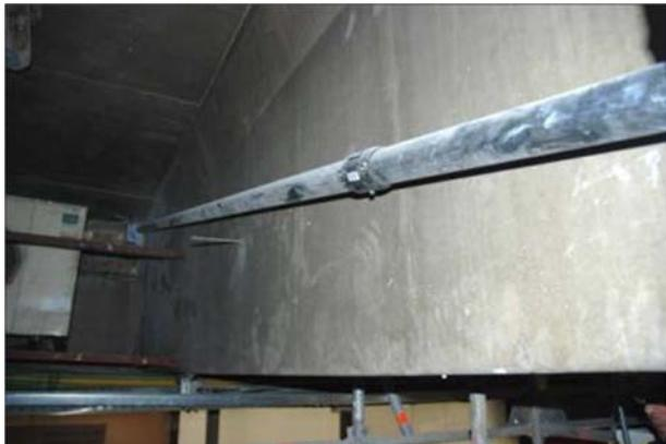
Figure 24. Existing beam strengthened with external post-tensioning.
