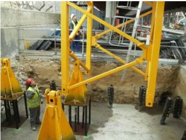
Figure 49. Erecting crane on platform 8.
