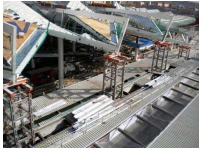
Figure 54. Shoring towers on platform 7.
