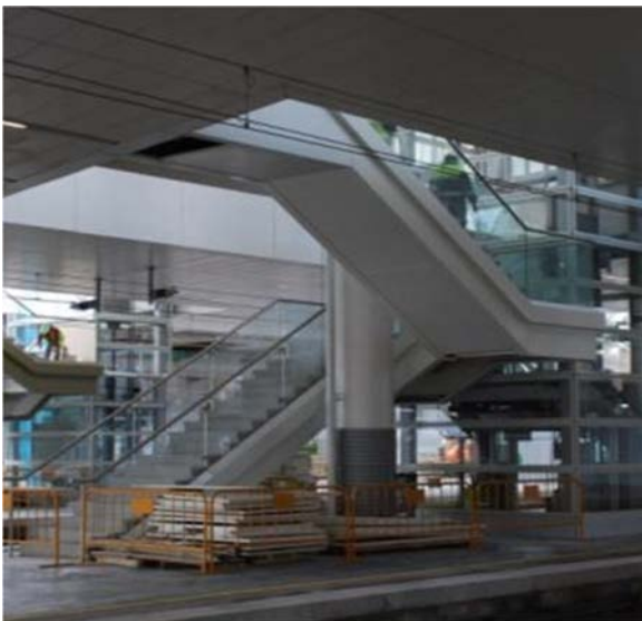
Figure 6. Stairway from platform to footbridge.
