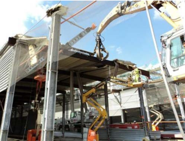
Figure 44. Demolition of provisional tunnels.
