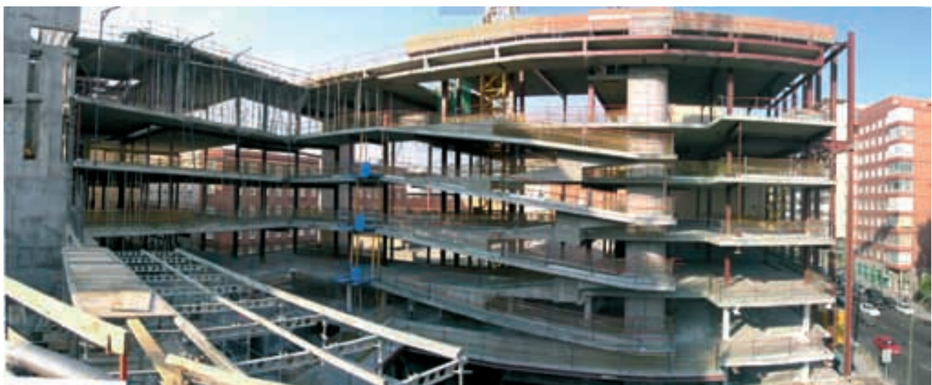
Figura 22. Vista general del Centro Coreográfico en fase de construcción Figure 22. General of the Choreographic Centre during construction.
