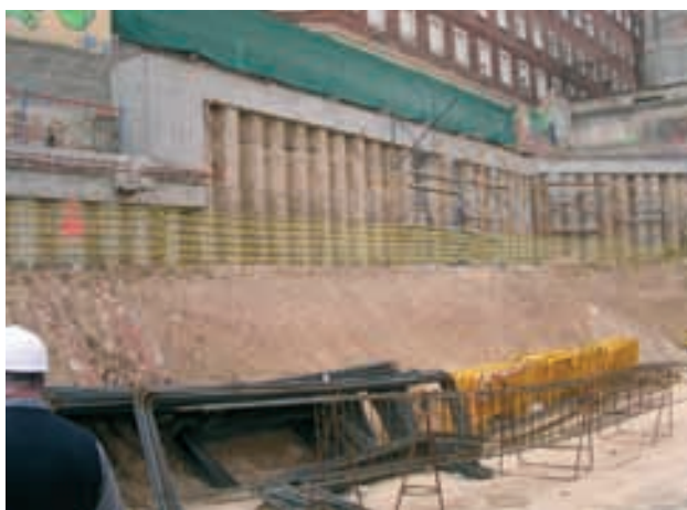
Figura 31. Contención perimetral del solar. Figure 31. Retaining wall.
