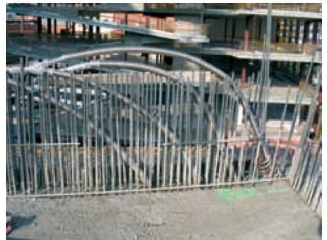
Figura 10. Pretensado de pantallas laterales del Teatro Principal Figure 10. Main Theatre lateral walls prestressing.
