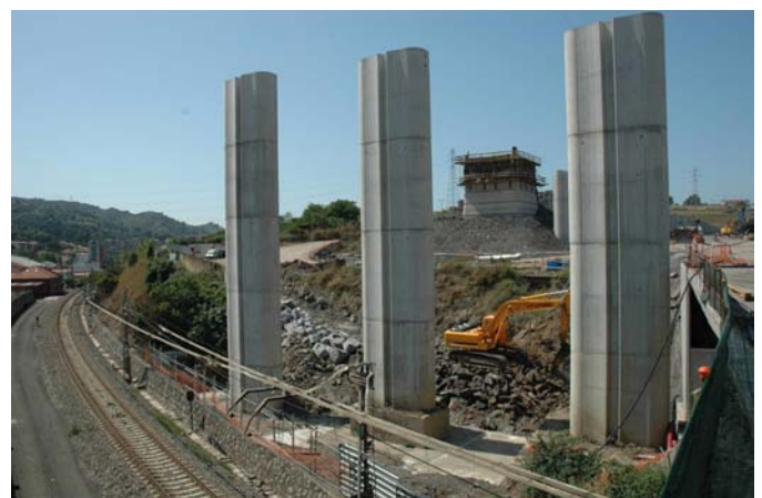
Figure 29. Piers in the transition area.
