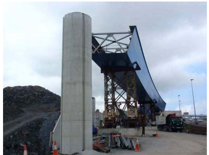
Figure 28. Piers of approach branches.
