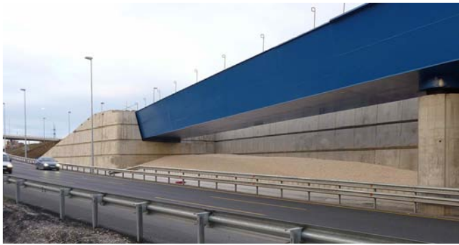
Figure 31. View of the abutments of the approach branches.
