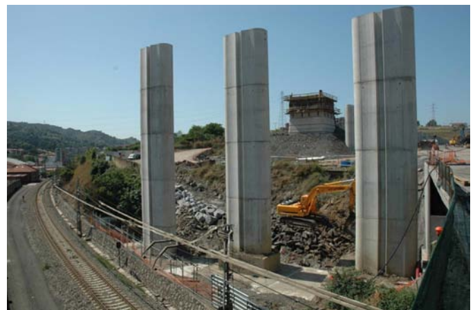
Figure 29. Piers in the transition area.
