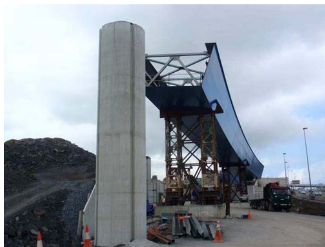
Figure 28. Piers of approach branches.
