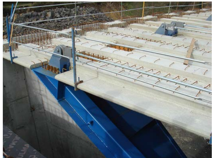
Figure 14. Main viaduct. Placed precast slabs.
