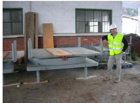
Figure 26. Image of the Pot type bearings.
