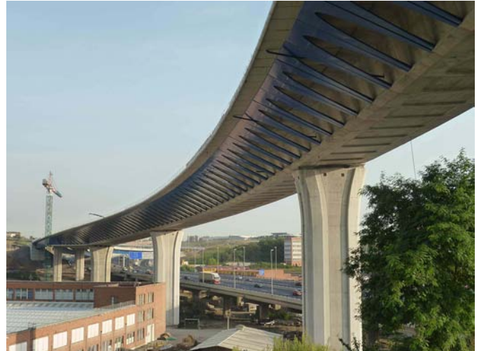
Figure 6. Overall view of the main viaduct.
