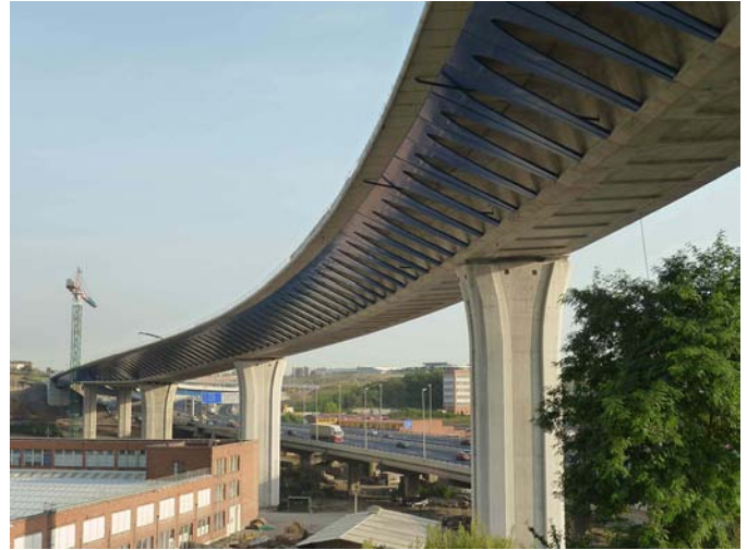
Figure 6. Overall view of the main viaduct.
