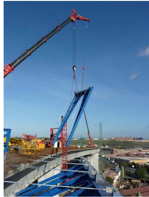
Figure 15. Main viaduct. Assembly of side brackets.
