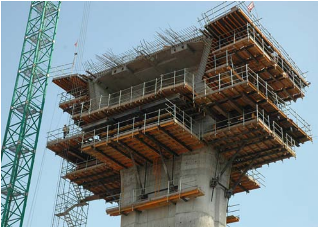
Figure 8. Work platforms of Segment Zero.
