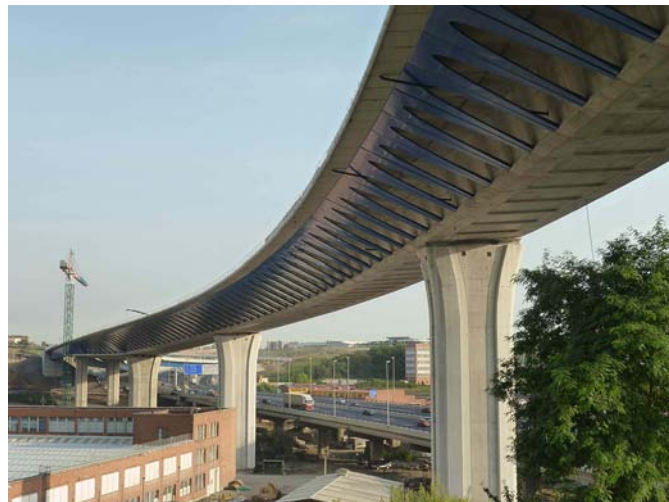
Figure 6. Overall view of the main viaduct.
