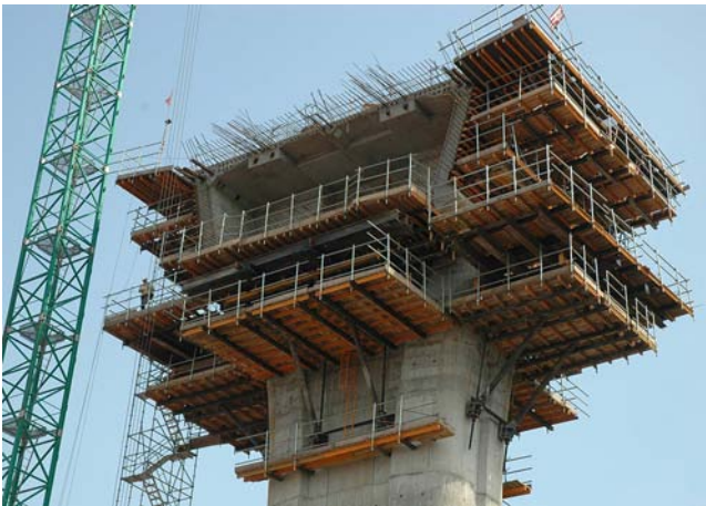
Figure 8. Work platforms of Segment Zero.
