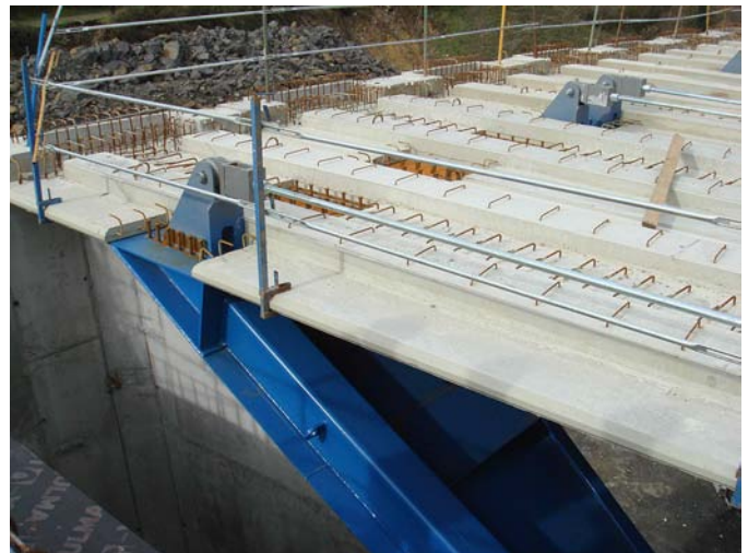
Figure 14. Main viaduct. Placed precast slabs.
