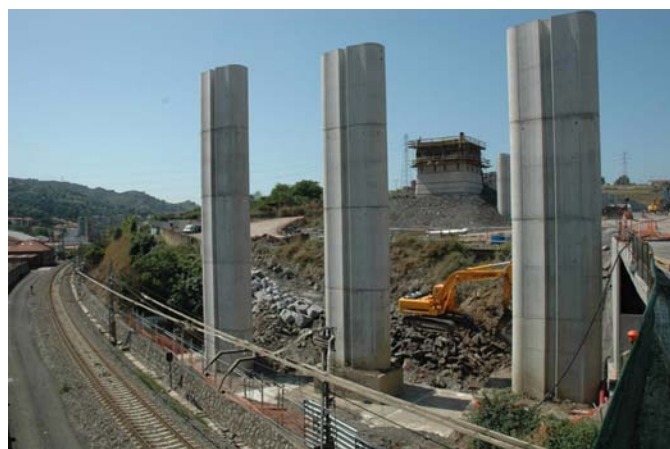
Figure 29. Piers in the transition area.
