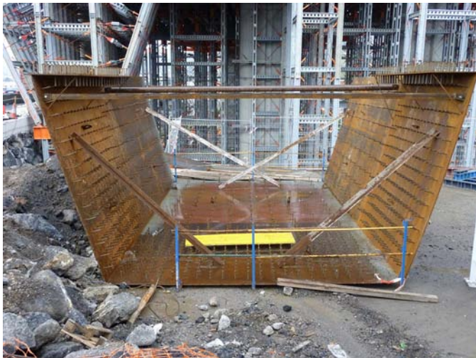
Figure 24. View of the connecting segment before being raised.
