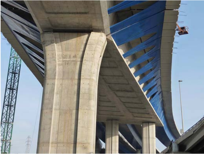
Figure 23. Lower view of the transition area.
