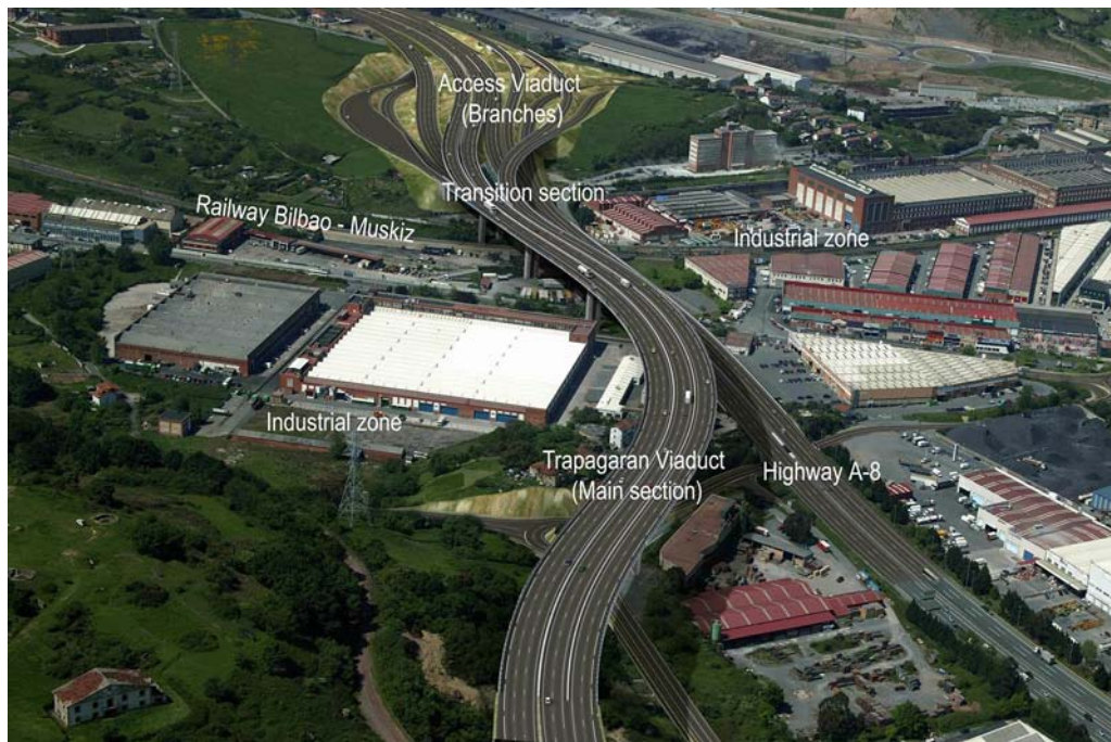
Figure 1. Virtual image of the area of the viaduct.
