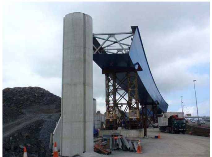
Figure 28. Piers of approach branches.
