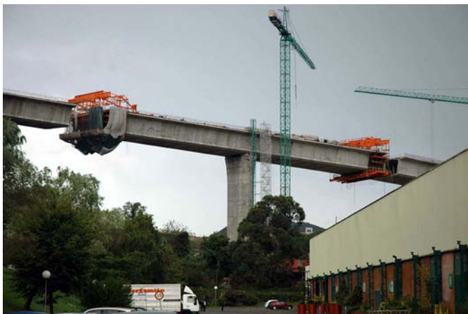
Figures 4 and 5. Views of constructing the core by balanced cantilever.
