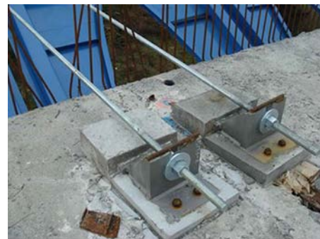
Figure 13. Main viaduct. Fixing blocks in the core.
