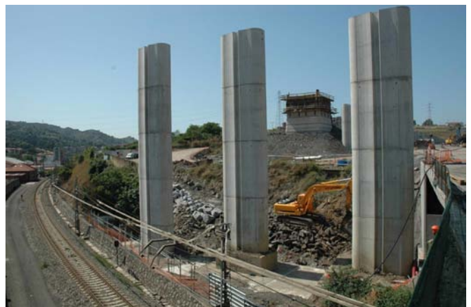
Figure 29. Piers in the transition area.
