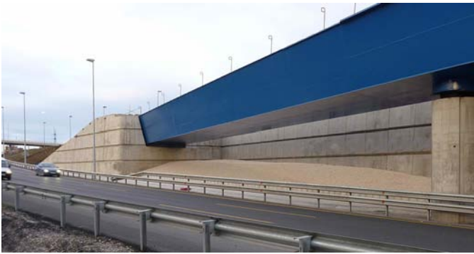
Figure 31. View of the abutments of the approach branches.
