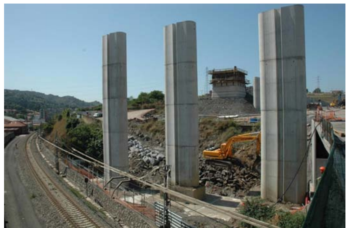
Figure 29. Piers in the transition area.
