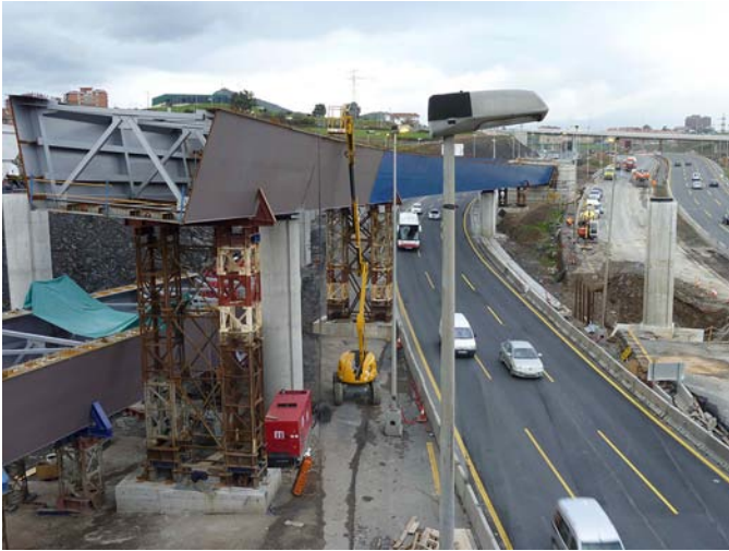
Figure 17. Approach viaduct. Steel stretches of branches B and C.
