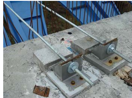
Figure 13. Main viaduct. Fixing blocks in the core.
