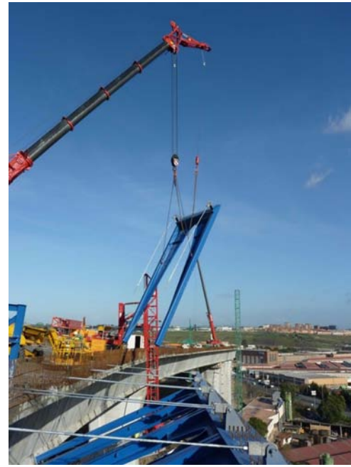
Figure 15. Main viaduct. Assembly of side brackets.
