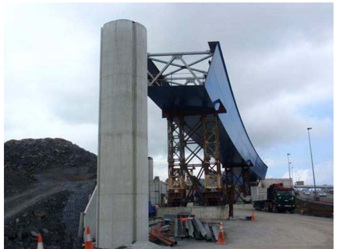
Figure 28. Piers of approach branches.
