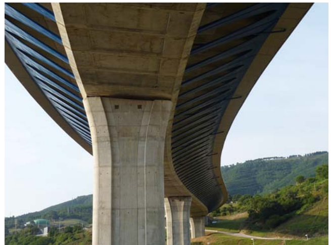
Figure 12. Main viaduct. Lower view.
