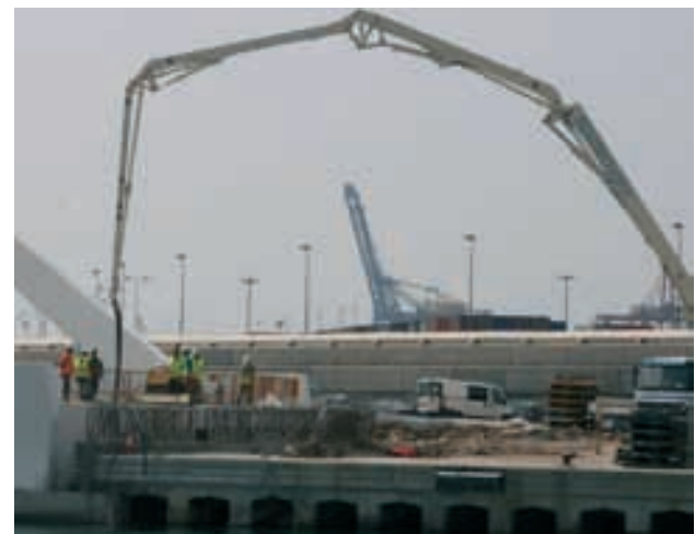
Figura 42. Hormigonado de contrapeso. Figure 42. Casting concrete in the counterweight.
