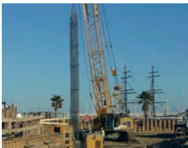
Figura 22. Ejecución de pantallas dorsales. Figure 22. Construction of rear diaphragm walls.
