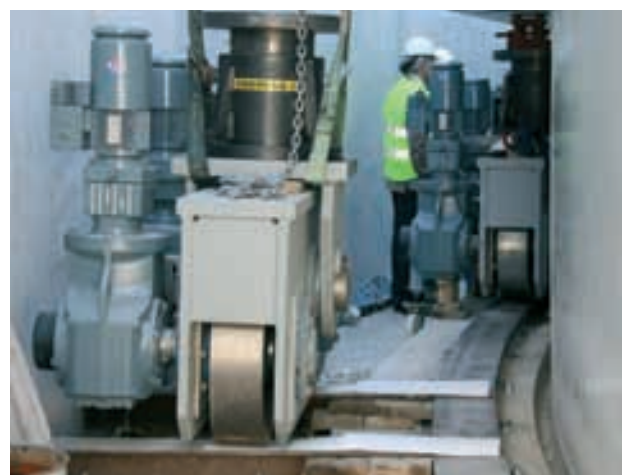
Figura 38. Colocación de carretones Figure 38. Traction wheel installation.
