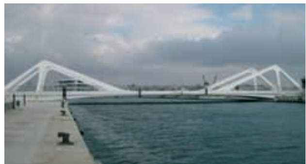
Figura 11. Puente cerrado. Hiperestatismo en servicio. Figure 11. Bridge closed. Static indeterminacy (bridge in service).
