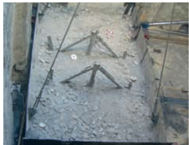
Figuras 27 y 28. Vaciado con retroexcavadora y descenso del contrapeso. Figures 27 and 28. Emptying counterweight with back hoe excavator and lowering counterweight into the pit.
