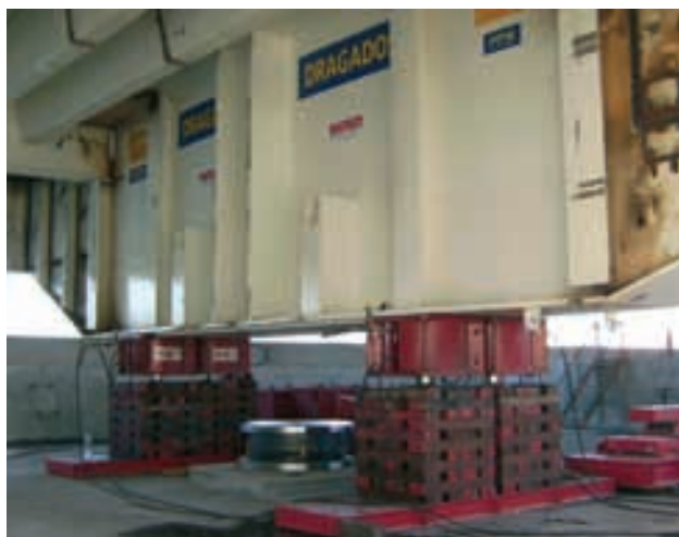
Figuras 40 y 41. Gateo y apoyo en rótula. Figures 40 and 41. Jacking and resting leaf on turntable.
