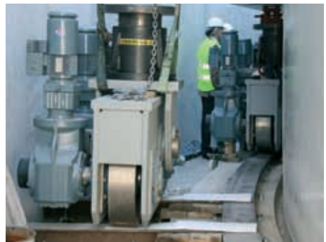
Figura 38. Colocación de carretones Figure 38. Traction wheel installation.
