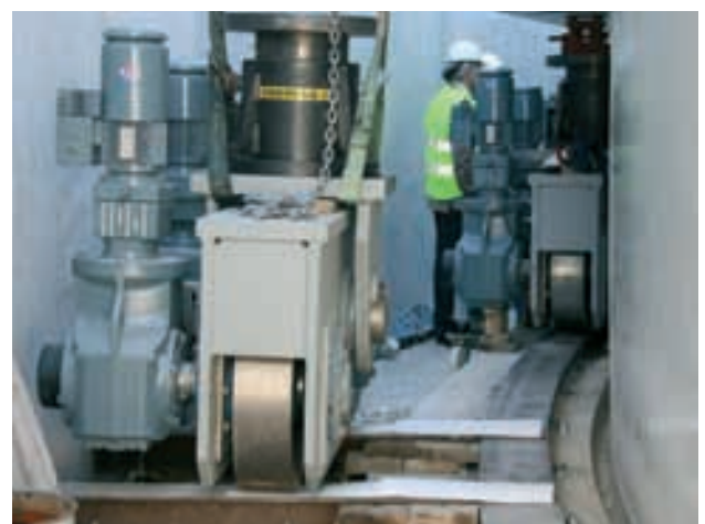
Figura 38. Colocación de carretones Figure 38. Traction wheel installation.
