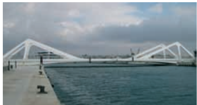
Figura 11. Puente cerrado. Hiperestatismo en servicio. Figure 11. Bridge closed. Static indeterminacy (bridge in service).
