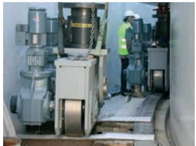
Figura 38. Colocación de carretones Figure 38. Traction wheel installation.
