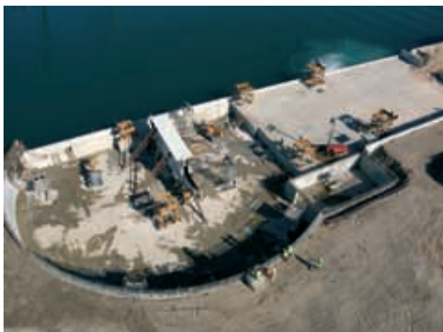
Figura 9. Recintos. Obra Civil. Figure 9. Pits. Civil works.
