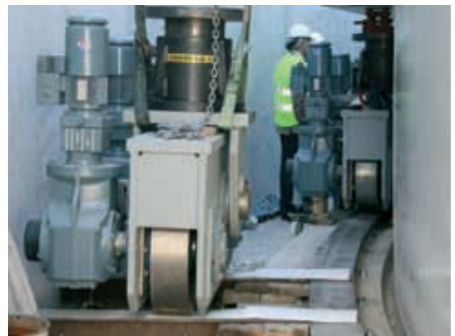
Figura 38. Colocación de carretones Figure 38. Traction wheel installation.
