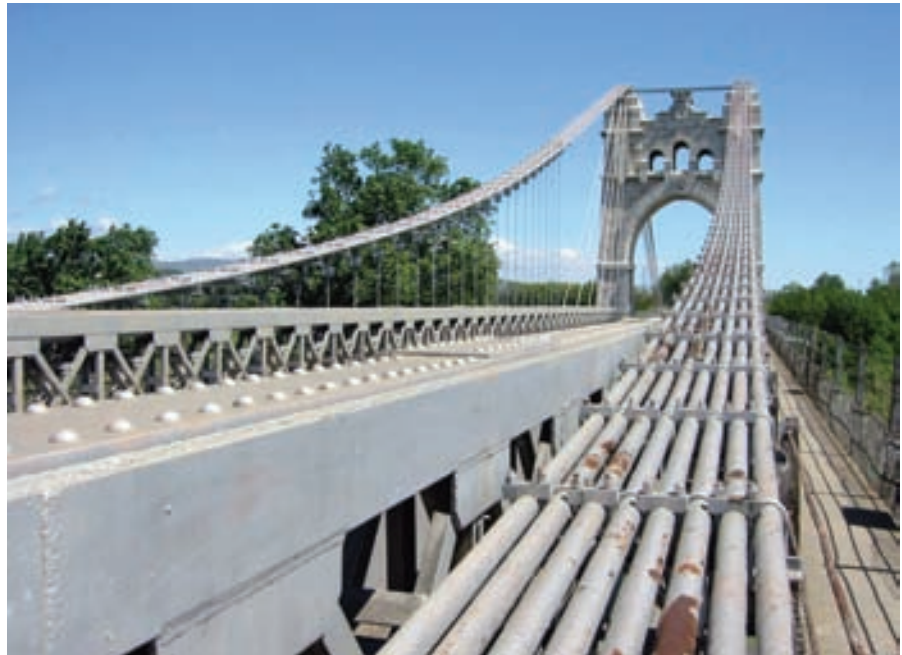
Figura 22. Cables principales. Figure 22. Main cables.
