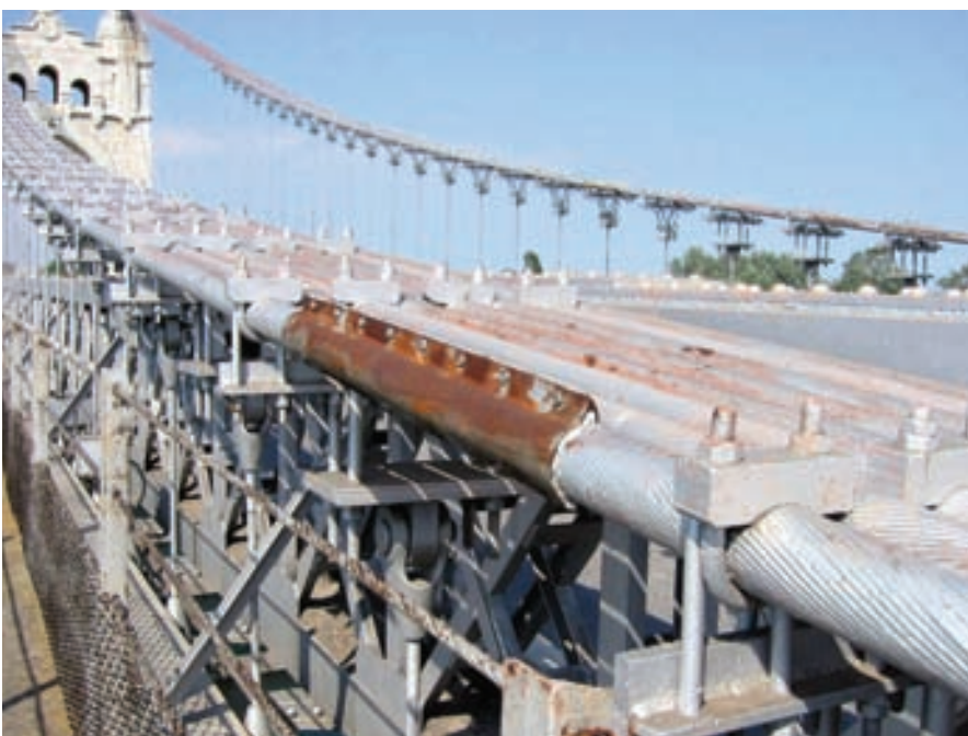
Figura 17. Cables reparados en 1972. Figure 17. Cables repaired in 1972.
