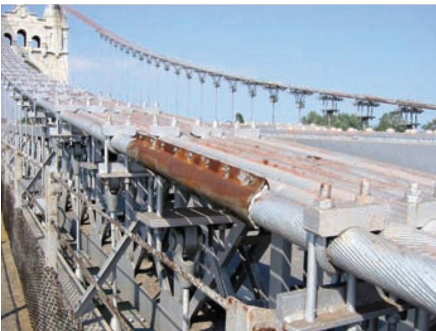
Figura 17. Cables reparados en 1972. Figure 17. Cables repaired in 1972.
