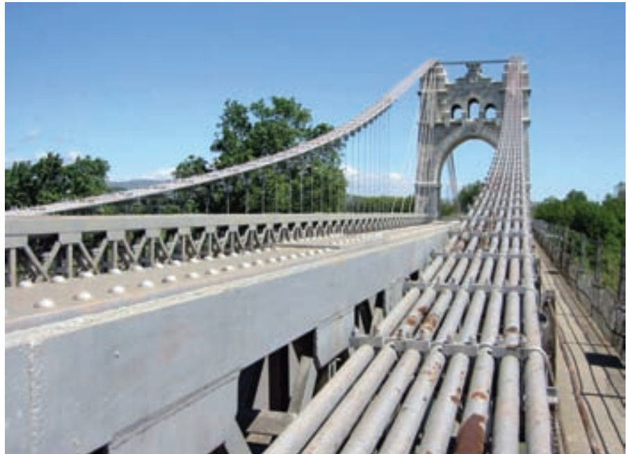
Figura 22. Cables principales. Figure 22. Main cables.
