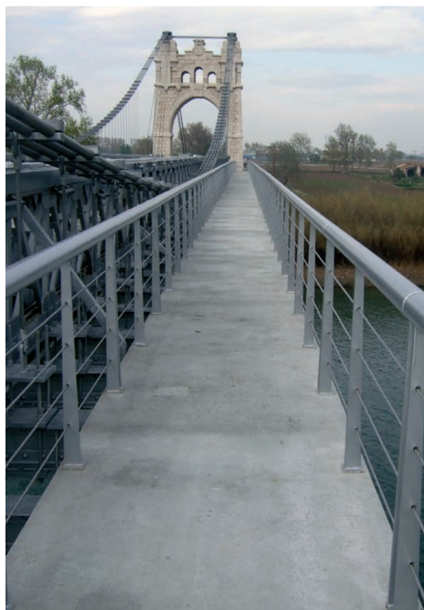
Figura 40. Nueva acera terminada. Figure 40. Finished walkway.
