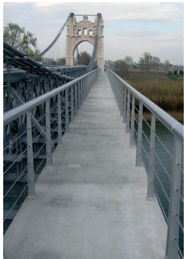
Figura 40. Nueva acera terminada. Figure 40. Finished walkway.
