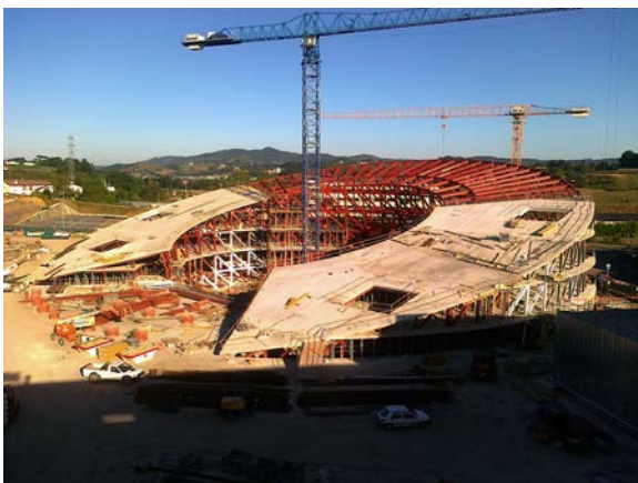
Figure 11. Construction of structural roof slab.
