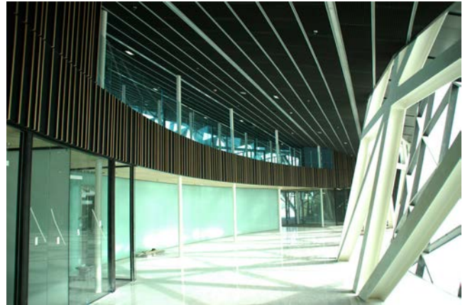
Figure 29. Indoor view of building showing inner truss and two rows of inner columns.
