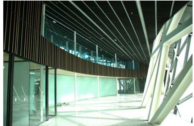
Figure 29. Indoor view of building showing inner truss and two rows of inner columns.
