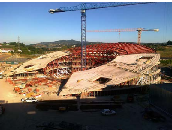
Figure 11. Construction of structural roof slab.
