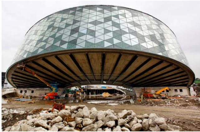
Figure 28. Front view of tower after construction of façade.
