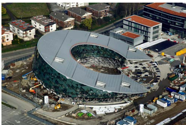
Figure 4. Aerial view of the roof.
