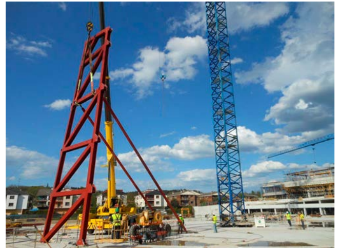
Figure 24. Hoisting the first truss panel: note the provisional props used to stabilise the structure during erection.
