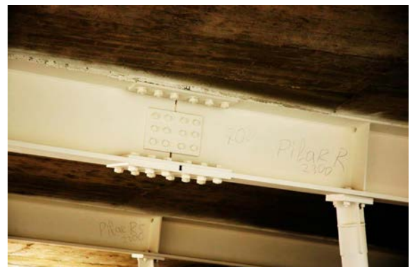
Figure 22. Bolted beam and beam-column joints.
