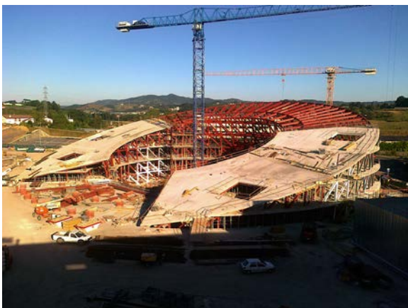
Figure 11. Construction of structural roof slab.
