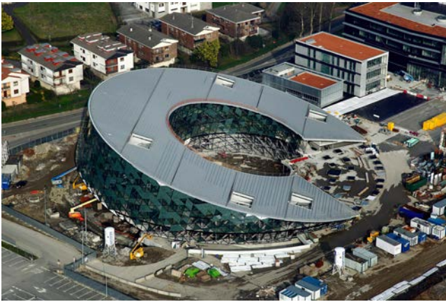
Figure 4. Aerial view of the roof.
