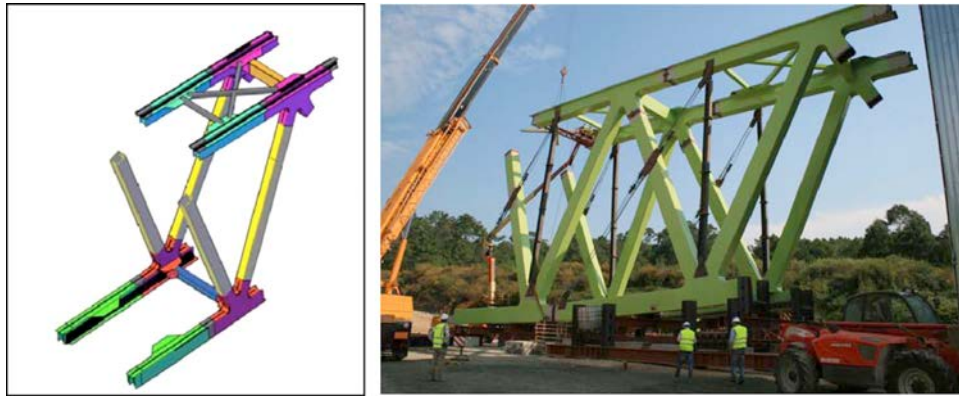
Figure 33. Segment breakdown into components and two segments assembled on the ground.
