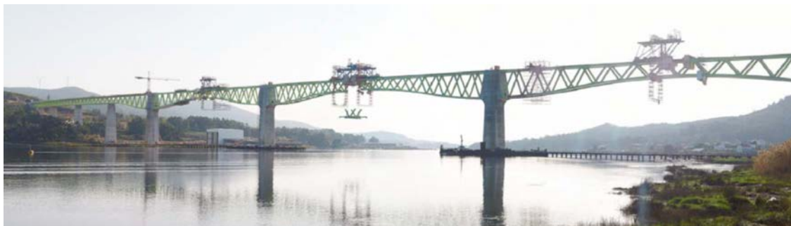
Figure 44. Hoisting the joining segment for span 7.
