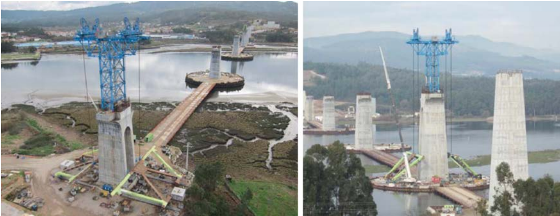
Figure 30. Zero segment construction and uprighting at the foot of the pier.
