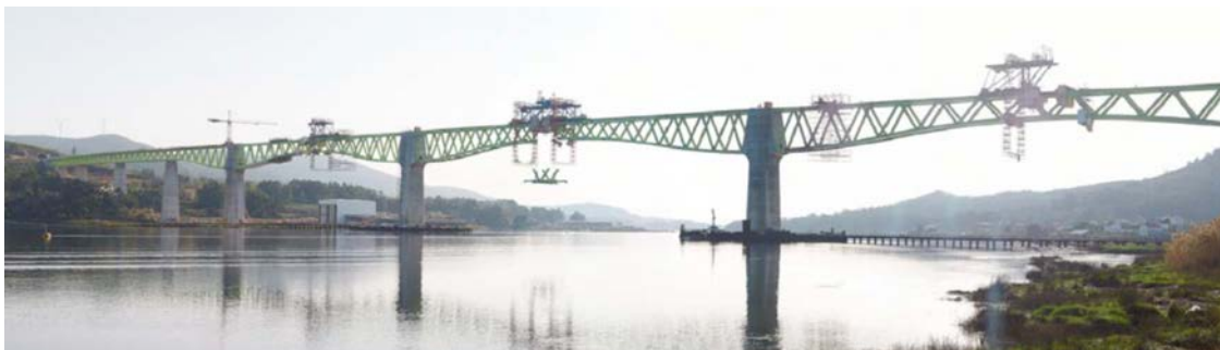
Figure 44. Hoisting the joining segment for span 7.
