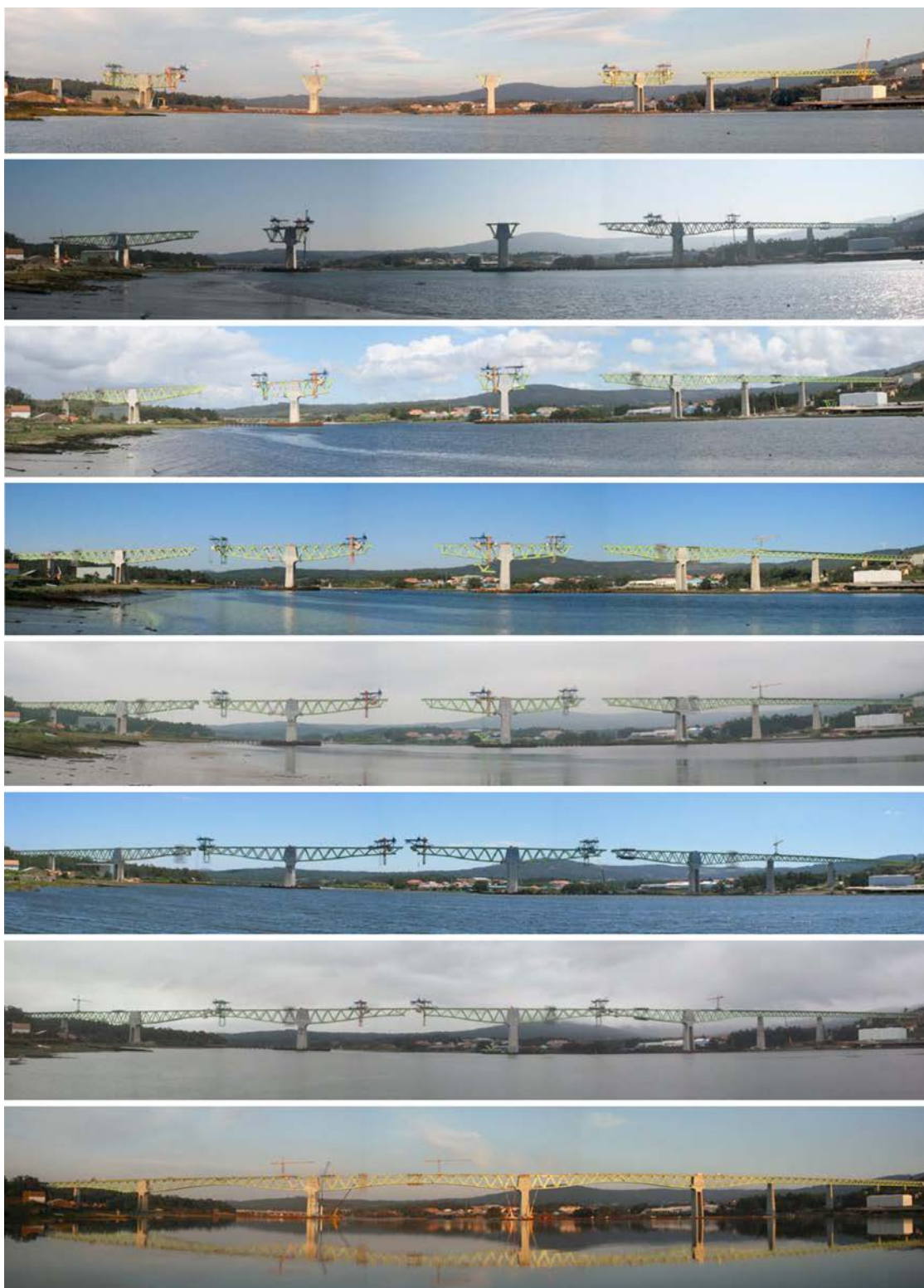
Figure 39. Balanced cantilevering from P5 (right) and P8 (left) and subsequently from P6 and P7.
