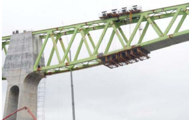
Figure 45. Travelling formwork for casting bottom slab concrete.
