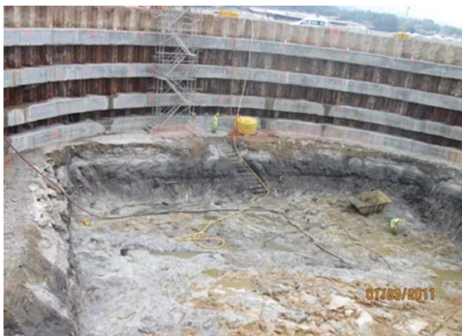
Figure 11. Rocky substratum under P7 prior to pouring the blinding.
