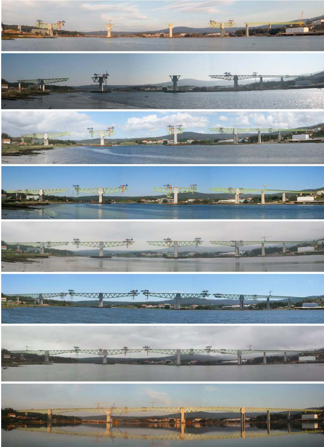
Figure 39. Balanced cantilevering from P5 (right) and P8 (left) and subsequently from P6 and P7.
