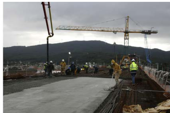
Figure 46. Laying full-width precast slabs and concrete casting on the upper slab.
