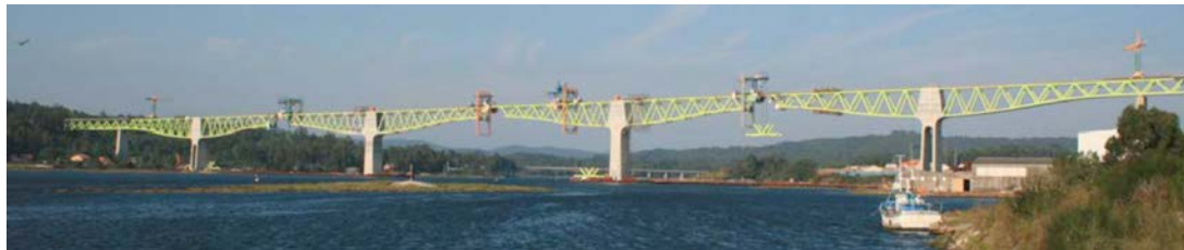
Figure 42. Hoisting the joining segment for span 6.
