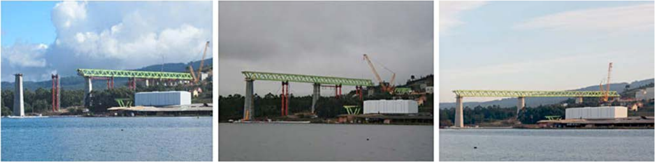
Figure 24. Second stage, 240-m section launched between P3 and P4, and hoisting segments in stage 3.
