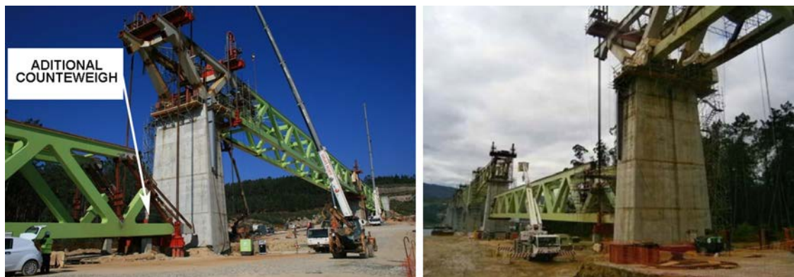
Figure 28. Hoisting sequence for spans 11 (left) and 10 (right).
