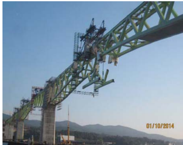
Figure 43. Hoisting the joining segment for span 8.
