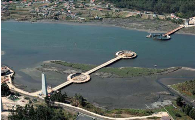
Figure 5. Wharf and foundation enclosures for riverbed piers P5, P6 and P7.
