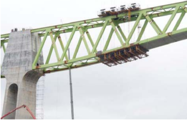
Figure 45. Travelling formwork for casting bottom slab concrete.
