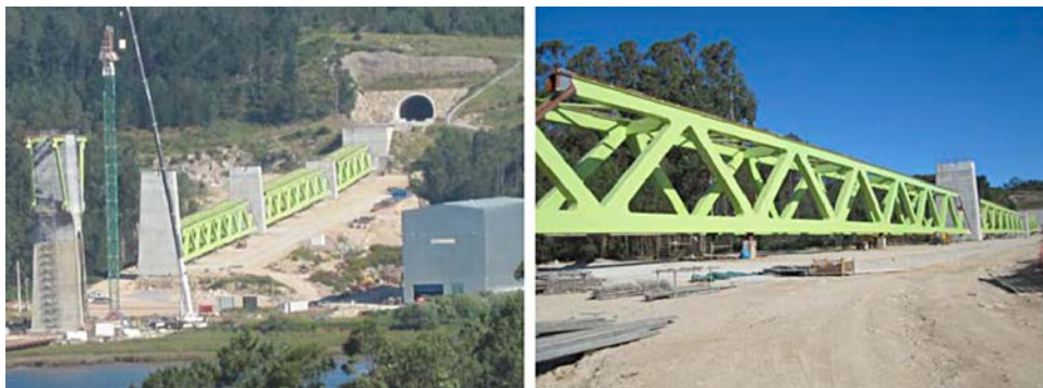
Figure 26. Sections for spans 10–12 built on the ground, ready for hoisting.
