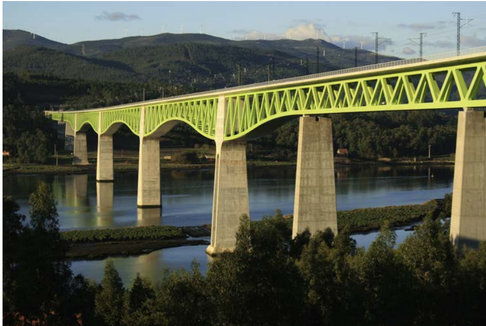
Figure 48. Finished viaduct, side view.
