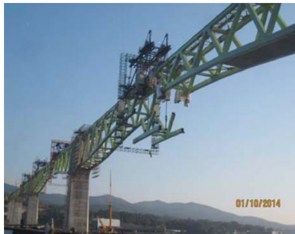
Figure 43. Hoisting the joining segment for span 8.
