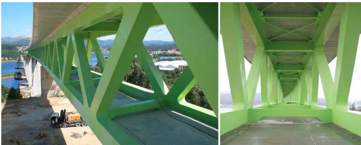
Figure 4. Side view and interior of the truss viewed from the bottom concrete slab.
