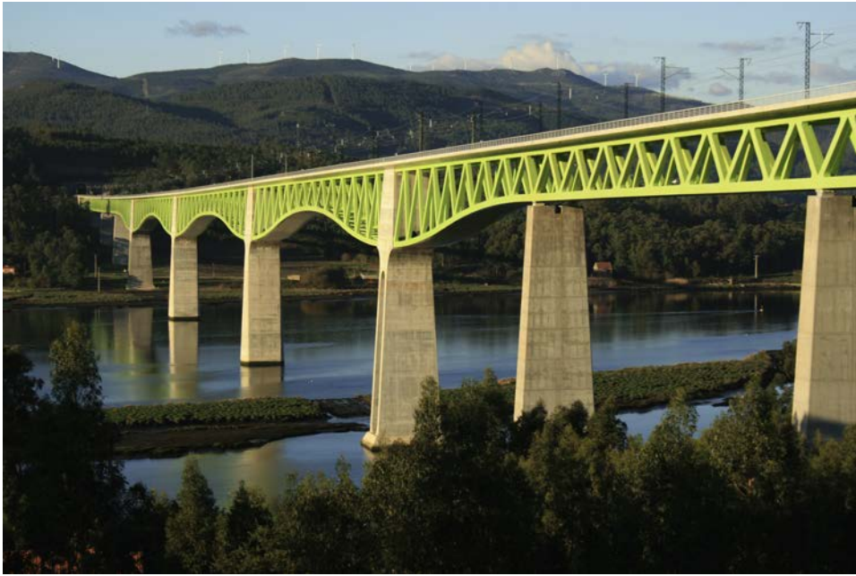
Figure 48. Finished viaduct, side view.
