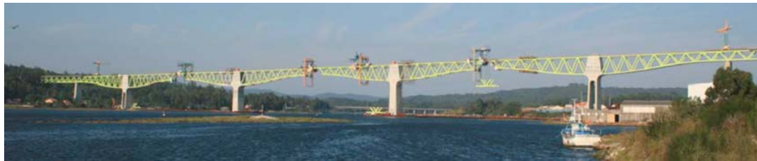
Figure 42. Hoisting the joining segment for span 6.
