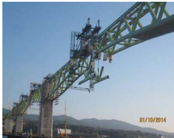
Figure 43. Hoisting the joining segment for span 8.
