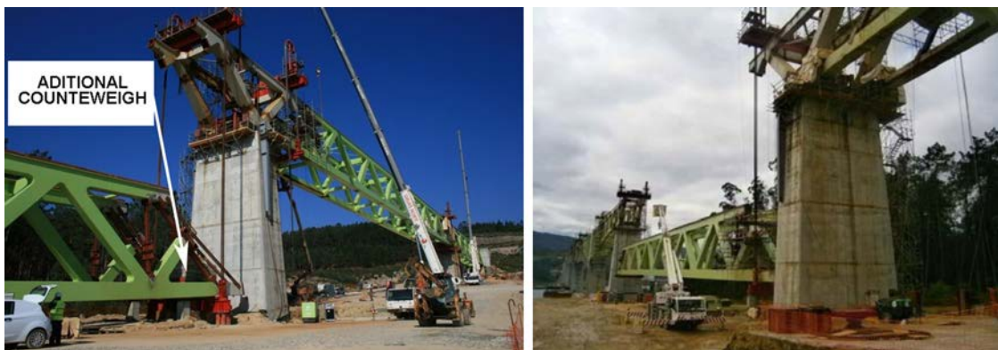
Figure 28. Hoisting sequence for spans 11 (left) and 10 (right).
