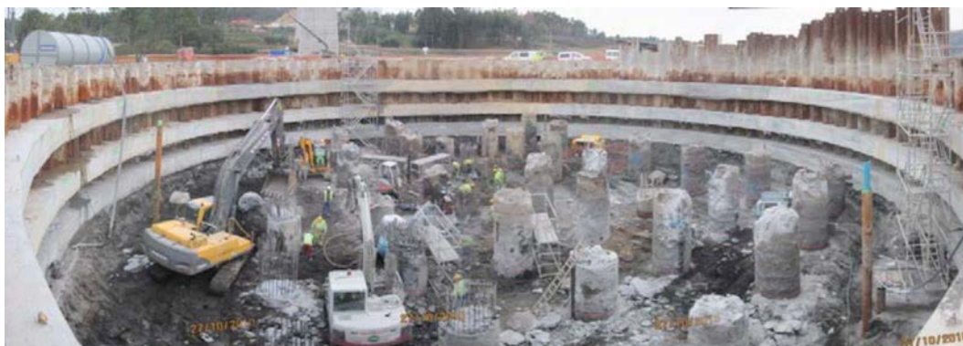
Figure 9. Cutting down P5 foundation pile heads.
