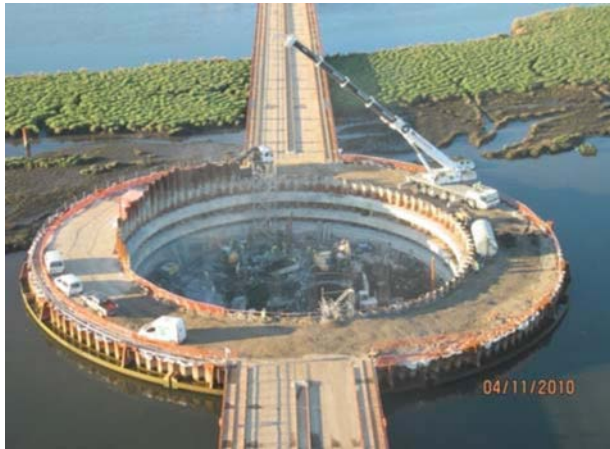
Figure 8. Inner excavation in P5 enclosure.
