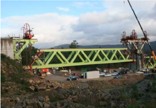
Figure 27. Hoisting sequence for 465-t approach span 12 between A2 and P11.
