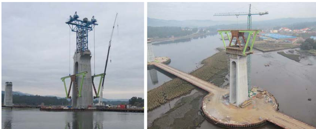
Figure 31. Hoisting zero segment and positioning on pierhead.
