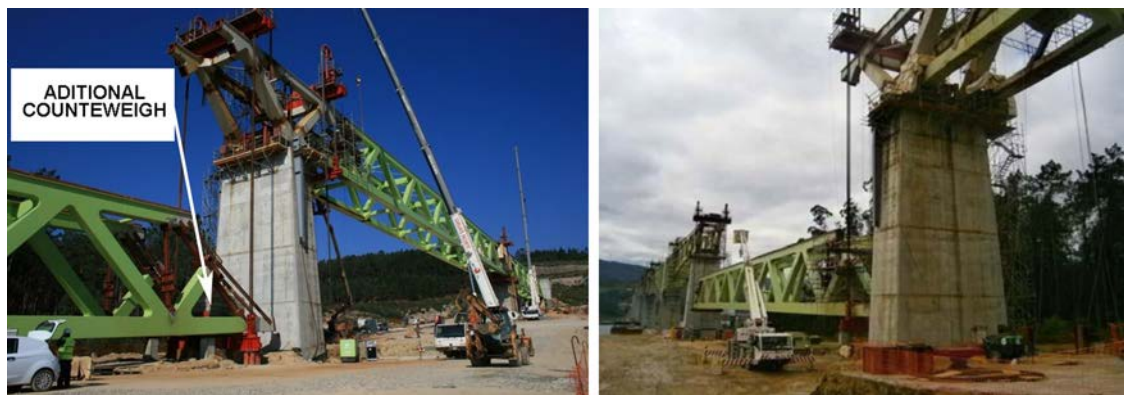
Figure 28. Hoisting sequence for spans 11 (left) and 10 (right).
