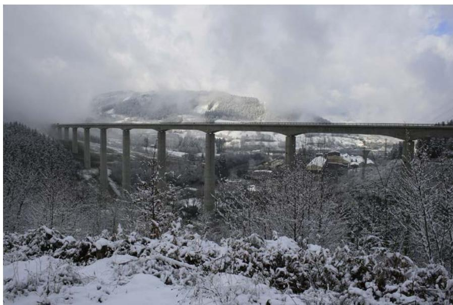
Figure 43. Viaduct during load test with lorries (4 February 2015).
