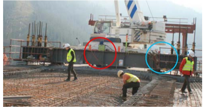
Figure 33. Transverse hanger beam; left circle: strain gauges on webs at mid-span; right circle: strain gauges on web alongside support.
