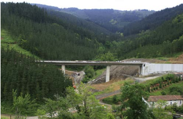
Figure 4. Olzaileko Brook Viaduct.
