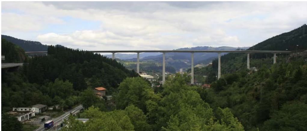
Figure 11. View of finished prestressed concrete viaduct.
