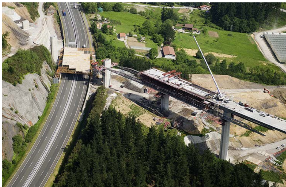
Figure 25. Overview of area of negative reinforcement completely cast in concrete and laying of precast slabs in the positive reinforcement section, for subsequent assembly and concrete casting of the top slab rebar.
