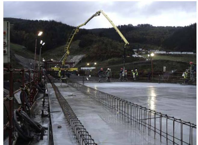
Figure 24. Casting the top slab with concrete pumped from the forward end of the preceding phase.
