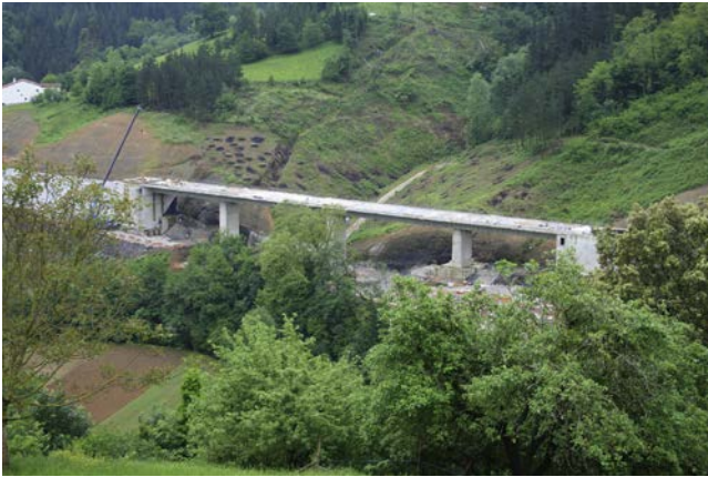
Figure 3. Altzeta Brook Viaduct.
