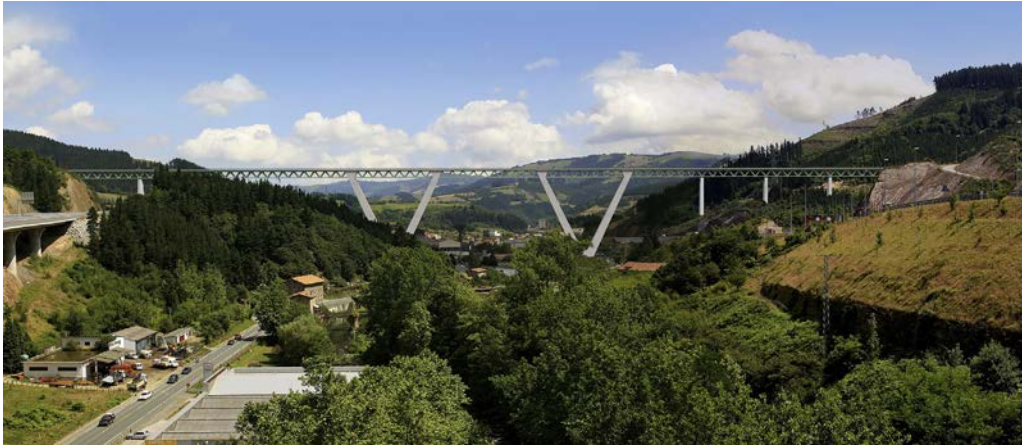
Figure 5. Simulation of the composite truss bridge with two V-shaped piers that won the 2007 ideas competition.
