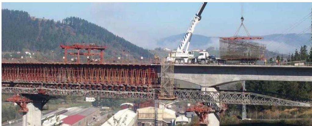
Figure 29. Positioning pre-assembled reinforcement on deck.
