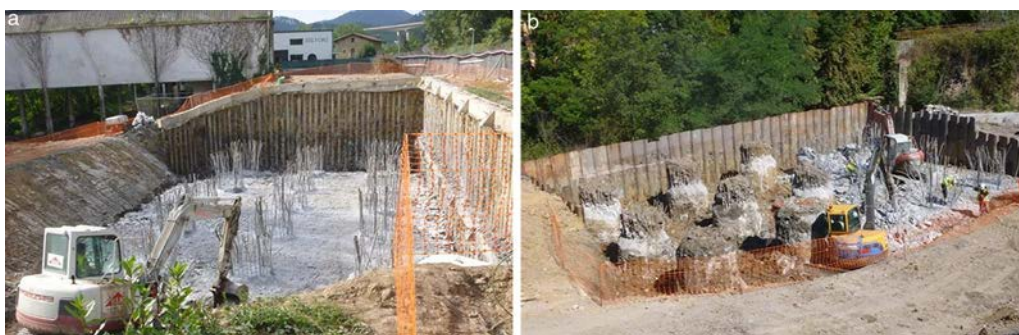
Figure 16. a) Micropile retaining walls for P-7 foundations; b) sheet retaining wall for P-8 pile foundations.
