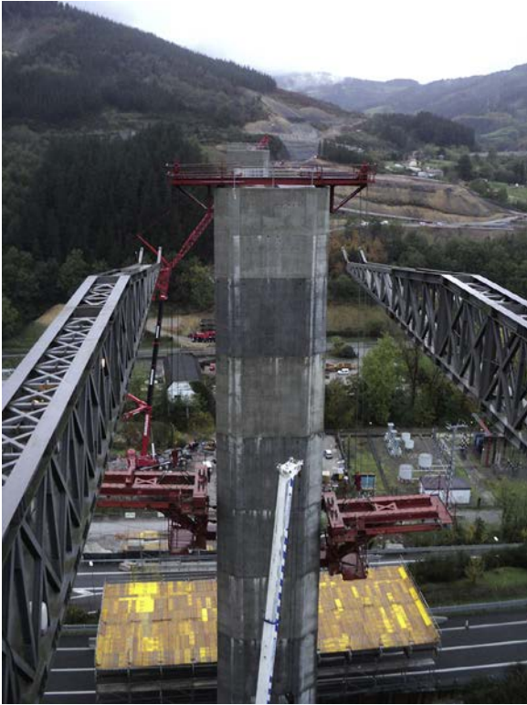
Figure 31. Lifting the ring brackets to support the MSS.
