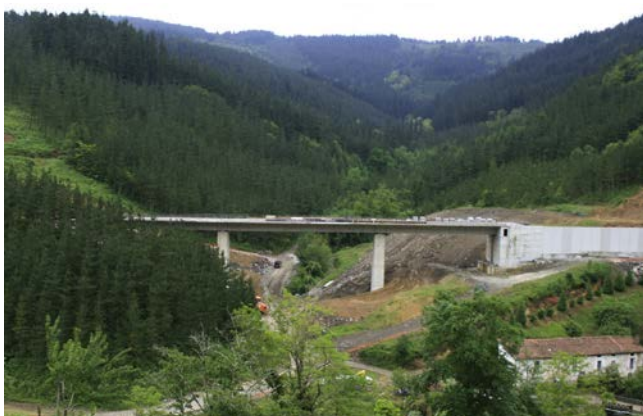
Figure 4. Olzaileko Brook Viaduct.
