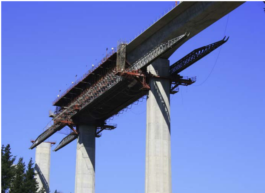
Figure 32. MSS support rings at top of pier.
