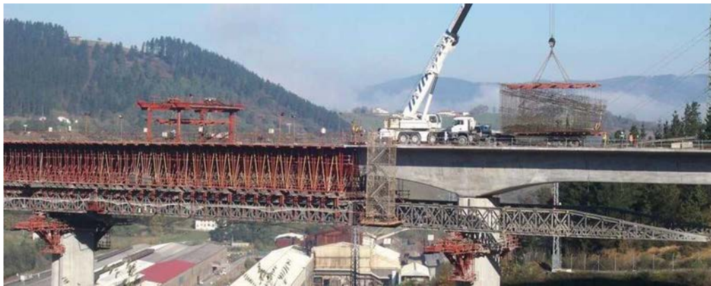
Figure 29. Positioning pre-assembled reinforcement on deck.
