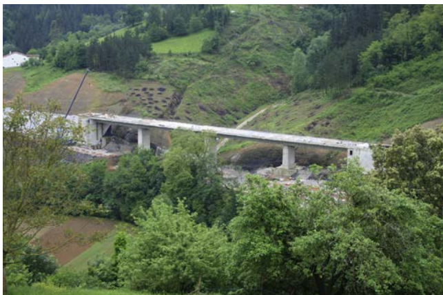
Figure 3. Altzeta Brook Viaduct.
