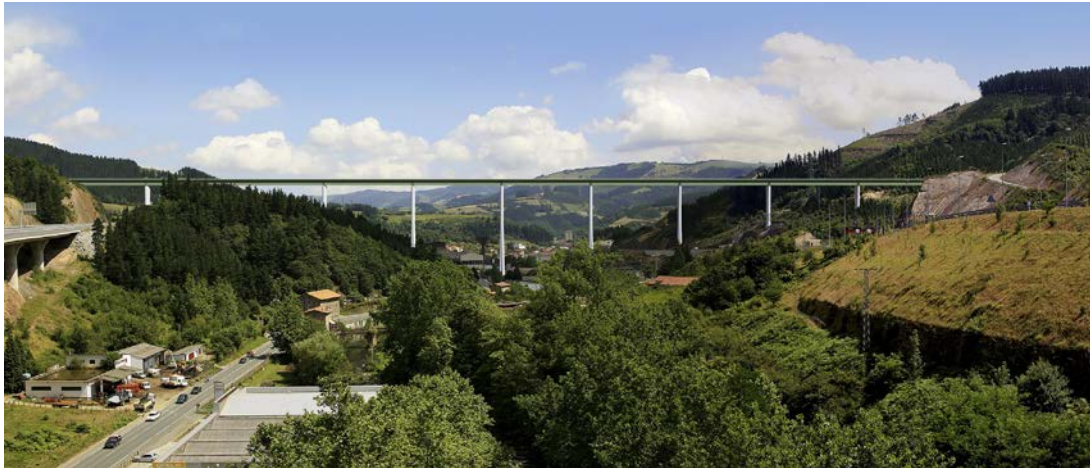
Figure 8. Simulation of composite closed web solution.
