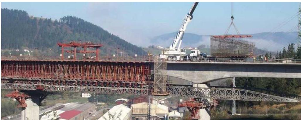
Figure 29. Positioning pre-assembled reinforcement on deck.
