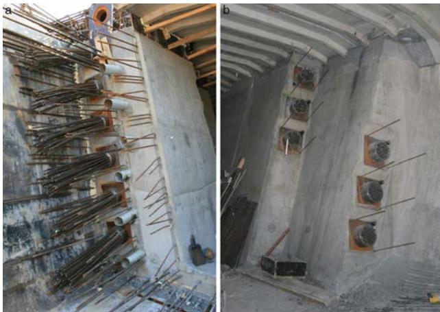
Figure 28. Continuity tendon anchorages and crosslinked wires and active anchorages at cantilever front; passive steel anchorages.
