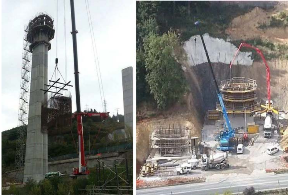
Figure 19. Reinforcing steel preassembly and lifting and concrete pumping for one cycle.
