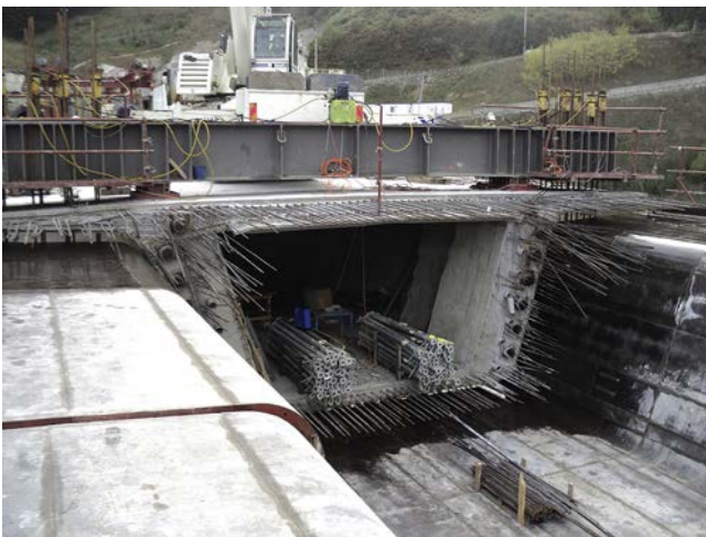
Figure 26. Cantilever front with anchorages for negative reinforcement tendons and parabolic continuity tendons and the system for hanging the MSS from the end of the cantilever.
