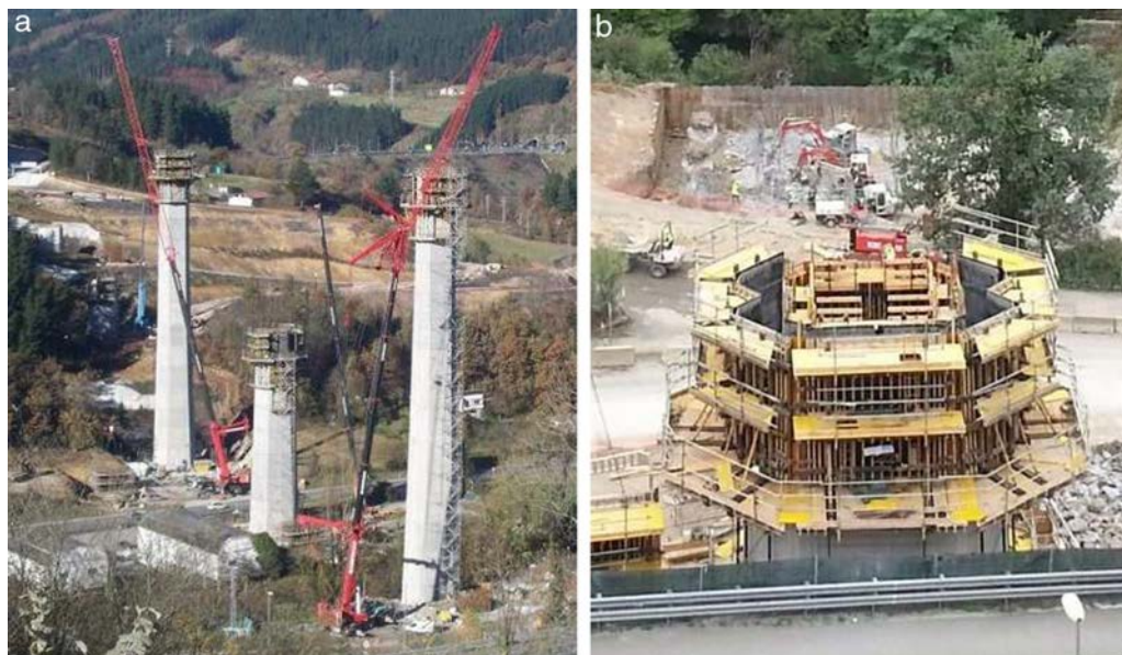
Figure 18. Overview and detail of the climbing forms for piers.
