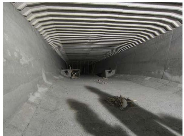
Figure 27. Inside of deck with anchorages for positive reinforcement prestressing in background.
