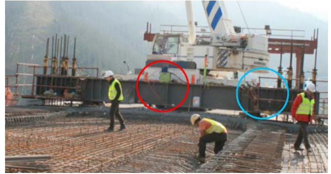
Figure 33. Transverse hanger beam; left circle: strain gauges on webs at mid-span; right circle: strain gauges on web alongside support.
