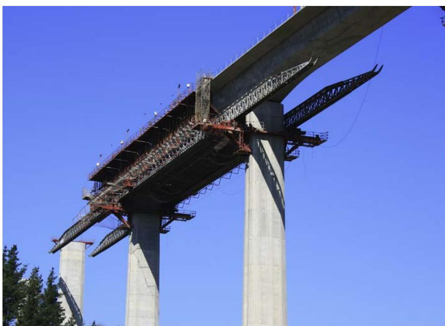
Figure 32. MSS support rings at top of pier.
