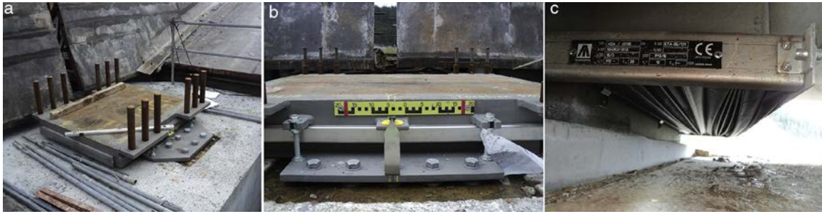
Figure 13. Bearing, ruler-based measuring system and dust cover.
