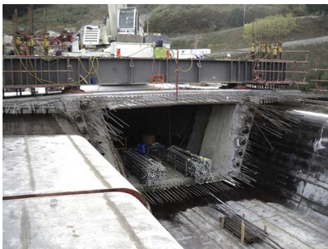
Figure 26. Cantilever front with anchorages for negative reinforcement tendons and parabolic continuity tendons and the system for hanging the MSS from the end of the cantilever.
