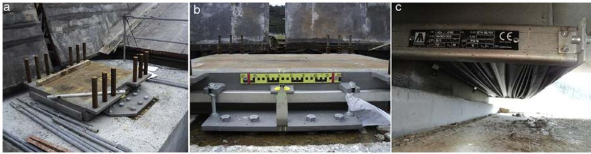
Figure 13. Bearing, ruler-based measuring system and dust cover.
