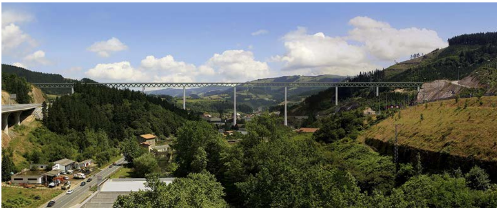
Figure 6. Simulation of composite truss solution with vertical piers chosen by ETS on the grounds of the typology study.
