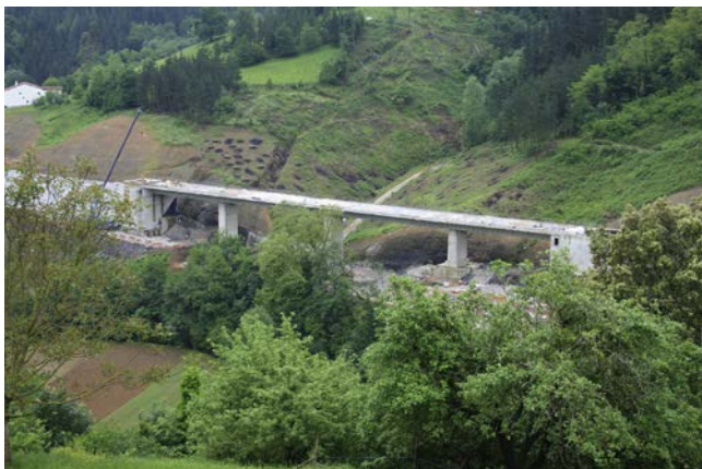
Figure 3. Altzeta Brook Viaduct.
