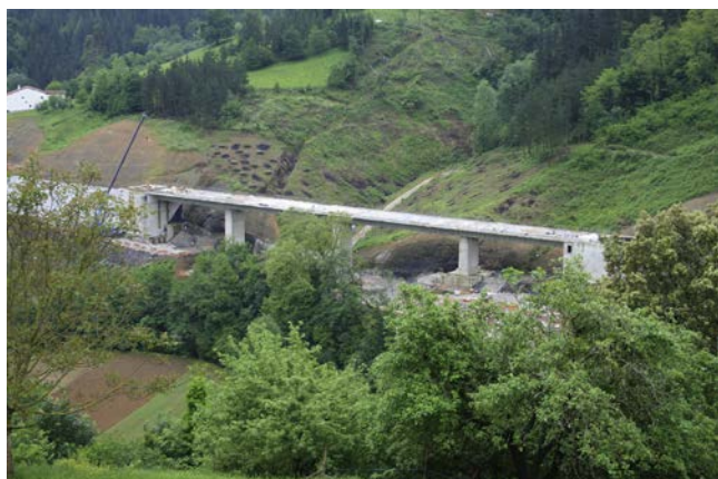
Figure 3. Altzeta Brook Viaduct.
