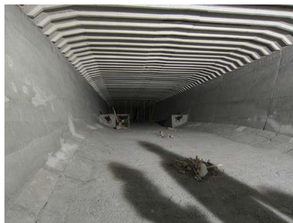
Figure 27. Inside of deck with anchorages for positive reinforcement prestressing in background.
