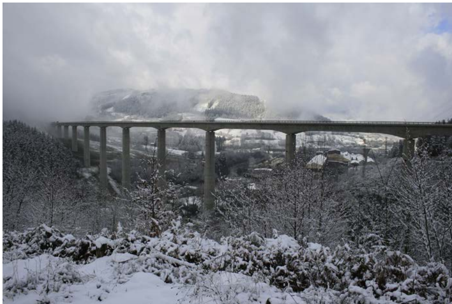
Figure 43. Viaduct during load test with lorries (4 February 2015).
