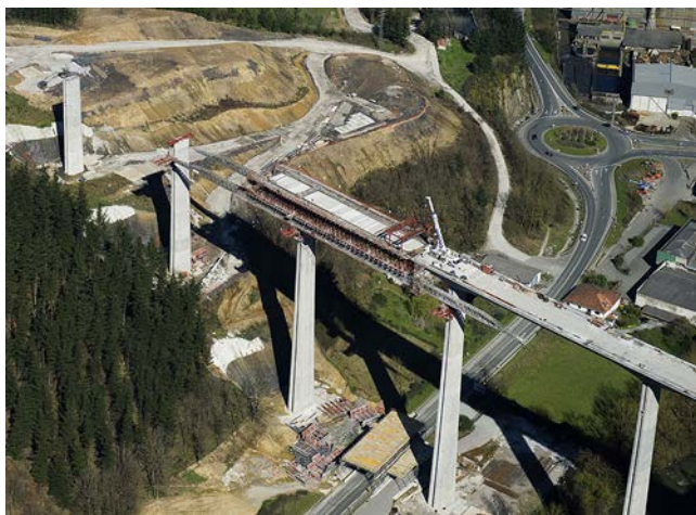
Figure 23. Laying of precast slabs on previously cast trough.
