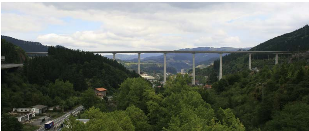
Figure 11. View of finished prestressed concrete viaduct.
