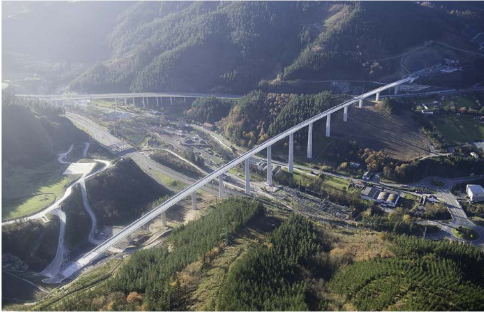
Figure 1. Finished River Deba Viaduct.
