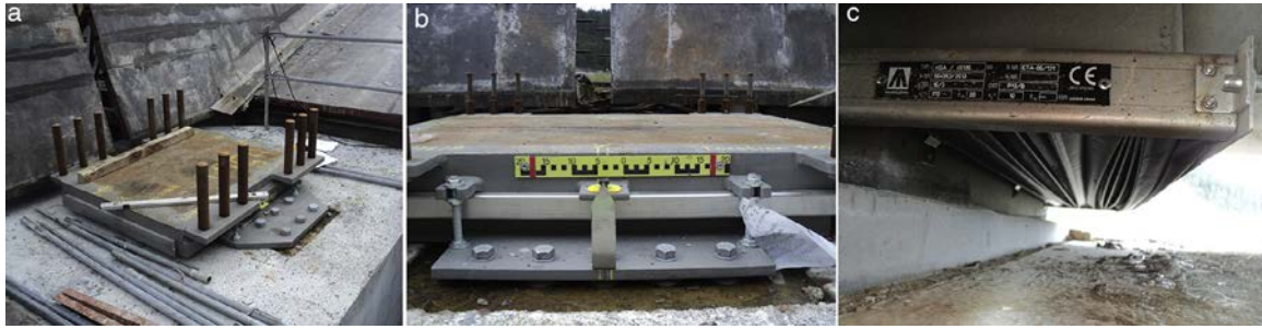
Figure 13. Bearing, ruler-based measuring system and dust cover.
