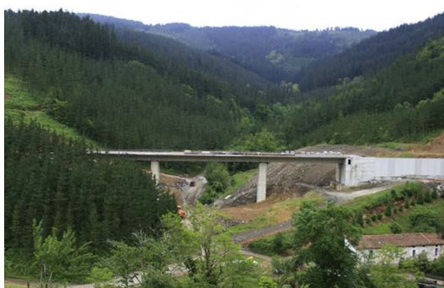
Figure 4. Olzaileko Brook Viaduct.
