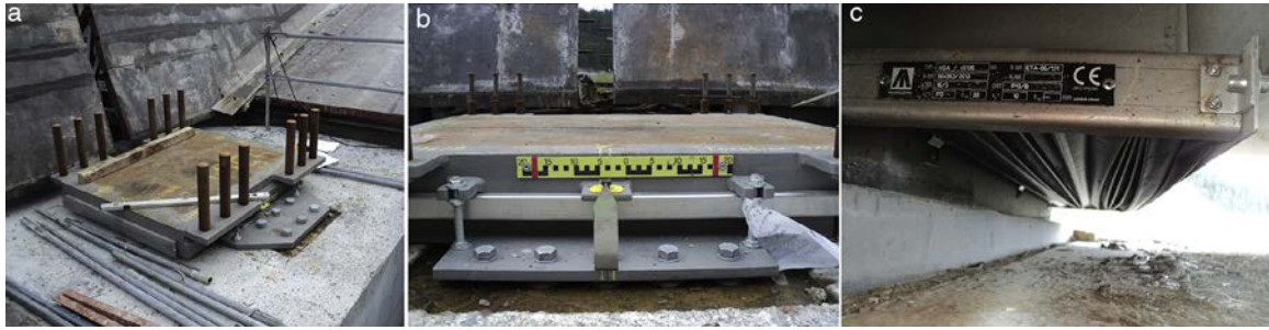
Figure 13. Bearing, ruler-based measuring system and dust cover.
