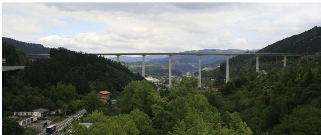
Figure 11. View of finished prestressed concrete viaduct.
