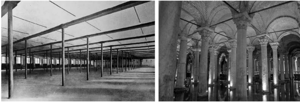
Figure 17. Plasteres panelled vaults in the Batlló factory, Barcelona (R. Guastavino, 1875) and the Basilica Cistern in Istanbul (532 A.C.) (right).
