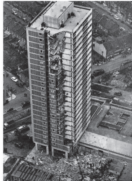
Figure 1. Partial collapse of the Ronan Point tower on May 16th 1968. London [2].
