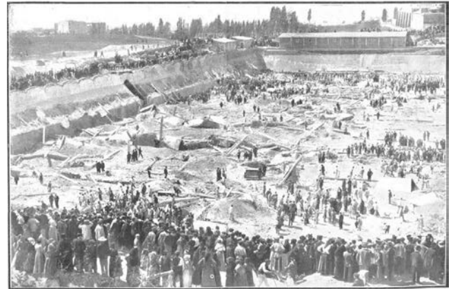
Figure 3. General view of the disaster area ( Nuevo Mundo , April 1905).
