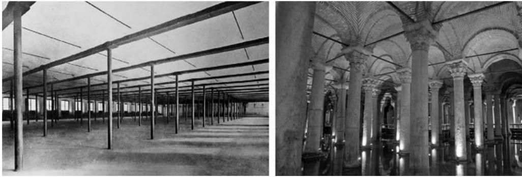
Figure 17. Plasteres panelled vaults in the Batlló factory, Barcelona (R. Guastavino, 1875) and the Basilica Cistern in Istanbul (532 A.C.) (right).
