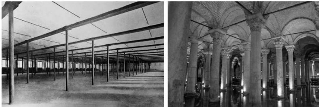
Figure 17. Plastered panelled vaults in the Batlló factory, Barcelona (R. Guastavino, 1875) and the Basilica Cistern in Istanbul (532 A.C.) (right).
