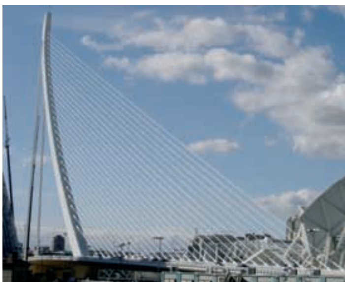
Figura 32. Tirantes y retenida ya tesados. Figure 32. Deck stays and back stays already stressed.
