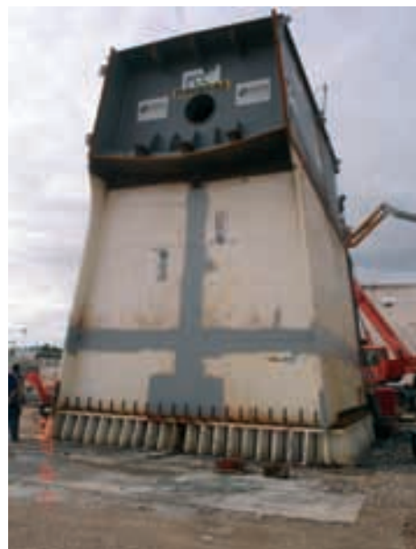
Figura 21. Base. Figure 21. Pier.
