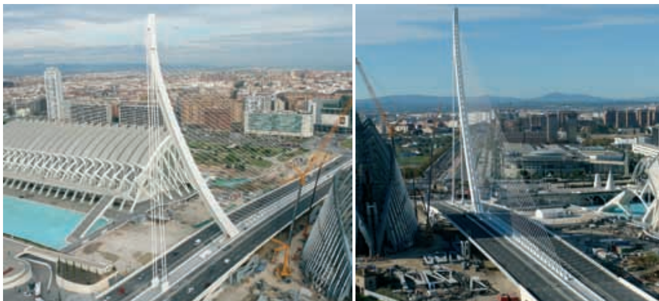
Figura 1. Vistas generales del puente. Figure 1. General view of the bridge.
