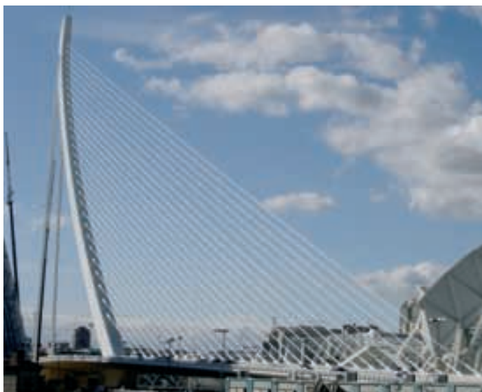
Figura 32. Tirantes y retenida ya tesados. Figure 32. Deck stays and back stays already stressed.
