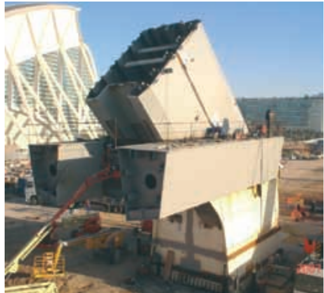
Figura 23. Unión de pilono, tablero y base. Figure 23. Connection of deck, pier and pylon.
