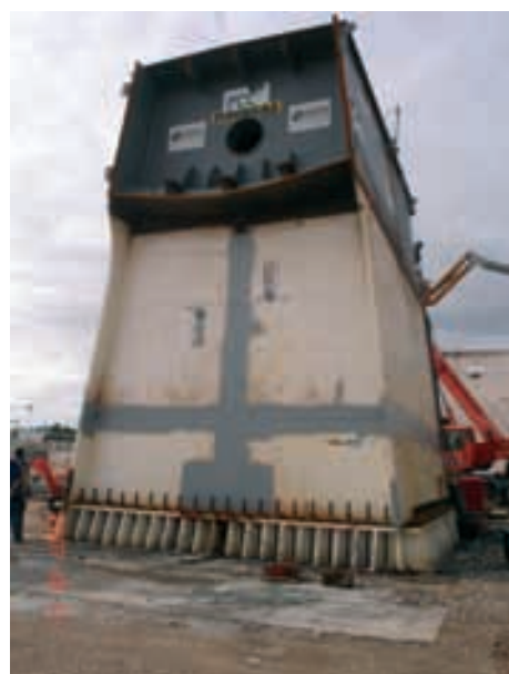
Figura 21. Base. Figure 21. Pier.
