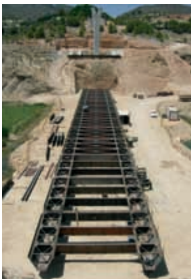
Figura 13. Bowstring (I). Tablero Figure 13. Bowstring (I). Deck
