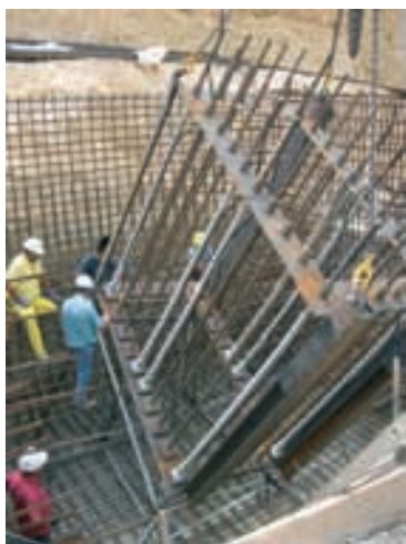
Figura 44. Replanteo de barras Figure 44. Bar stake-out
