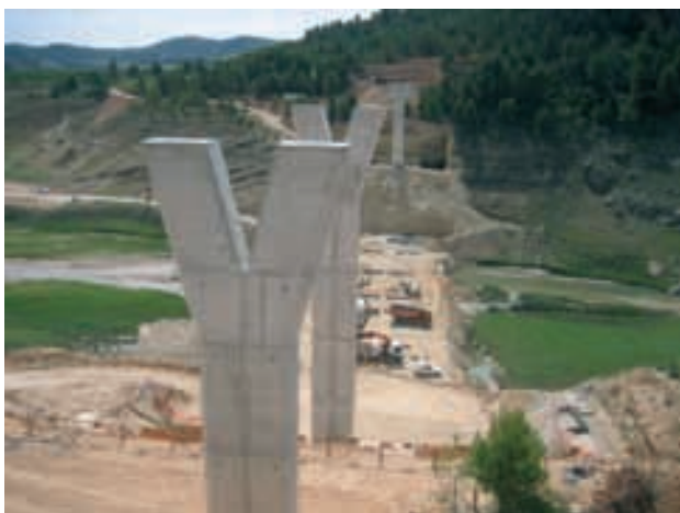
Figura 9. Pilas y plataforma del bowstring Figure 9. Piers and bowstring platform
