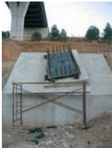
Figura 45. Replanteo placa apoyo Figure 45. Support plate stake-out
