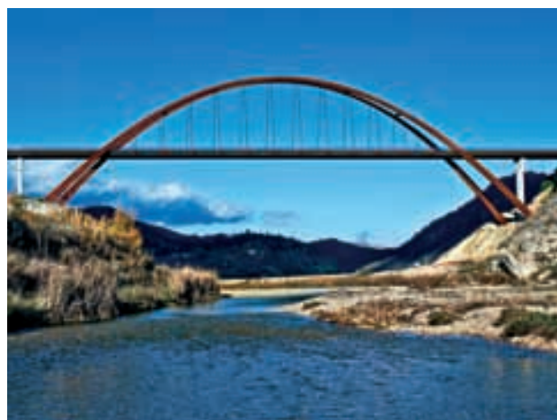
Figura 4B. Vista desde el río Figure 4B. View from the river
