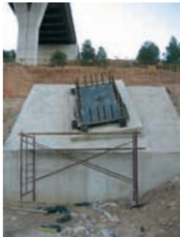
Figura 45. Replanteo placa apoyo Figure 45. Support plate stake-out
