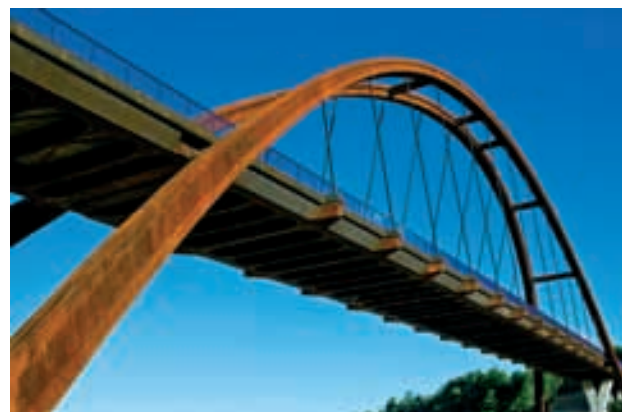
Figura 56. Acabados (II) Figure 56. Finishes (II)
