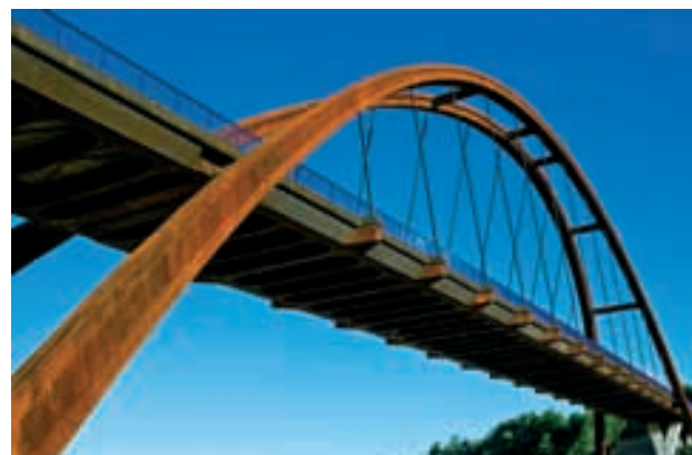
Figura 56. Acabados (II) Figure 56. Finishes (II)
