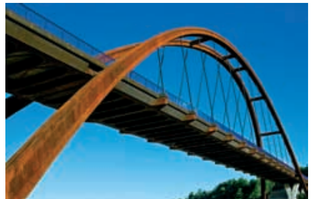
Figura 56. Acabados (II) Figure 56. Finishes (II)
