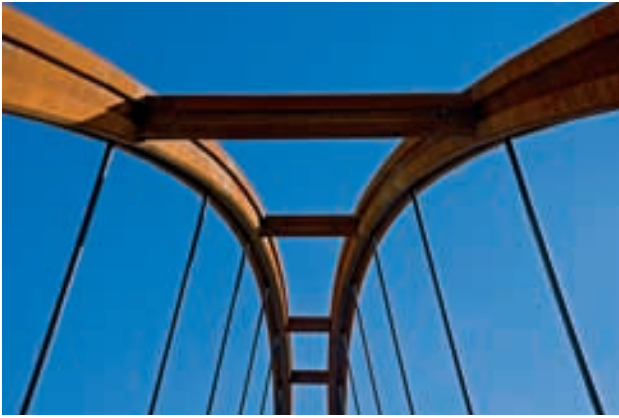
Figura 55. Acabados (I) Figure 55. Finishes (I)
