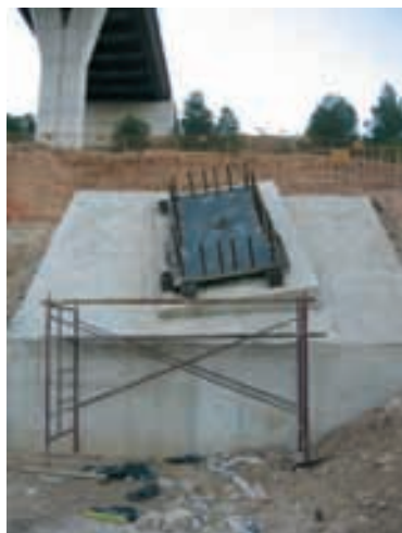
Figura 45. Replanteo placa apoyo Figure 45. Support plate stake-out
