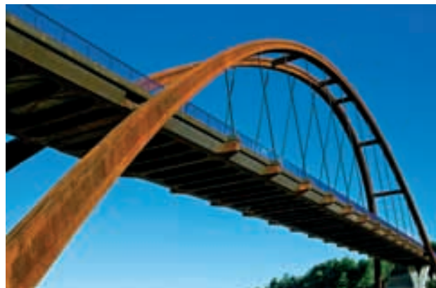
Figura 56. Acabados (II) Figure 56. Finishes (II)
