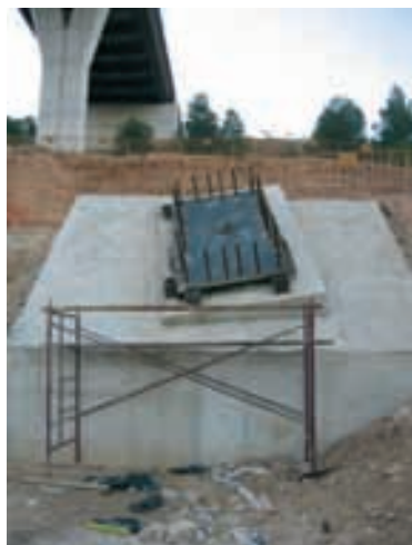
Figura 45. Replanteo placa apoyo Figure 45. Support plate stake-out
