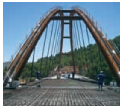
Figura 27. Hormigonado del tablero Figure 27. Laying concrete on the deck
