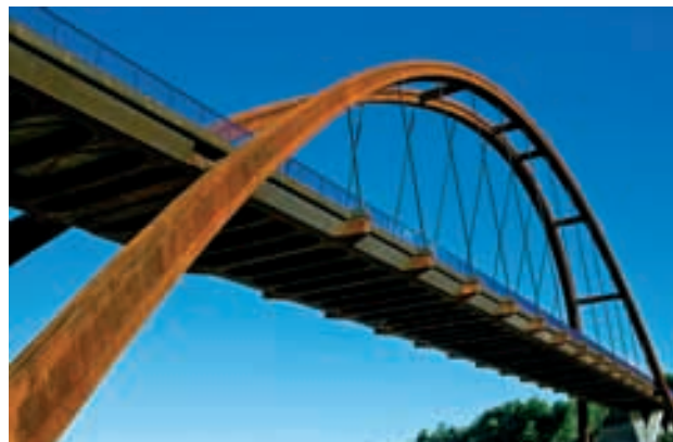
Figura 56. Acabados (II) Figure 56. Finishes (II)
