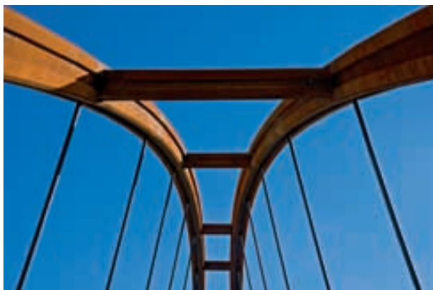
Figura 55. Acabados (I) Figure 55. Finishes (I)
