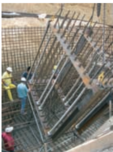
Figura 44. Replanteo de barras Figure 44. Bar stake-out
