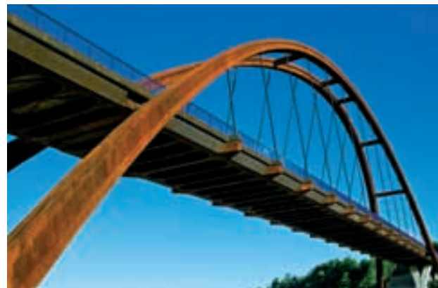
Figura 56. Acabados (II) Figure 56. Finishes (II)
