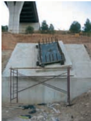
Figura 45. Replanteo placa apoyo Figure 45. Support plate stake-out
