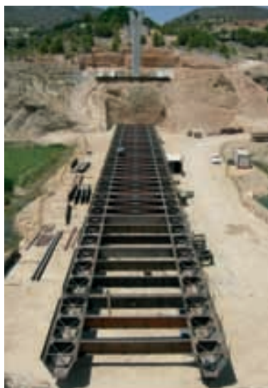
Figura 13. Bowstring (I). Tablero Figure 13. Bowstring (I). Deck
