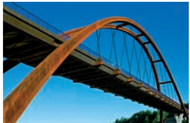
Figura 56. Acabados (II) Figure 56. Finishes (II)
