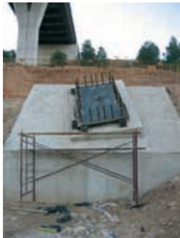
Figura 45. Replanteo placa apoyo Figure 45. Support plate stake-out
