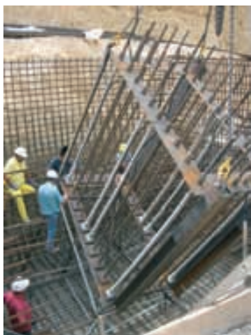
Figura 44. Replanteo de barras Figure 44. Bar stake-out
