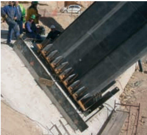
Figura 49. Empotramiento con contratueras Figure 49. Fixing with grip nuts
