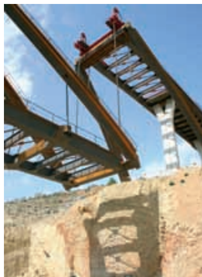
Figura 20. Izado a media carrera Figure 20. Hoisting operation
