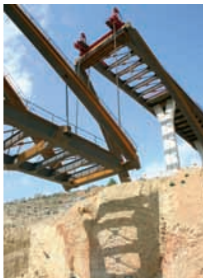
Figura 20. Izado a media carrera Figure 20. Hoisting operation
