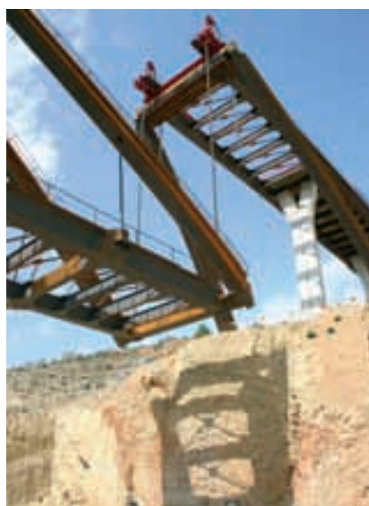
Figura 20. Izado a media carrera Figure 20. Hoisting operation
