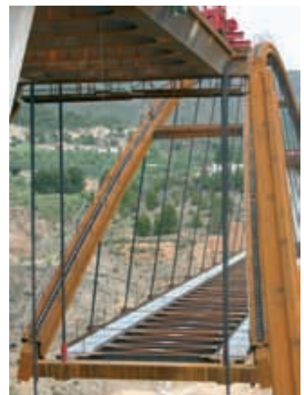
Figure 21. Riostra de bowstring Figure 21. Bowstring brace
