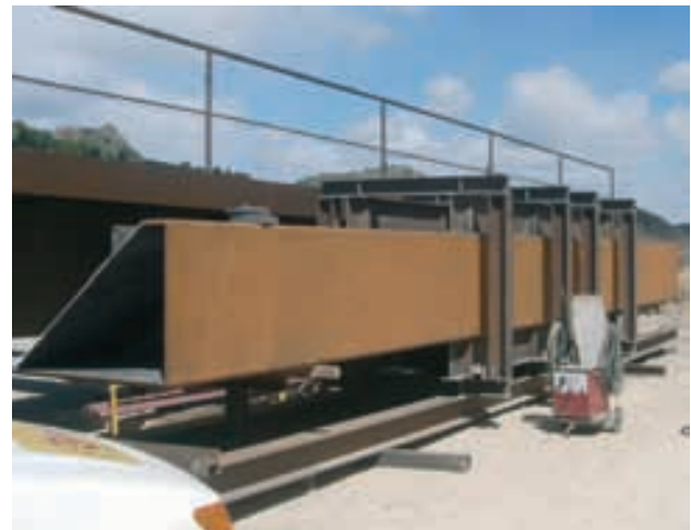
Figura 50. Riostra de voladizo Figure 50. Cantilever brace
