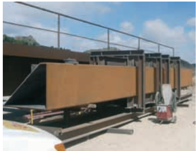
Figura 50. Riostra de voladizo Figure 50. Cantilever brace
