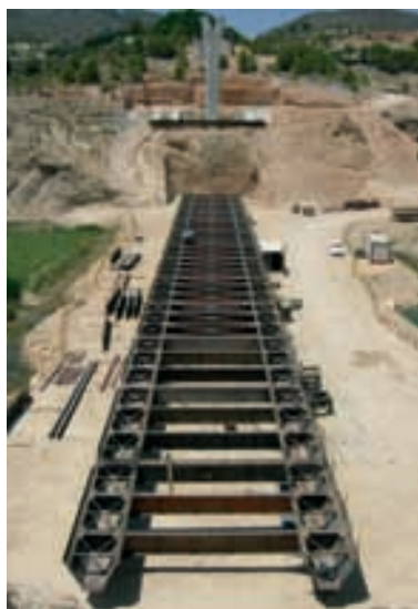
Figura 13. Bowstring (I). Tablero Figure 13. Bowstring (I). Deck
