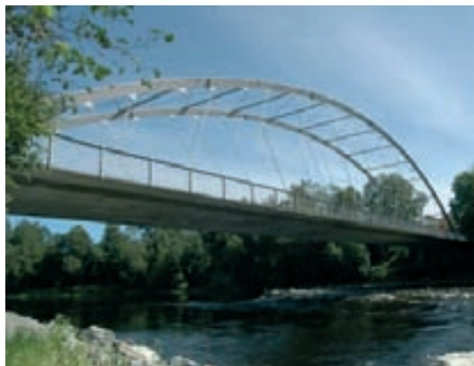
Figura 1. Puente de Steinkjer(1963) Figure 1. Steinkjer Bridge (1963)
