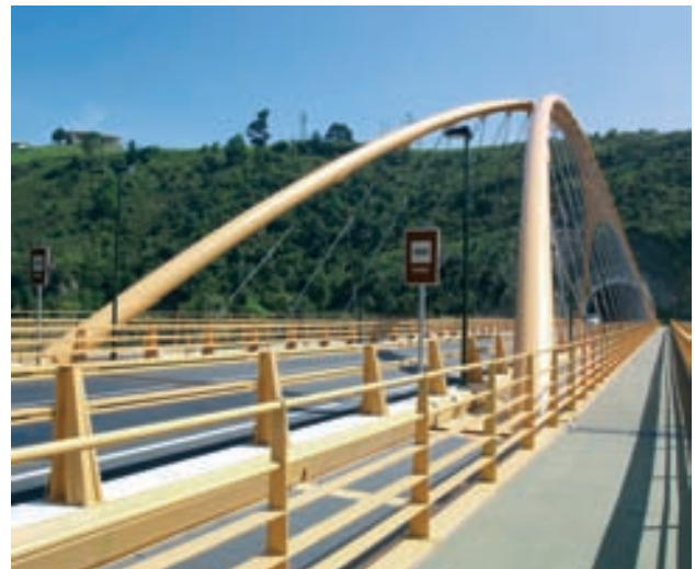
Figura 10. Vista de las aceras voladas laterales Figure 10. View of the lateral sidewalks on cantilever ribs
