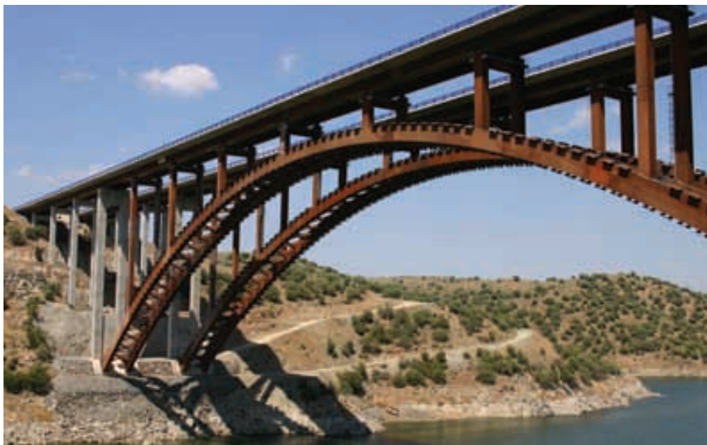
Figura 63. Vista general de la obra terminada Figure 63. General view of the finished work.
