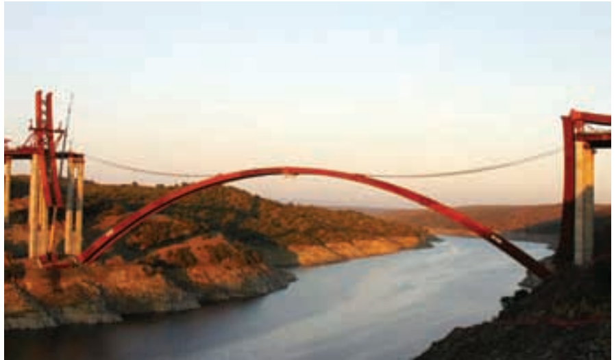
Figura 35. Cierre en clave. Figure 35. Crown closure.
