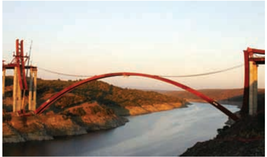
Figura 35. Cierre en clave. Figure 35. Crown closure.
