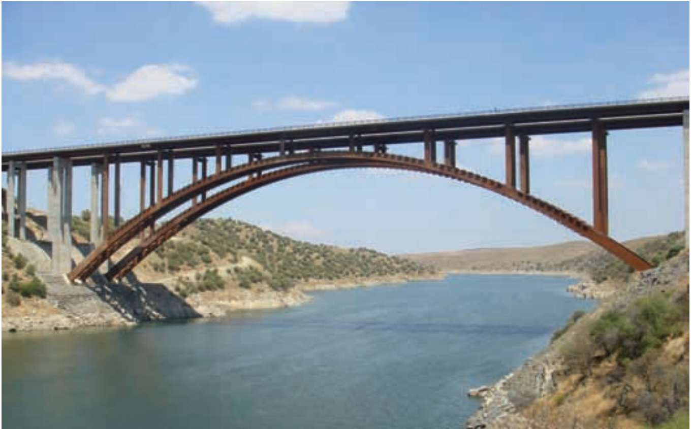
Figura 1. Vista general. Figure 1. General view.
