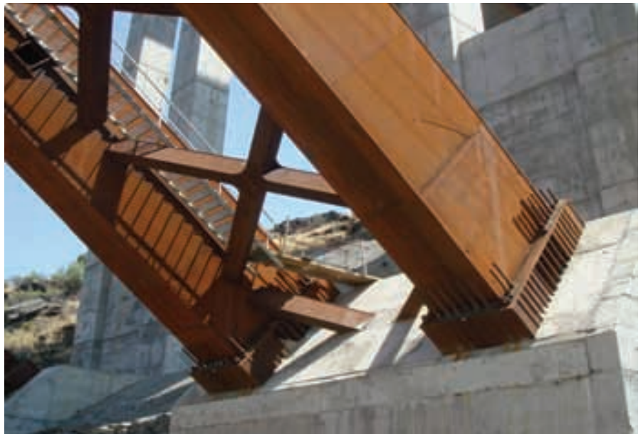
Figura 36. Empotramiento del arco en su base. Figure 36. Fixing the arch in its base.
