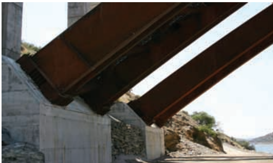
Figura 10. Empotramiento del arco. Figure 10. Arch fixing.
