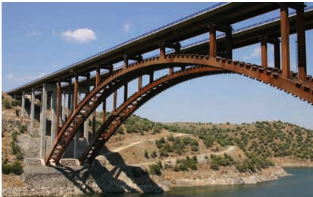
Figura 63. Vista general de la obra terminada Figure 63. General view of the finished work.
