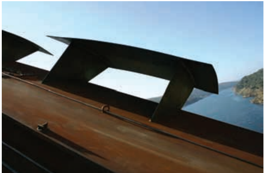
Figura 58. Deflector. Detalle. Figure 58. Guide vane. Detail.
