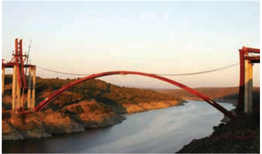
Figura 35. Cierre en clave. Figure 35. Crown closure.
