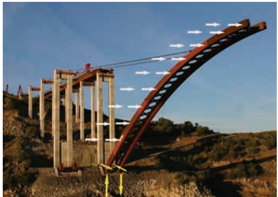
Figura 50. Efecto del viento lateral sobre un semiarco durante la maniobra de abatimiento. Figure 50. Side wind effect on one semi-arch during the swivel lowering operation.
