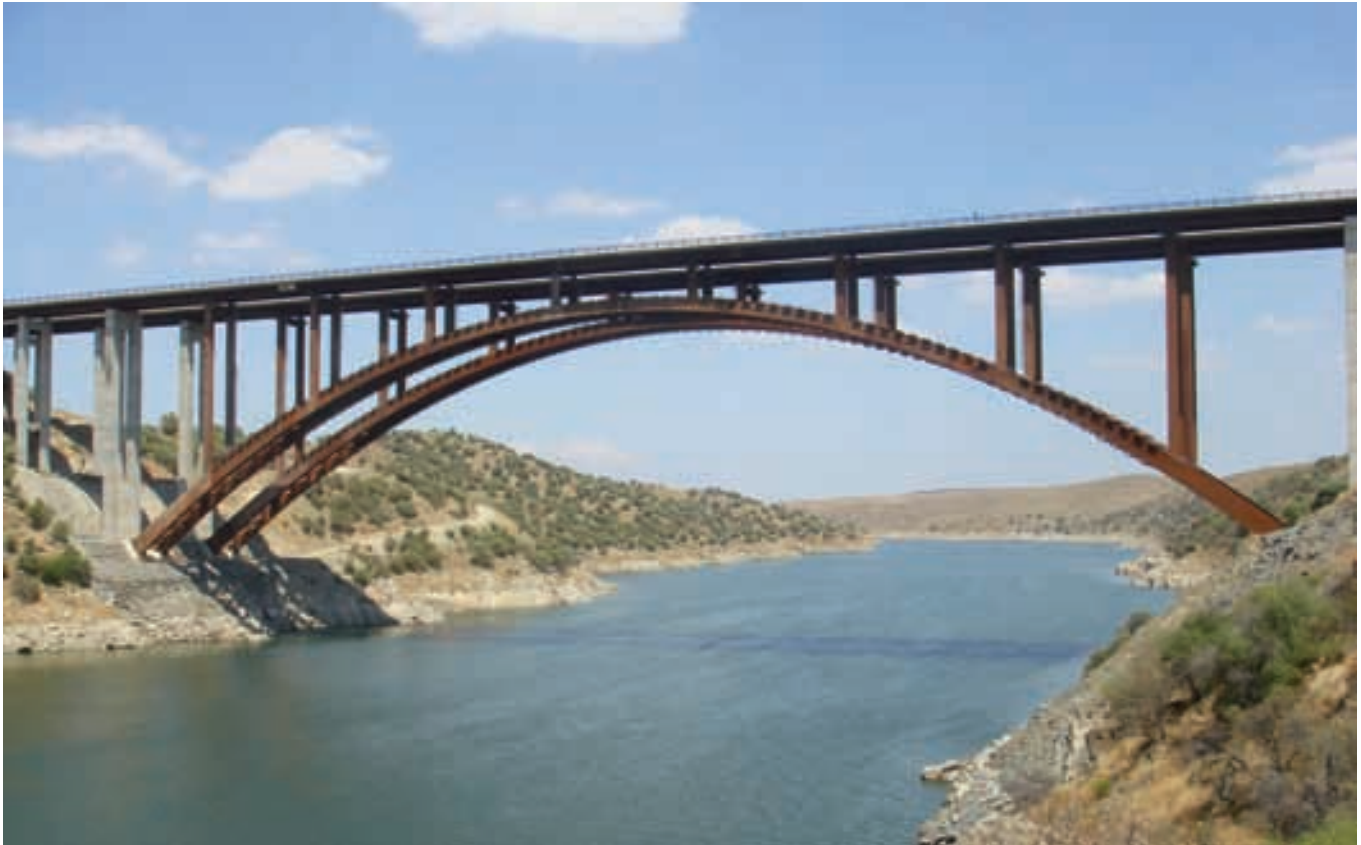
Figura 1. Vista general. Figure 1. General view.
