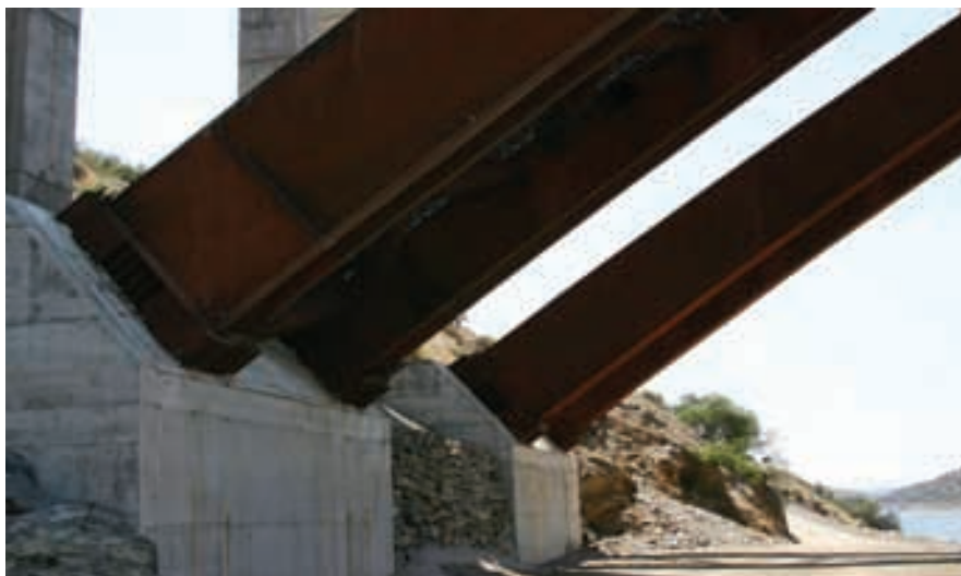
Figura 10. Empotramiento del arco. Figure 10. Arch fixing.
