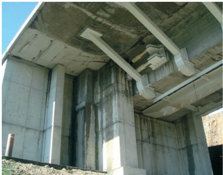
Figura 11. Vista general del estribo y dispositivos transmisores de carga Figure 11. General view of the abutments and of the shock transmission devices
