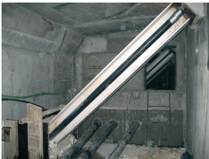
Figura 21. Puntales, diagonales y desviador en centro de vano Figure 21. Inclined internal supports and transverse wall in the centre of the span
