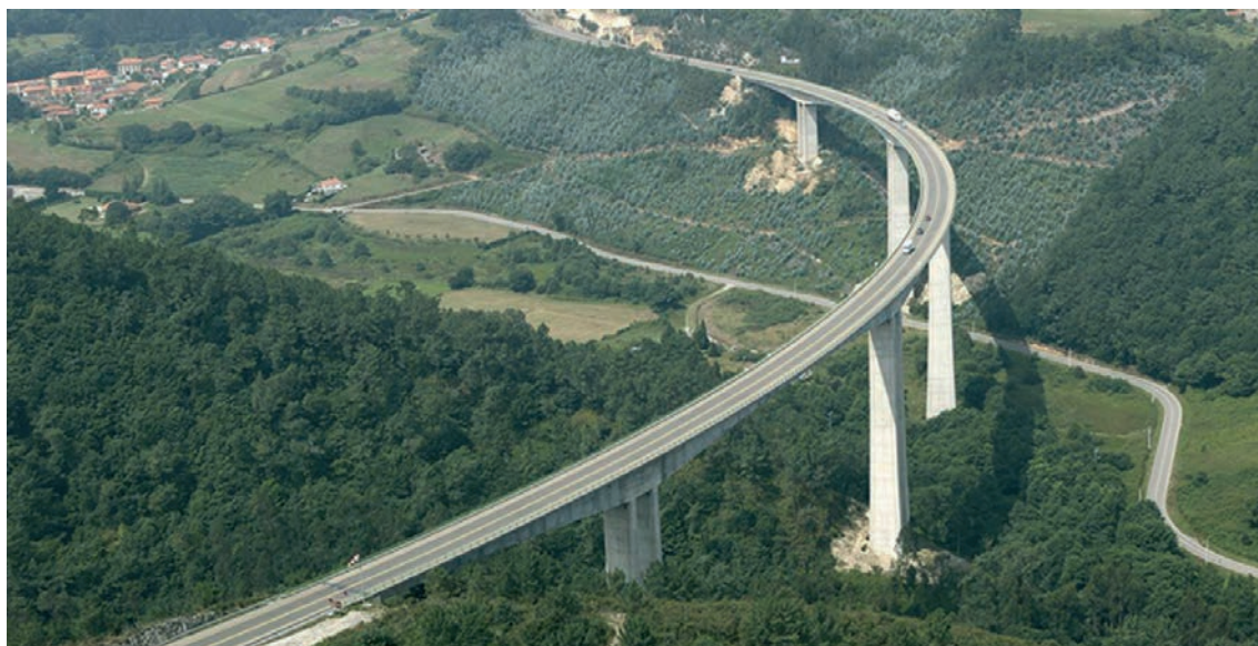
Figura 2. Viaducto original Figure 2. Existing bridge
