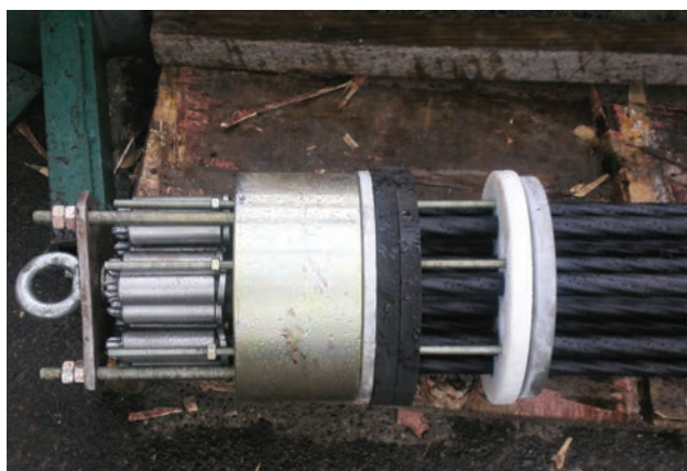
Figura 27. Nuevo anclaje superior con manguitos Figure 27. New top unions equipped with extrusion sleeves
