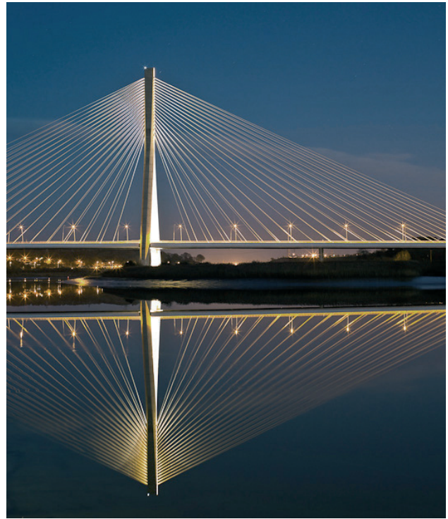
Figura 34. Foto nocturna del puente Figure 34. Night view of the bridge
