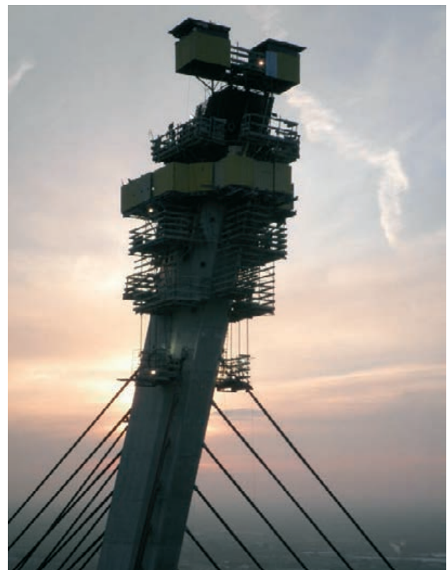
Figura 20. Encofrado autotrepante Figure 20. Self-climbing formwork
