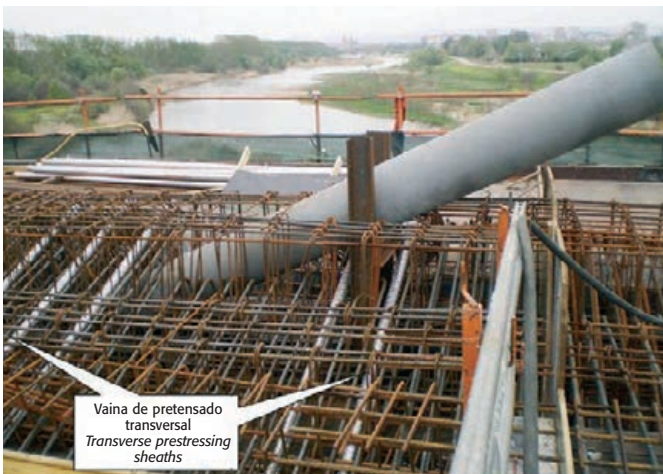
Figura 9. Vainas de pretensado transversal en la salida del tirante Figure 9. Transverse prestressing sheaths around the base of the stay
