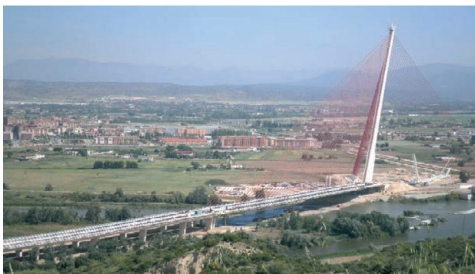
Figura 43. Vista del puente terminado con Talavera al fondo Figure 43. View of the finished bridge with Talavera in the background
