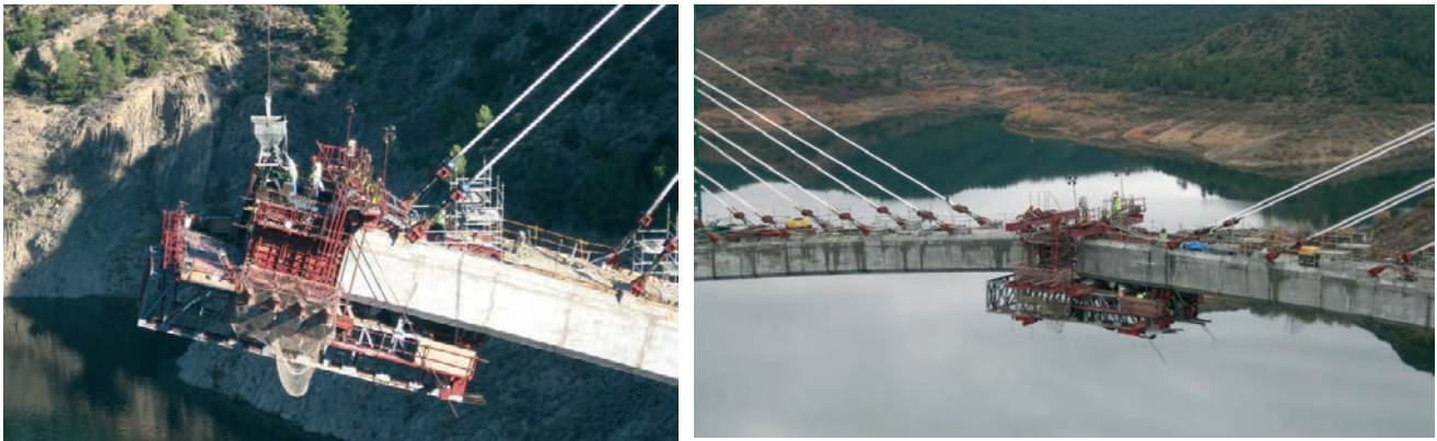
Figura 20. Detalles del carro de avance y del cierre en clave Figure 20. Details of the form traveller and the connection at the key
