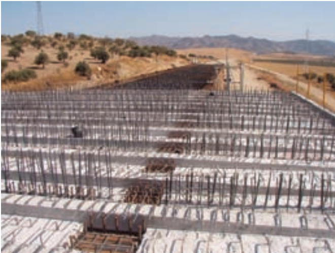
Fig. 12. Vista de prelasas superiores. Fig. 12. View of the top pre-slabs.
