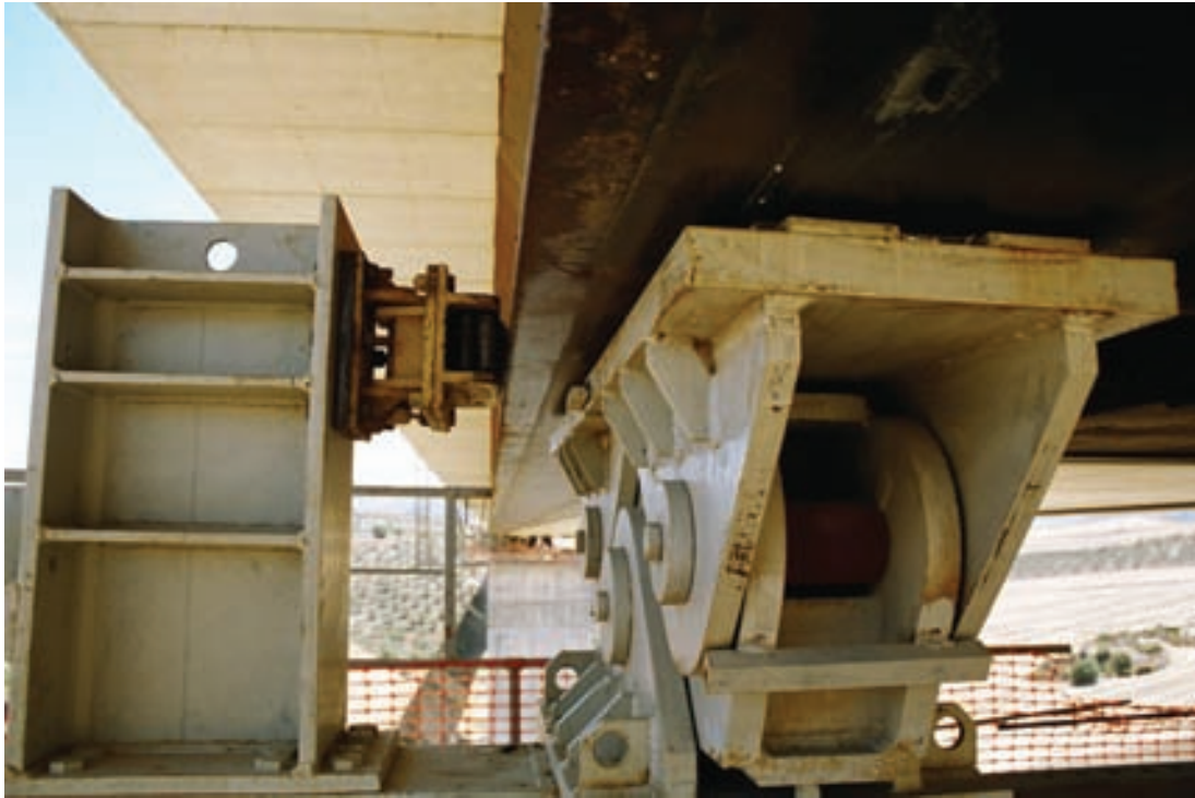
Fig. 18. Detalle de apoyos deslizantes con topes laterales durante el empuje. Fig. 18. Detail of sliding bearings with side stops during launching.
