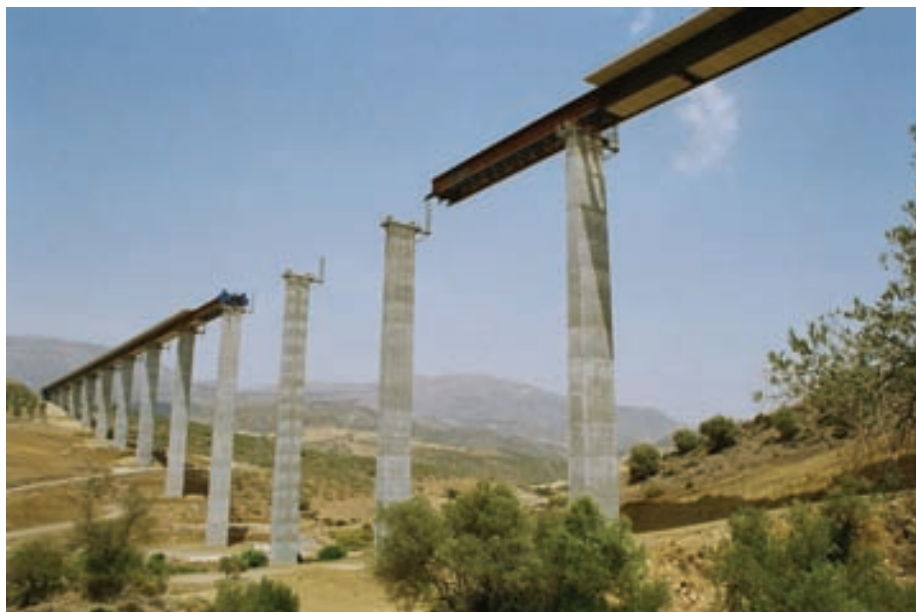
Fig. 31. Vista de pilas durante el empuje. Fig. 31. View of piers during launching.
