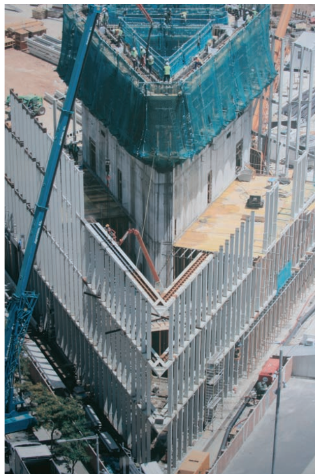
Figura 7. Avance de fachada y núcleo Figure 7. Concrete core and steel facade under construction
