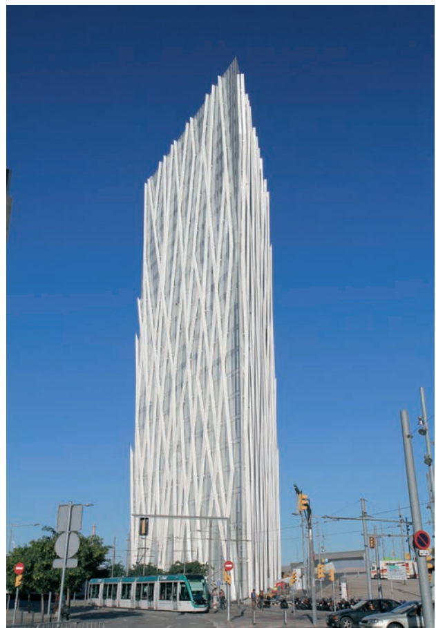
Figura 3. Vista de la torre Diagonal ZeroZero desde la Avenida Diagonal Figure 3. Diagonal ZeroZero tower elevation from the Avenida Diagonal
