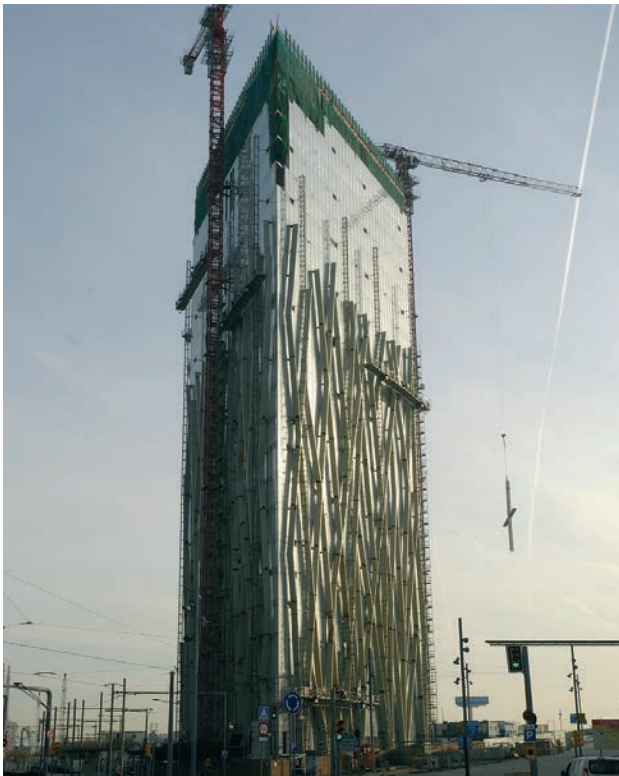
Figura 31. Elevación nudo mediante grúa torre Figure 31. Elevation of a bamboo intersection node by means of the tower crane
