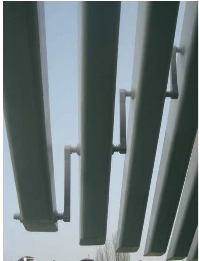
Figura 58. Arriostramientos finalizados Figure 58. Bracing system already finished
