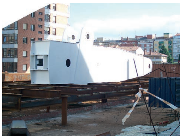
Figura 30. Palanca guiadora antes de ser instalada en el foso Figure 30. Lever arm before its installation in the housing of the cylinders
