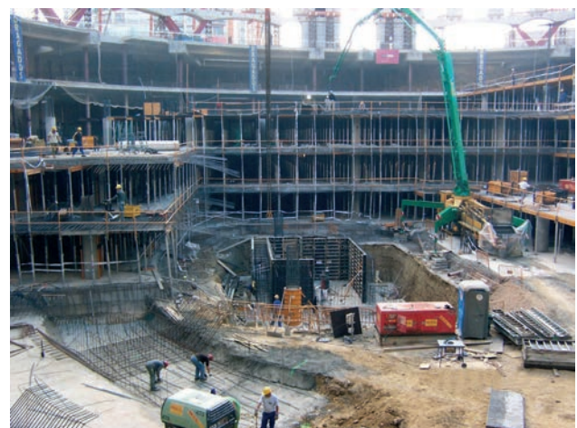
Figuras 36 y 37. Vista general y detallada de la construcción ascendente sectorizada Figures 36 & 37. General and detailed view of upward construction divided into sectors
