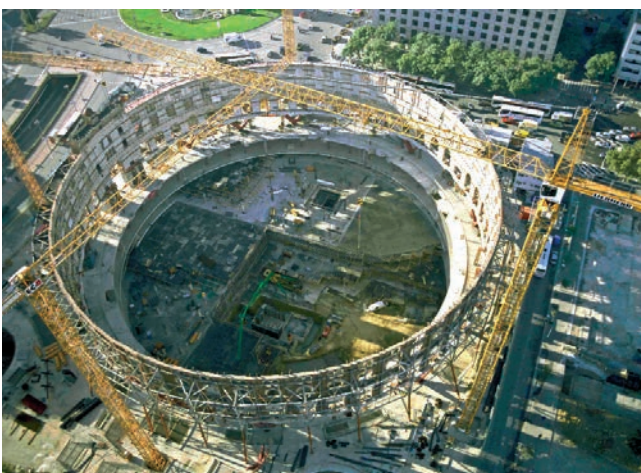
Figuras 36 y 37. Vista general y detallada de la construcción ascendente sectorizada Figures 36 & 37. General and detailed view of upward construction divided into sectors
