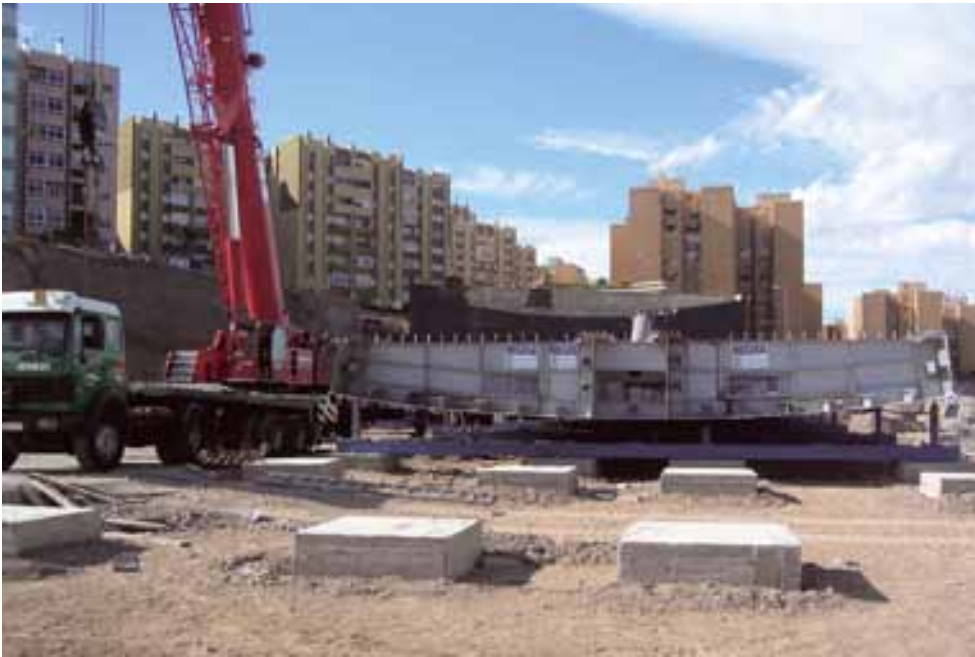
Figura 13. Marco transversal. Figure 13. Transverse frame.
