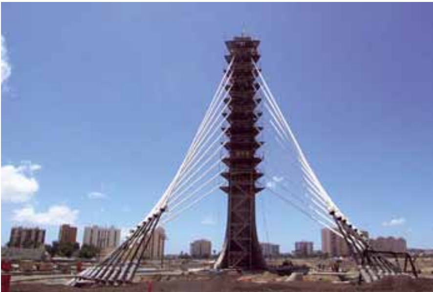
Figura 37. Vista trasera de los tirantes durante el montaje. Figure 37. Rear view of the stays during assembly.
