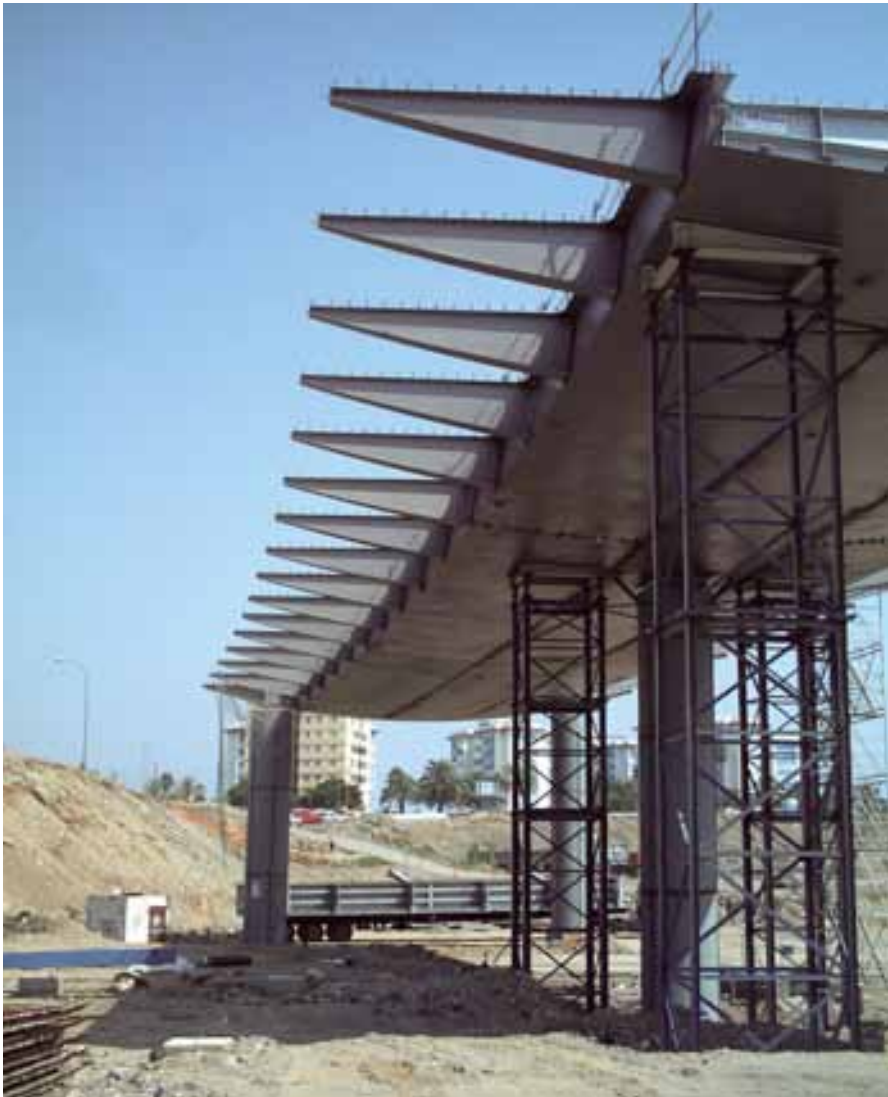
Figura 14. Costillas metálicas Figure 14. Metal ribs.
