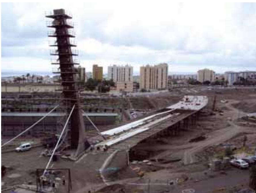
Figura 35. Montaje de la primera terna de tirantes. Figure 35. Assembly of the first batch of stays.
