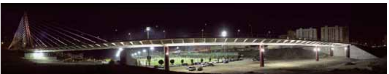
Figura 6. Vista del viaducto iluminado desde el parque Figure 6. View of the illuminated viaduct from the park.
