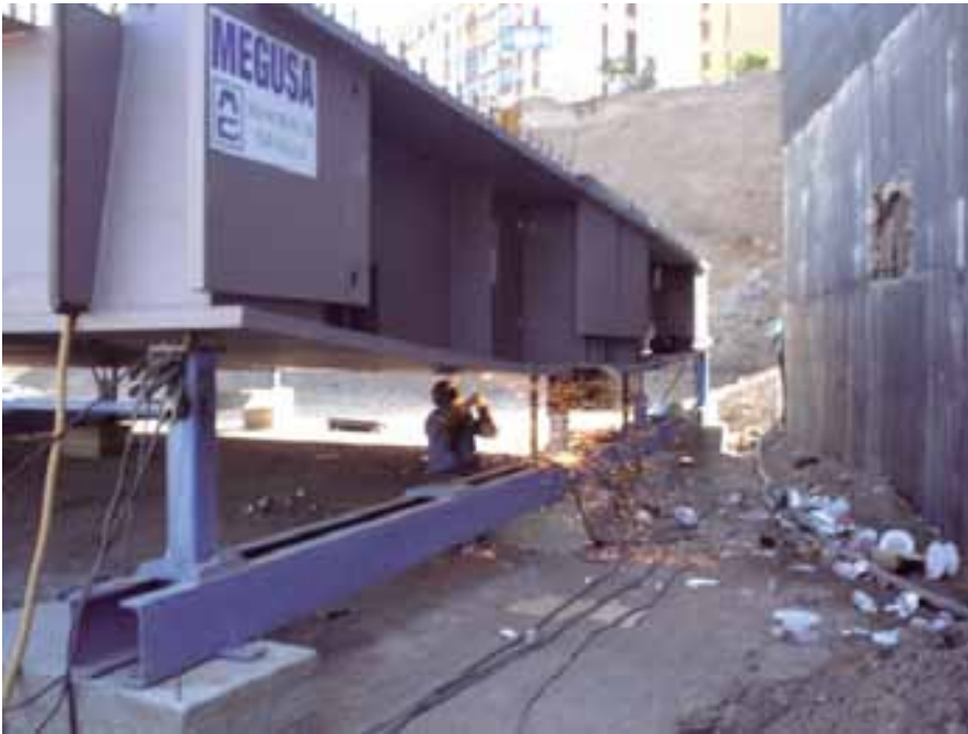
Figura 16. Diafragma de estribo 1. Figure 16. Diaphragm of abutment 1.
