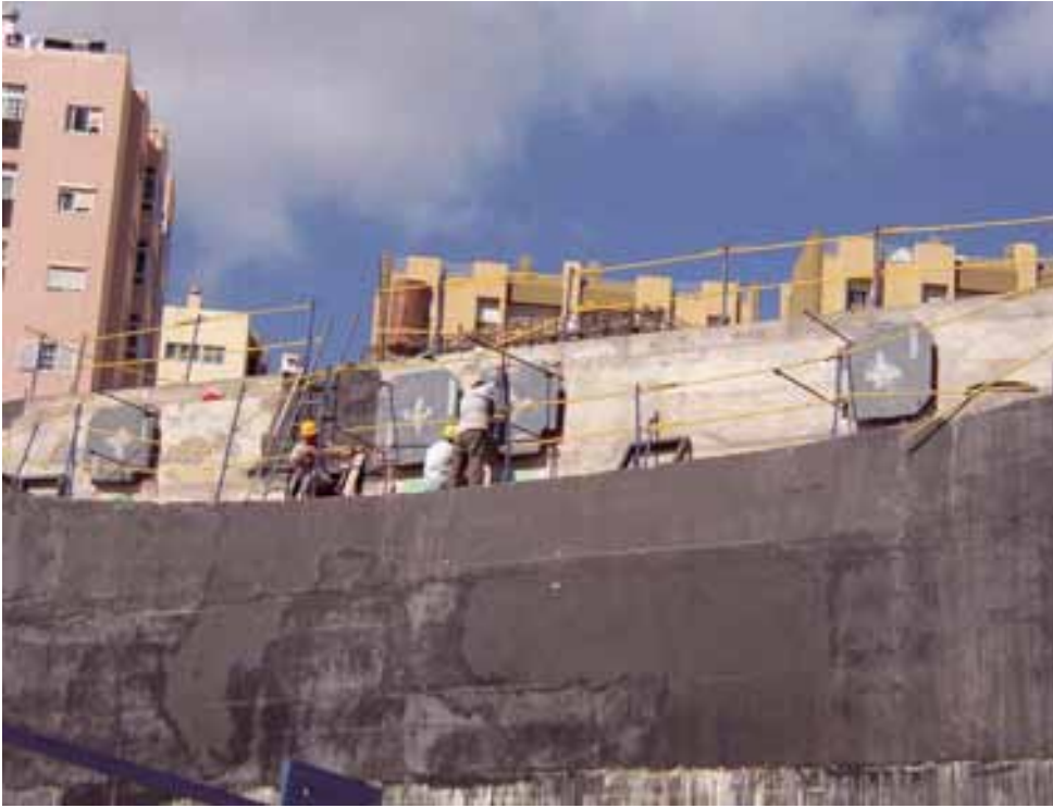
Figura 30. Frontal del cuerpo principal del estribo 1. Figure 30. Front wall of the main body of abutment
