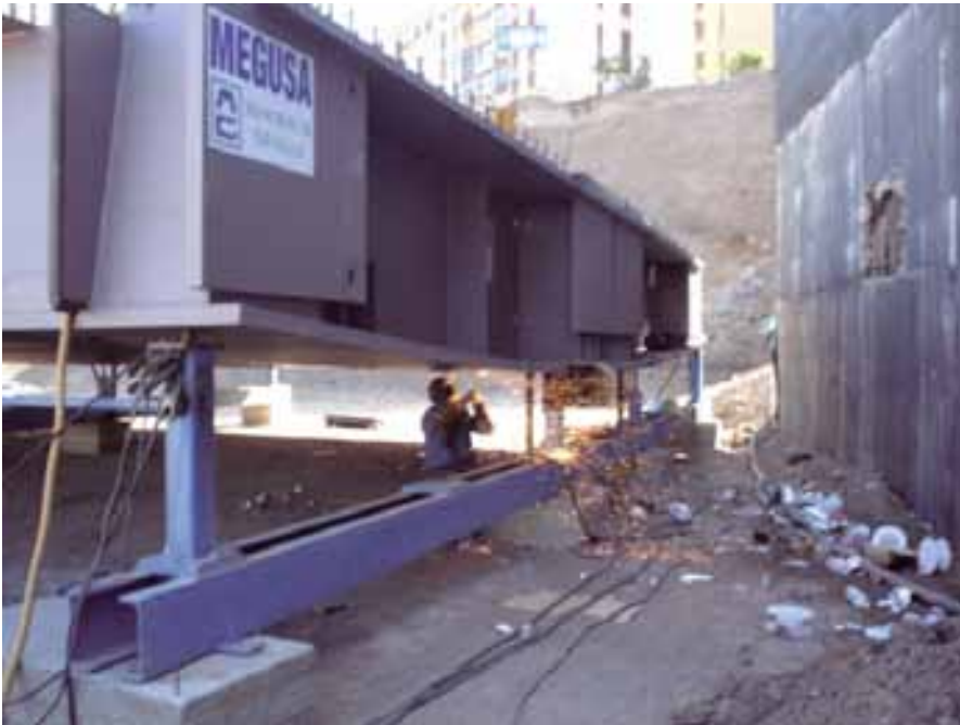
Figura 16. Diafragma de estribo 1. Figure 16. Diaphragm of abutment 1.
