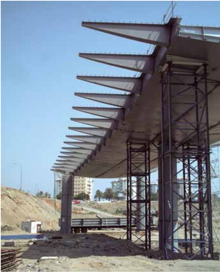
Figura 14. Costillas metálicas Figure 14. Metal ribs.
