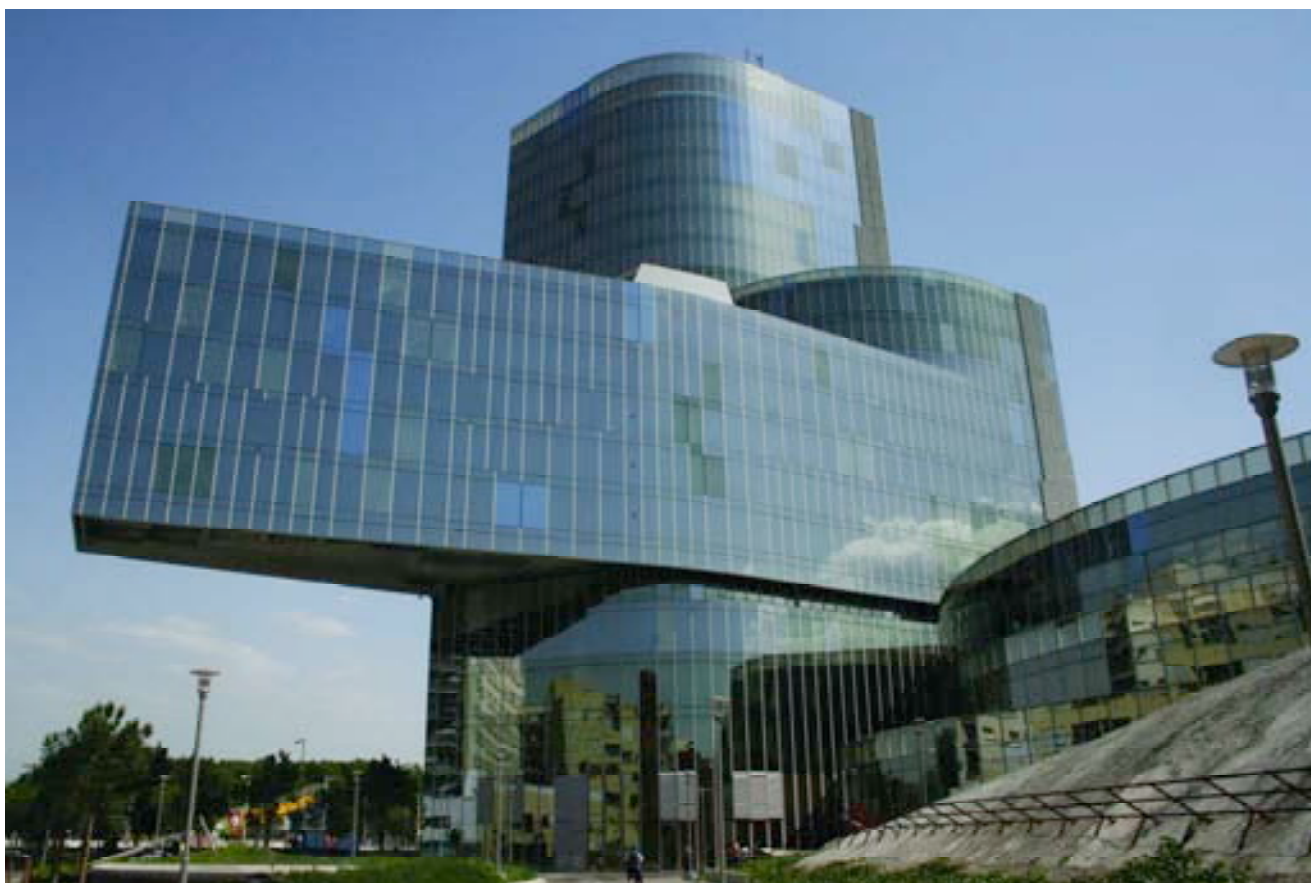
Figura 39. Vista general desde la fachada dorsal. Figure 39. General view from the rear façade.
