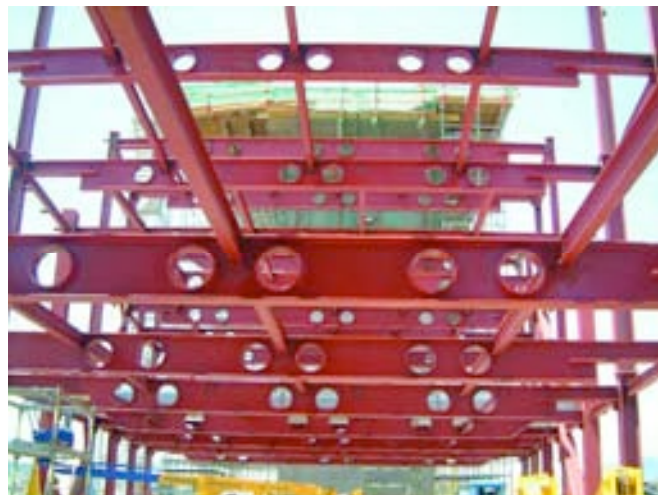
Figura 28. Estructura de vigas de una planta del Portaaviones. Figure 28. Beam structure on one floor of the Aircraft-carrier building.
