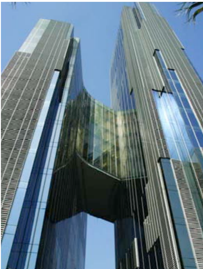
Figura 37. Vista dorsal del frente y la calle interior Figure 37. Rear view of the front and inner avenue.
