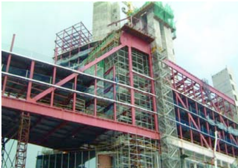
Figura 22. Vista de la ejecución de la fase 4 del Portaaviones. Figure 22. View of stage 4 construction of the Aircraft-carrier building.
