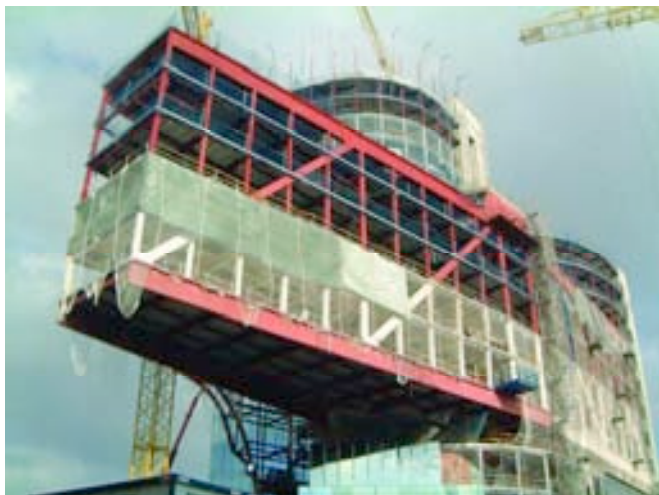
Figura 27. Vista final de la ejecución del Portaaviones. Figure 27. Final view of the construction of the Aircraft-carrier building.
