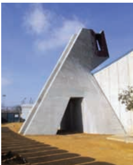
Figura 16. Vista del soporte desde el exterior. Figure 16. View of the support from the outside.
