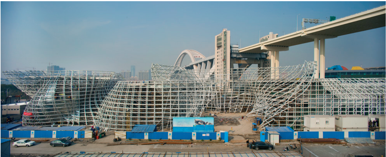
Figura 2. Vista general del pabellón en construcción, con la estructura de fachada completada Figure 2. General view of the pavilion under construction, with the facade structure completed
