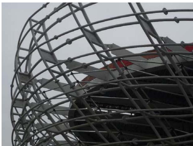
Figura 20. Detalle de la cubierta de la Sala Expositiva 2. Las vigas triangulares se unen por medio de bulones a la fachada, rigidizada por paneles en esa zona Figure 20. Detail of the roof of Exhibition Room 2, where the triangular beams are connected through pin-bolts to the facade, reinforced in this area with plates
