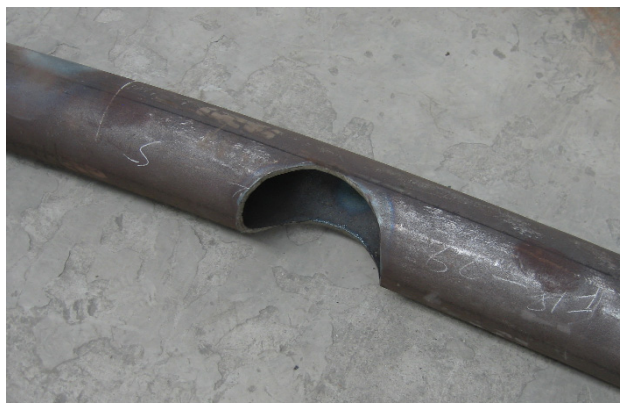
Figura 34. Corte completado con soplete sobre el tubo curvo Figure 34. Intersection cut finished by hand after curving
