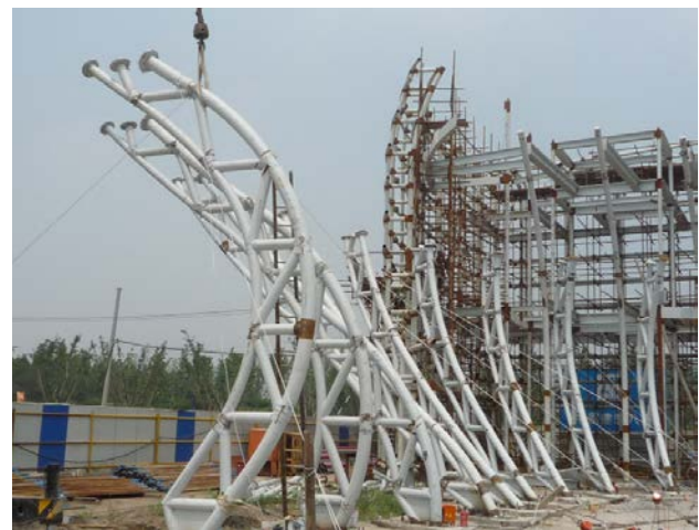
Figura 36. Montaje de la Sala Expositiva 2 Figure 36. Exhibition Room 2 under construction
