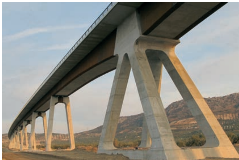
Figura 7. Pila central Figure 7. Central pier
