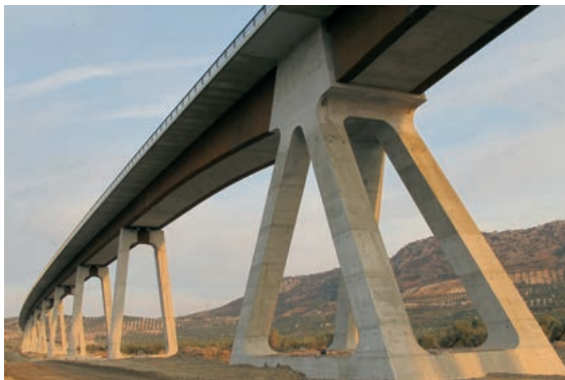
Figura 7. Pila central Figure 7. Central pier
