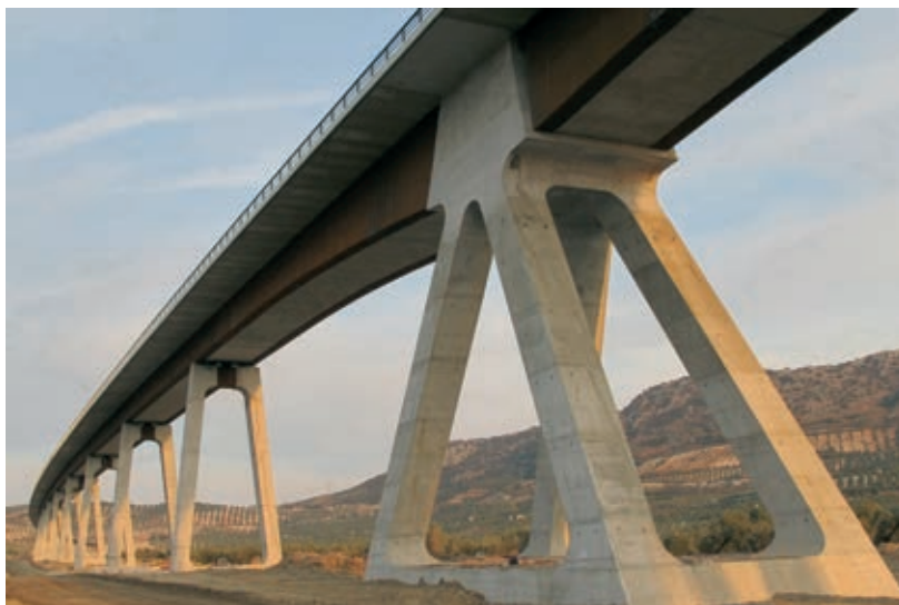
Figura 7. Pila central Figure 7. Central pier
