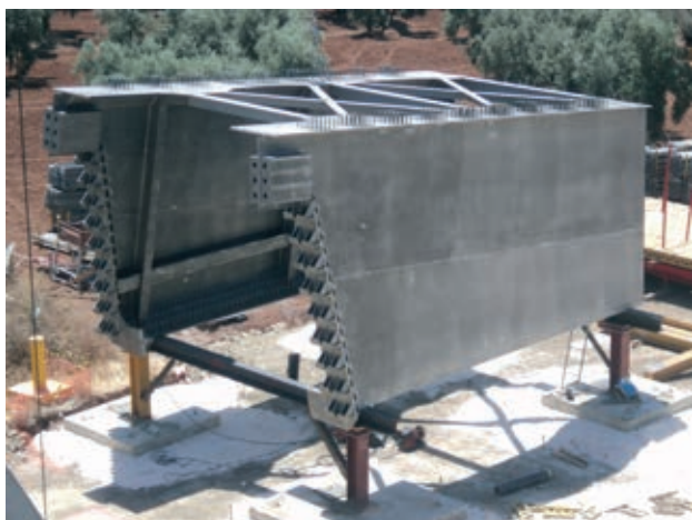
Figura 19. Conexión Pila-Tablero Figure 19. Pier-deck connection
