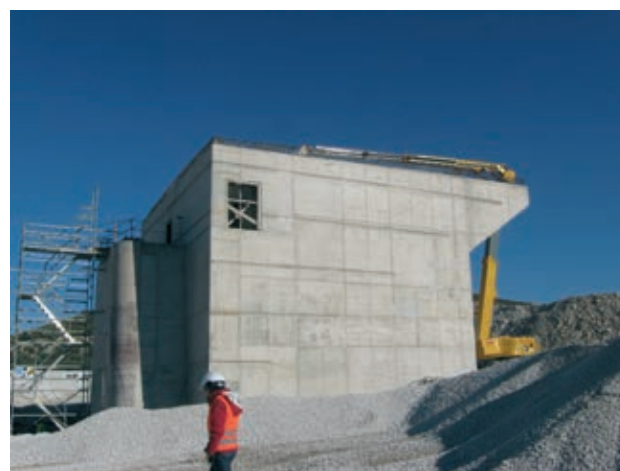
Figura 8. Estribo Figure 8. Abutment
