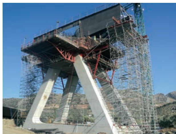
Figura 19. Conexión Pila-Tablero Figure 19. Pier-deck connection
