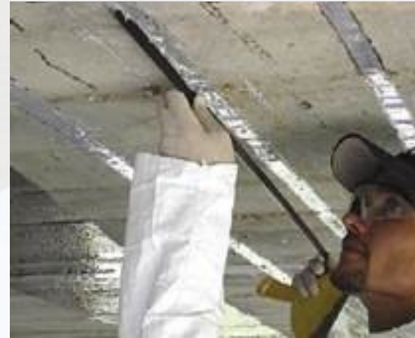
Near surface mounted (NSM) reinforcement
