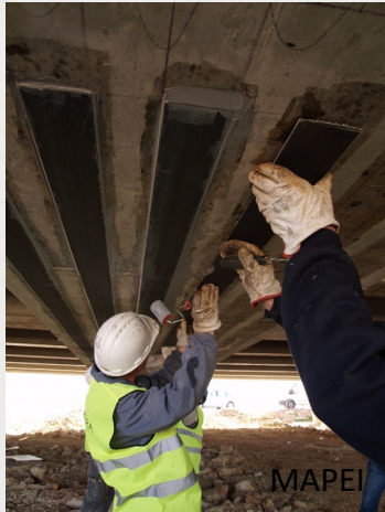
Externally bonded reinforcement (EBR)
