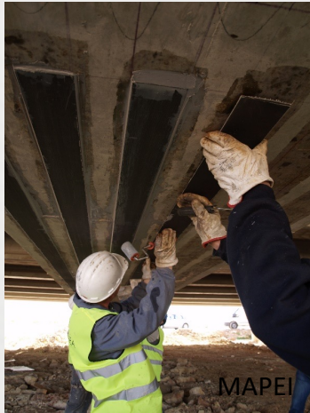
Externally bonded reinforcement (EBR)
