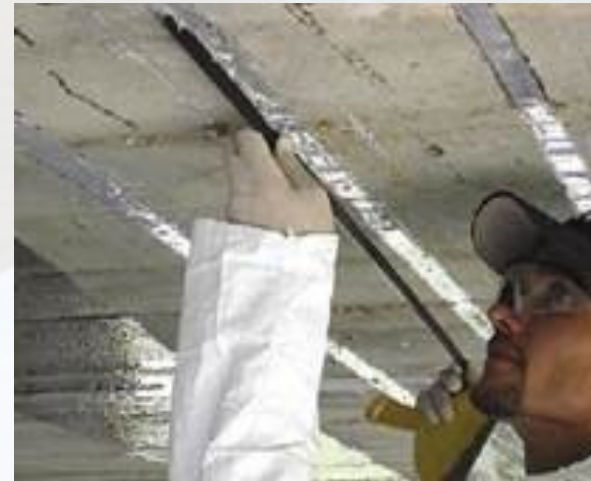
Near surface mounted (NSM) reinforcement
