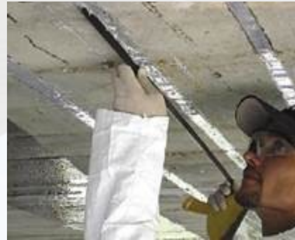
Near surface mounted (NSM) reinforcement
